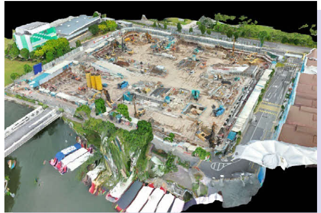
Drone flight showing aerial view of the site, conducted bi-weekly for site progress.
