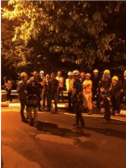
Briefing to Crane Operator, CCS and SCDF's team
