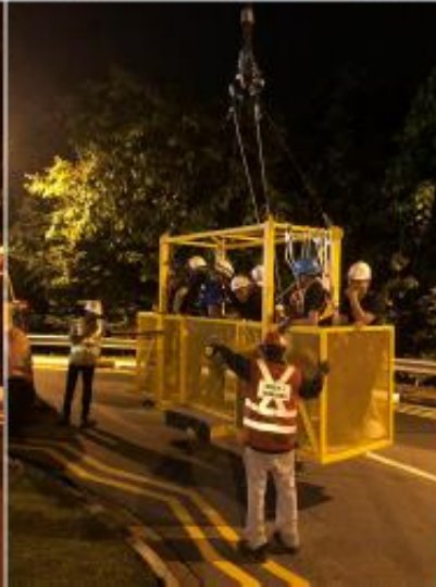
Rigger man ensuring all lifting components is secured
