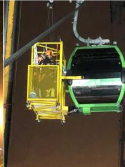
Rescue-Cage being anchored to the cabin
