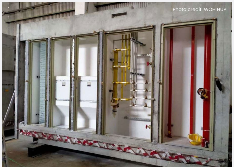
Ⓜ Fitting out of the integrated Prefab MEP riser
