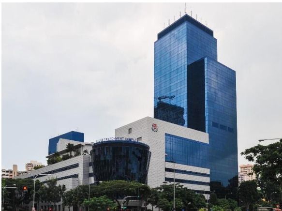
Police Cantonment Complex
