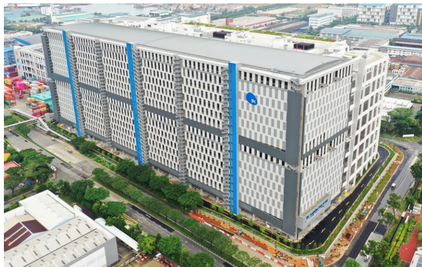
Photo Credit to Kimly Construction Pte Ltd
