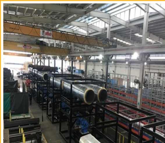
Prefabricated Mechanical and Electrical Plumbing (MEP)
