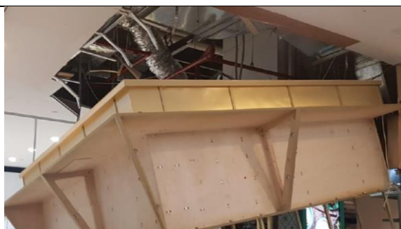
Figure 2-7: Collapsed Suspended Ceiling Due to Additional Load from Cabinet
