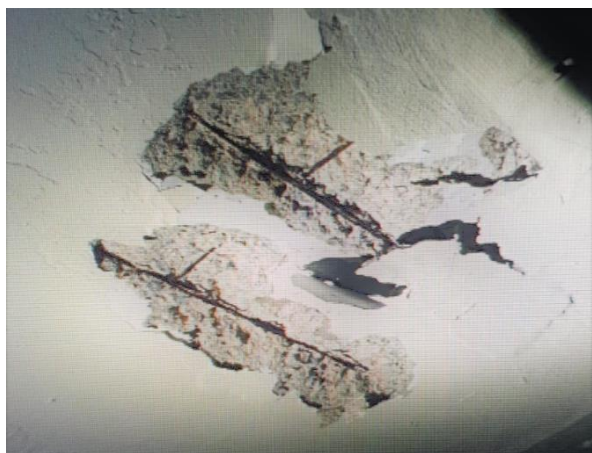
Figure 7-3: Spalling Concrete at Ceiling Soffit
