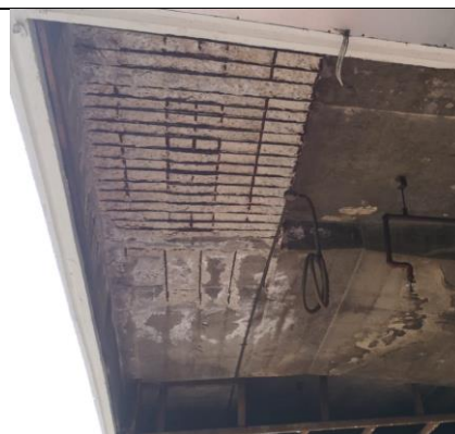
Figure 2-6: Collapsed Suspended Ceiling Due to Spalling Concrete at Ceiling Soffit
