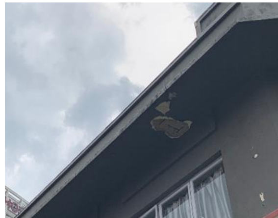
Figure 7-2: Spalling Concrete at Roof Eave
