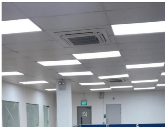
Figure 2-1: Gypsum Suspended Ceiling in Office Spaces
