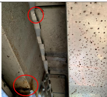
Figure 2-5: Collapsed Suspended Ceiling Due to Water Ingress and Rusty Screws
