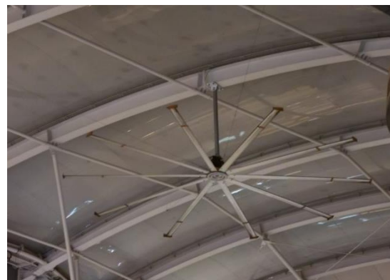
Figure 5-2: HVLS Fan attached to steel structure
