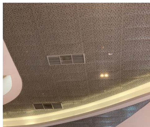
Figure 2-2: Metallic Suspended Ceiling in Shopping Mall
