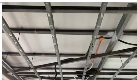
Figure 2-8: Collapsed Suspended Ceiling Due to Progressive Failure of Panel Support
