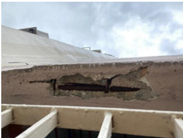
Figure 7-1: Spalling Concrete at Facade Edge
