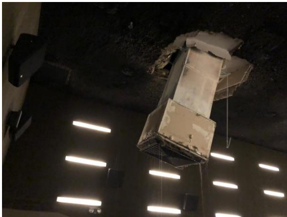
Figure 3-5: Collapsed ACMV Duct Due to Excessive Condensation
