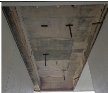
Figure 2-9: Collapsed Suspended Ceiling at Building Periphery Due to Failure of Timber Supporting Frame with Nails
