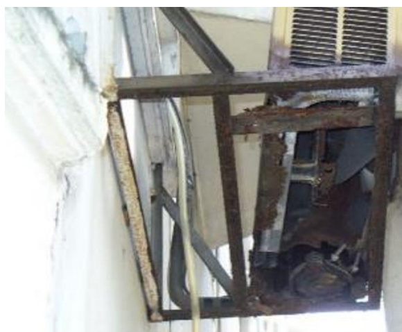
Figure 4-6: Corroded Aircon Compressor Fixture
