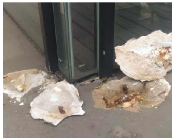
Figure 7-4: Spalling Concrete at Ledge
