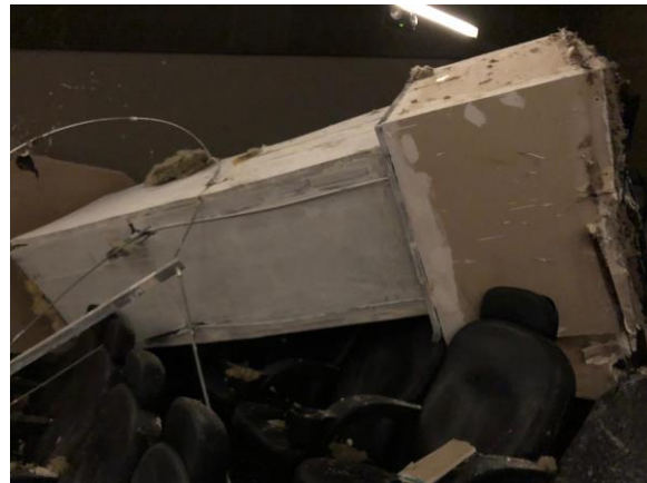
Figure 3-6: Collapsed ACMV Duct Due to Excessive Condensation
