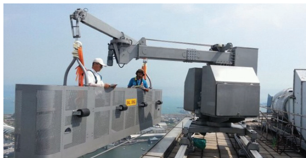
Access for Maintenance: A building maintenance unit (BMU) allows safe, easy access for maintenance crews; it obviates riskier and more labour-intensive methods, such as scaffolding.
