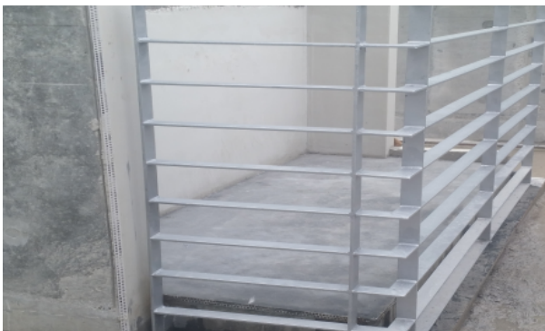
Figure: Railing Installation
