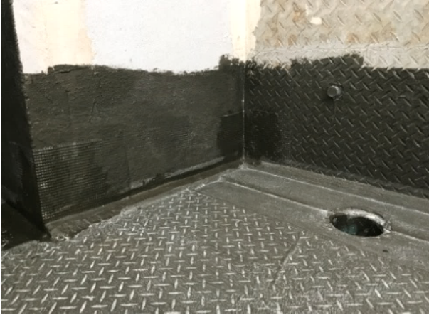
Figure: Waterproofing Application
