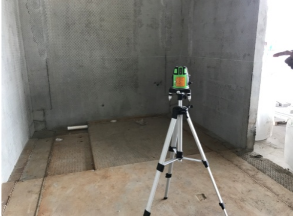
Figure: Alignment verification.
