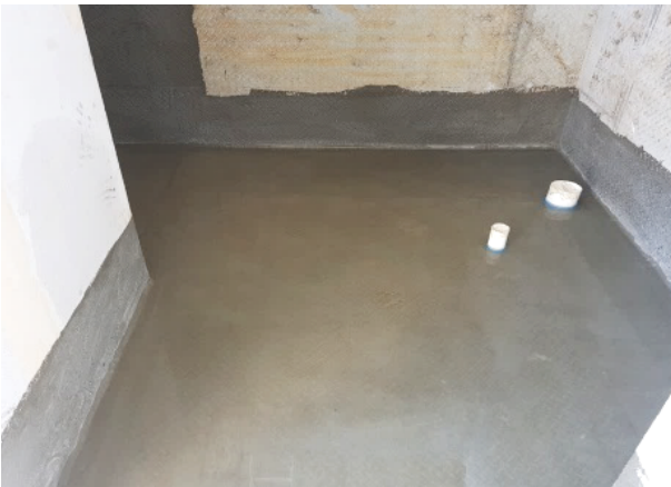
Figure: Water Ponding Test
