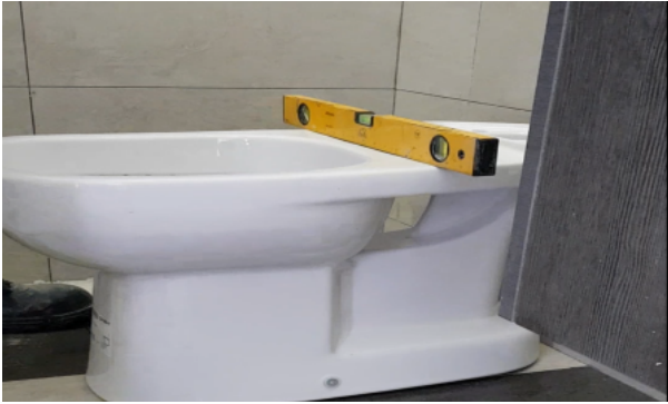
Figure: WC Installation
