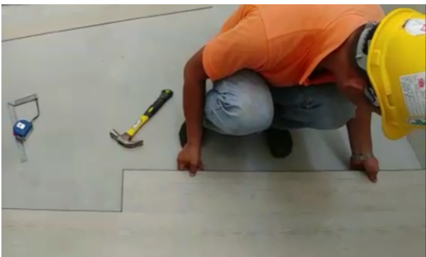
Figure: Floor finishes Installation
