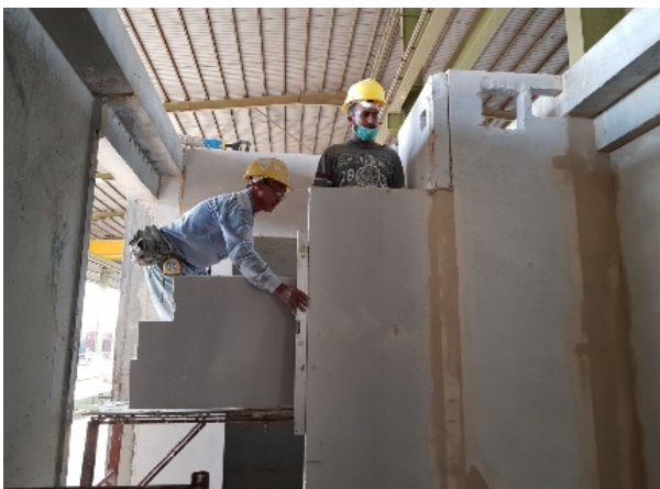
Figure: Lightweight Panel Installation
