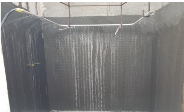
Figure: Spray Test
