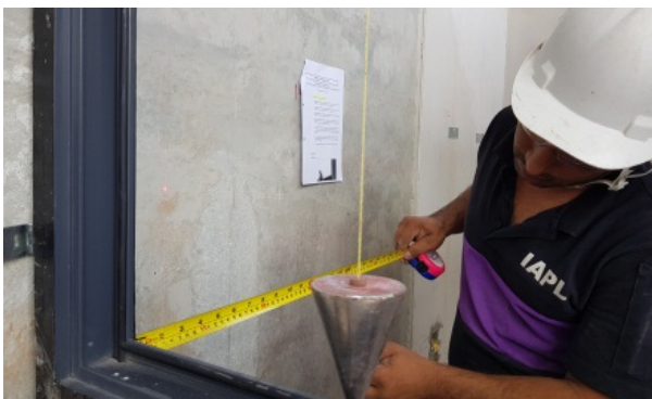
Figure: QC check on Window Installation
