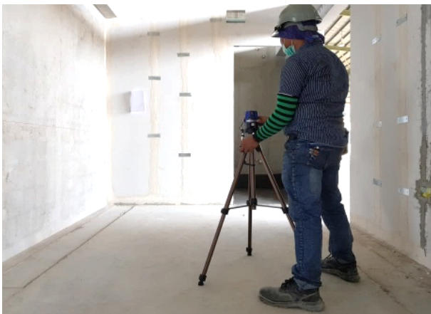
Figure: Levelling of module
