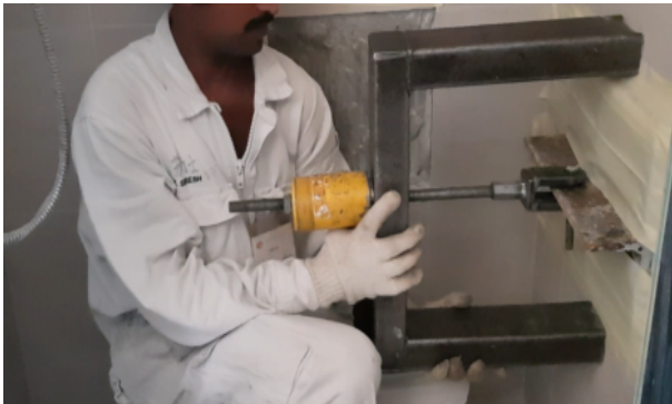
Figure: Alignment verification.
