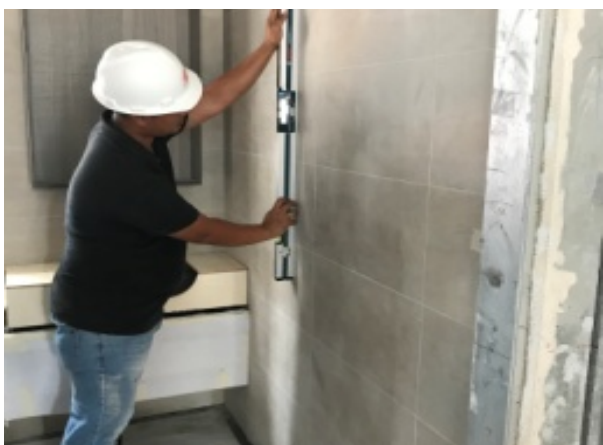
Figure: QC Check on Tiling
