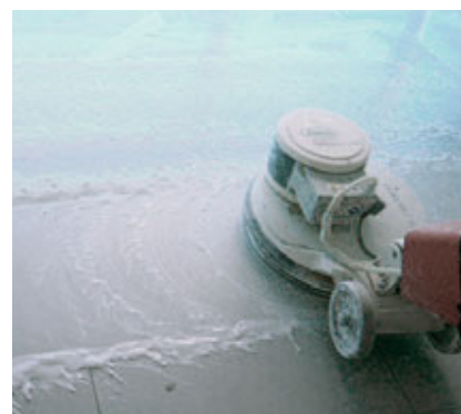
Fig. 6.3 – Wet polishing on a marble floor.
