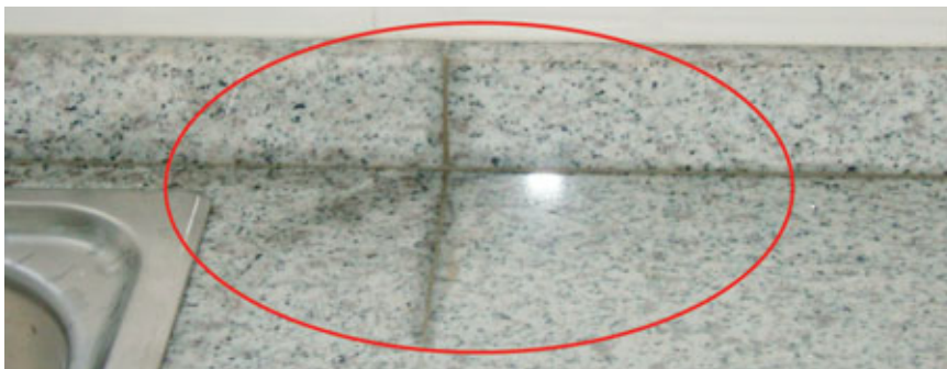
Fig. 2.4 – Porosity in natural stones attracts liquid and moisture ingress.
