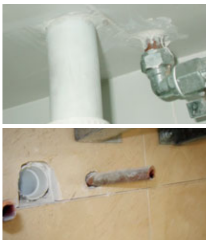
Fig. 13.13 – Examples of untidy pipe protrusions from tiled surfaces.
