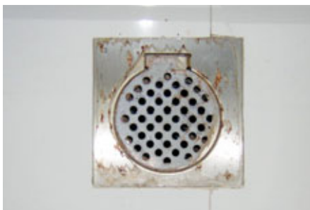
Fig. 13.5 – Tarnishing and blockage of grating are common after use.
