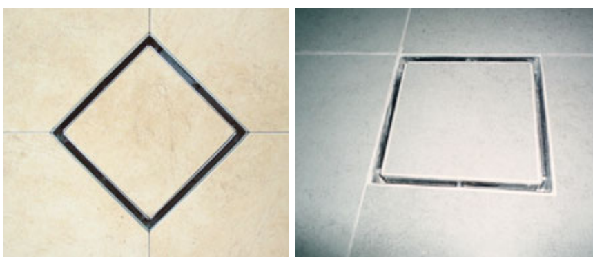
Fig. 13.8 – Discharge traps are hidden beneath the floor finishes.
