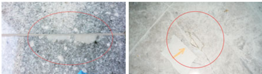
Fig. 9.3 – Fillers without stone chips may not achieve reflective effect of original condition.
