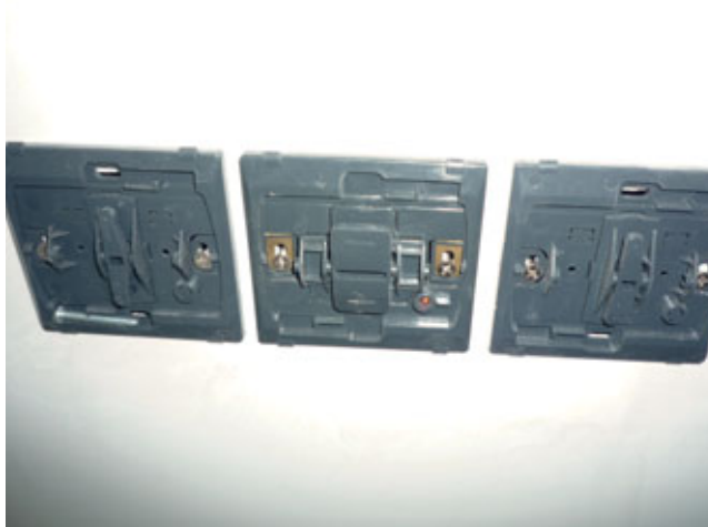
Fig. 13.20 – The final coat of wall paint can be carried out.
