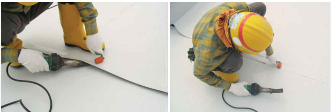
Fig. 12.3 – Using hot air torch to weld the joint of PVC membranes.
