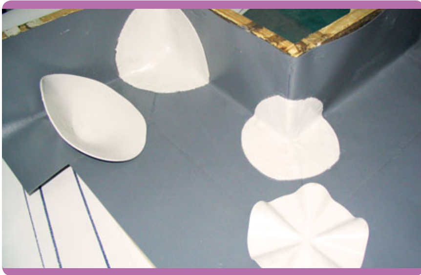
Fig. 12.11 – Prefabricated corner pieces for internal and external corners.
