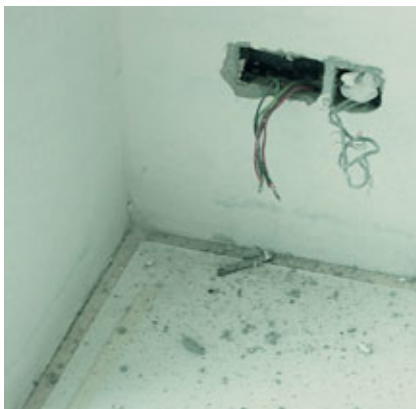
Fig. 13.17 – Adjusting position (after plastering and painting) leads to unpleasant consequences.
