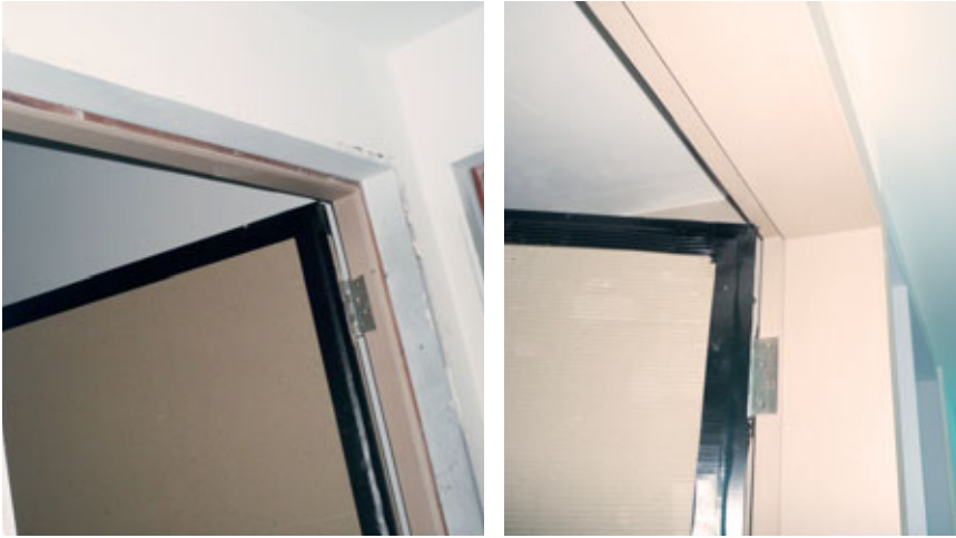
Fig. 10.13 – A typical installation process using integrated frame and architrave.
