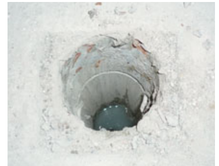
Fig. 13.4 – A typical 100 mm floor trap sleeve cast together with concrete slab.
