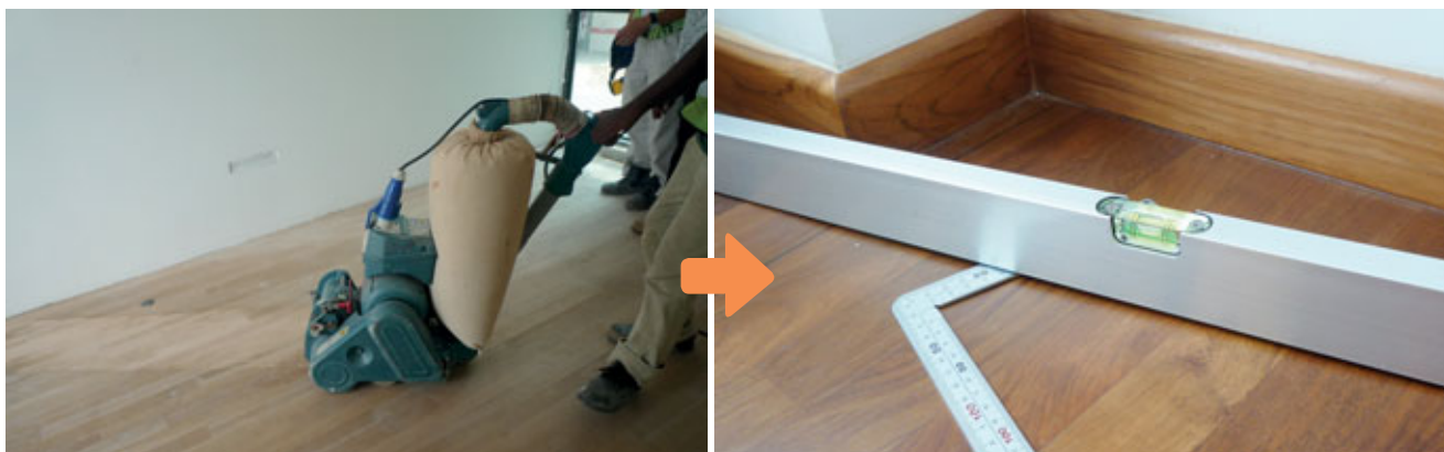
Fig. 8.8 – Poor control in the sanding process may also lead to unevenness in the finished surface.
