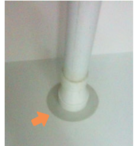
Fig. 13.16 – Rubber based universal end cap for sanitary discharge pipe.
