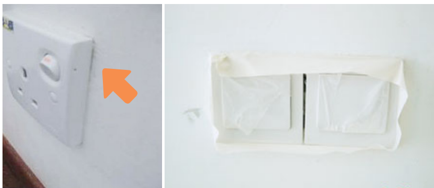
Fig. 13.18 – Inconsistent gap and paint stains are possible issues.
