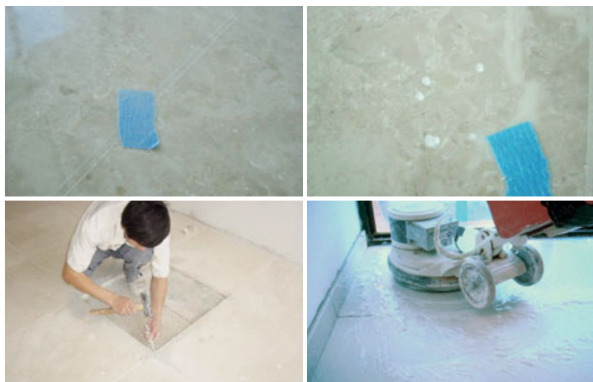
Fig. 9.1 – Stones are prone to minor chips and scratches during construction. Replacing it can have consequences like tone difference, wet polishing and others.
