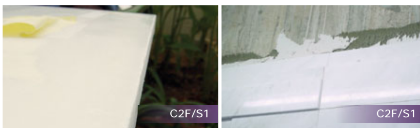
Fig. 5.2 – Porous natural stones with a substrate of cement render or concrete.
