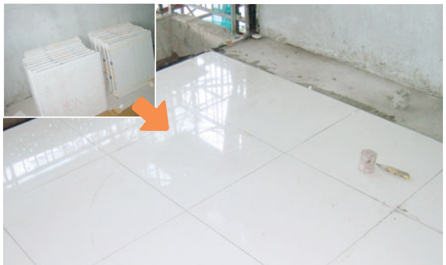
Fig. 1.9 – Direct installation (without dry lay) saves time and cost in construction.
