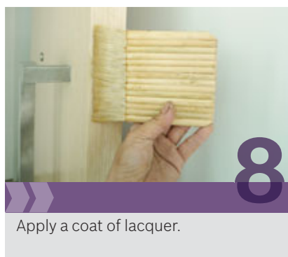
Fig. 9.9 – Sequences in veneer surface rectification using timber putty.
