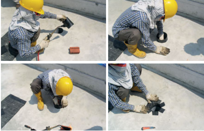
Fig. 12.8 – Wrapping around pipe penetration.
