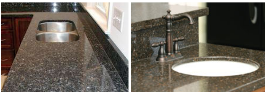
Fig. 2.5 – Non-porous surface does not require sealing in the counter-top.
