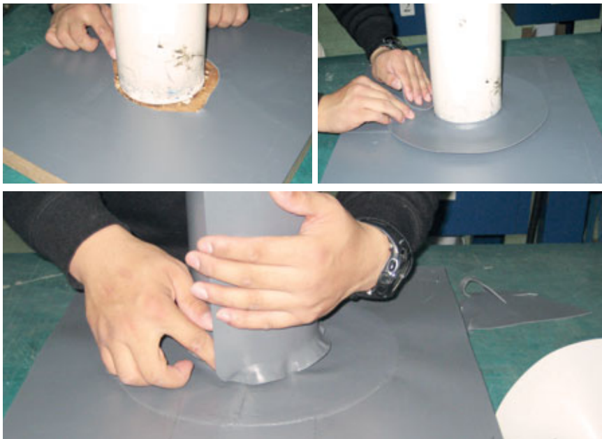
Fig. 12.12 – PVC coated strips for perimeter terminations.
