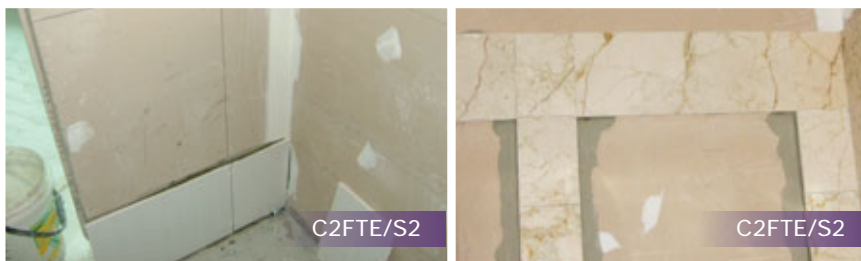
Fig. 5.3 – Installation of tiles and stones on partition board substrate.
