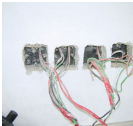
Fig. 13.17 – Adjusting position (after plastering and painting) leads to unpleasant consequences.
