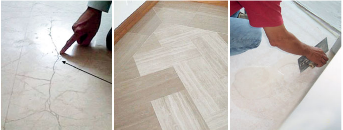
Fig. 1.12 – Difficult to address inherent flaws in natural stones, especially after installation.
