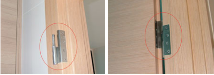
Fig. 10.7 – Hollow core door suitable for lift-off hinges door system because of its light weight.
