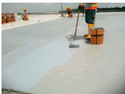
Fig. 12.1 – Application of liquid-applied membrane using roller.
