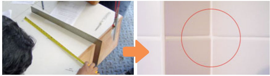
Fig. 3.4 – Size variation will lead to inconsistent joints.
