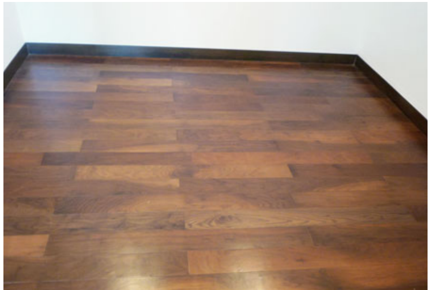
Fig. 8.3 – Engineered wood strips are generally more stable in dimension.
