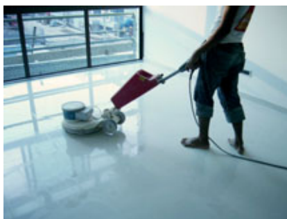
Fig. 7.5 – A topical wax coating on a marble floor, applied after the installation.
