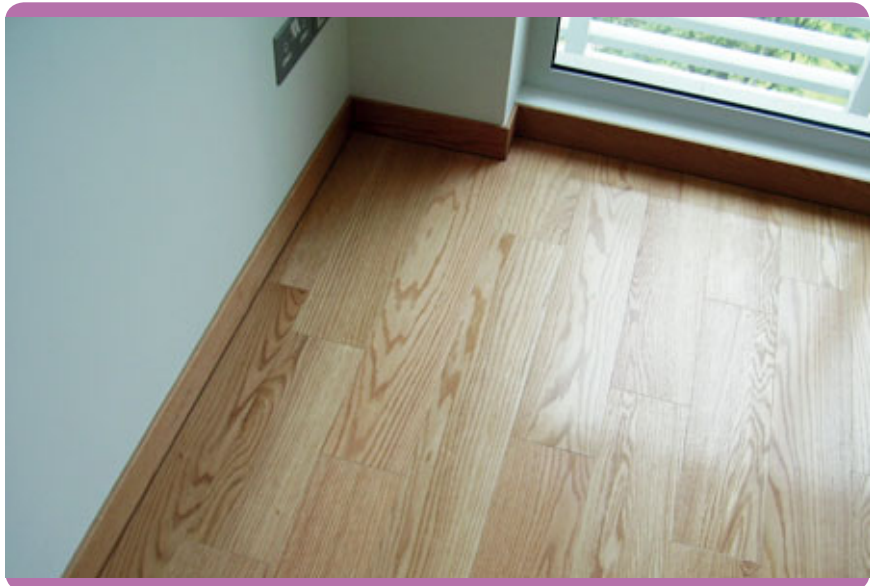
Fig. 8.4 – The controlled factory environment provides a uniform coating on the surface.
