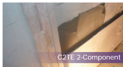
Fig. 5.4 – High water absorbent tiles with a substrate of cement render.
