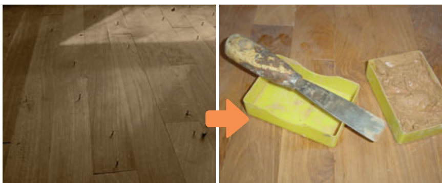
Fig. 8.7 – Nail-hole marks and patch-up often undermine the aesthetics of flooring.
