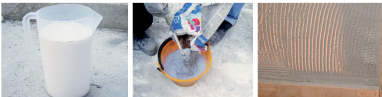
Fig. 5.8 – 2-component adhesive: Add powder + latex liquid.
