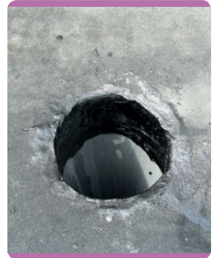
Fig. 12.9 – After laying the horizontal membrane around pipe penetration.
