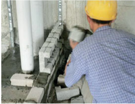
Fig. 13.3 – Recess formed to embed services without hacking wall.
