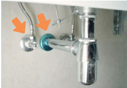
Fig. 13.15 – Permanent end caps for bottle trap and supply pipes conceal untidy work.
