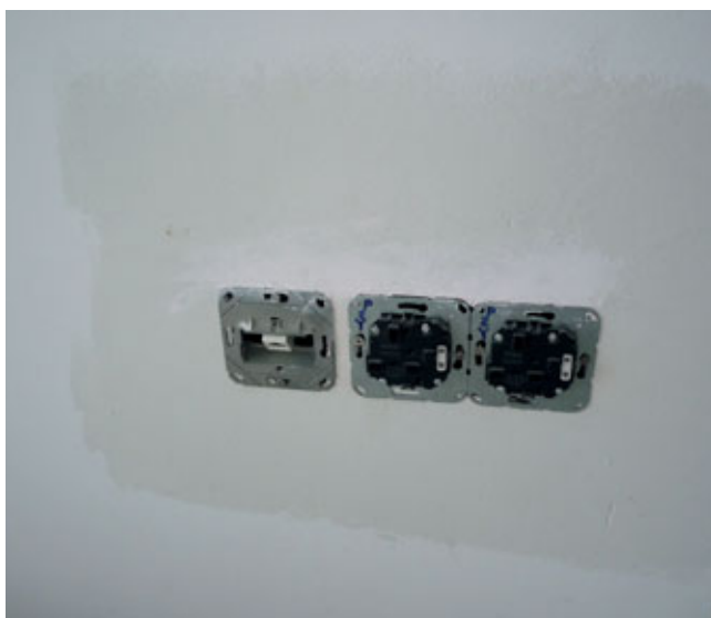
Fig. 13.19 – Waviness on the wall can be leveled with putty after the base plate installation.
