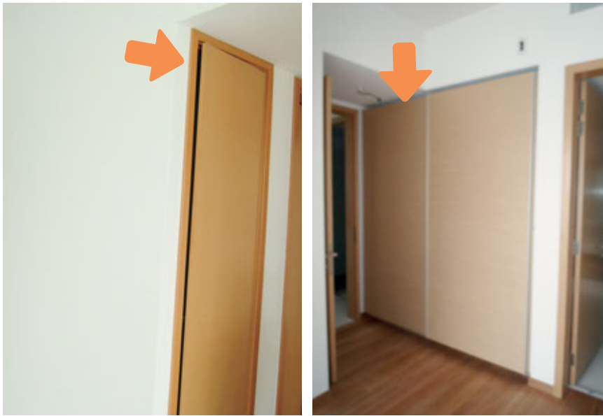
Fig. 10.3 – Warp or twist are caused mainly by expansion and contraction of timber.
