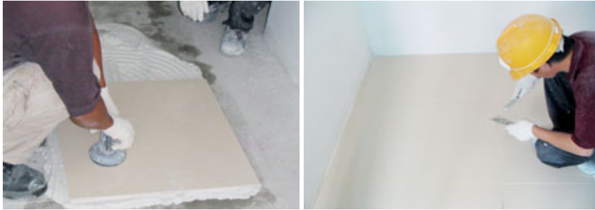
Fig. 1.17 – Use of compatible adhesive and grout enhances the performance of agglomerated marble.
