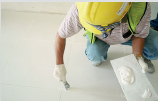
Epoxy joints for marble floor
