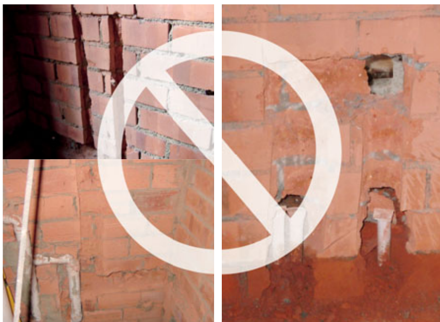
Fig. 13.1 – Hacking brick walls weakens the wall structure and is labour intensive.
