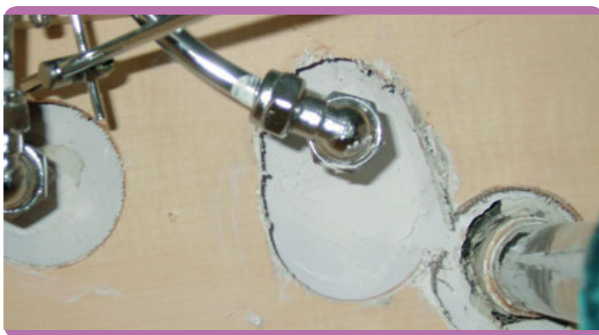
Fig. 13.14 – Untidy water supply inlets through vanity cabinet.
