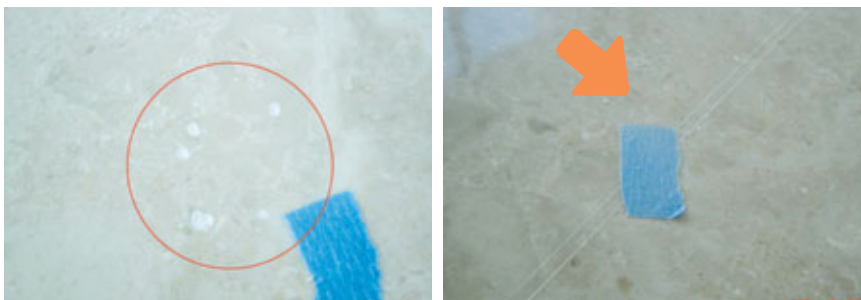
Fig. 1.15 – Scratches and damage by other trades during construction.
