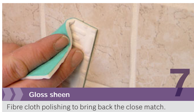
Fig. 9.7 – Sequences in ceramic tiles rectification.
