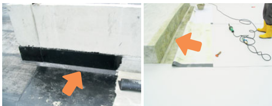
Fig. 12.5 – 25 mm fillets along parapet wall for bitumen and PVC membrane.
