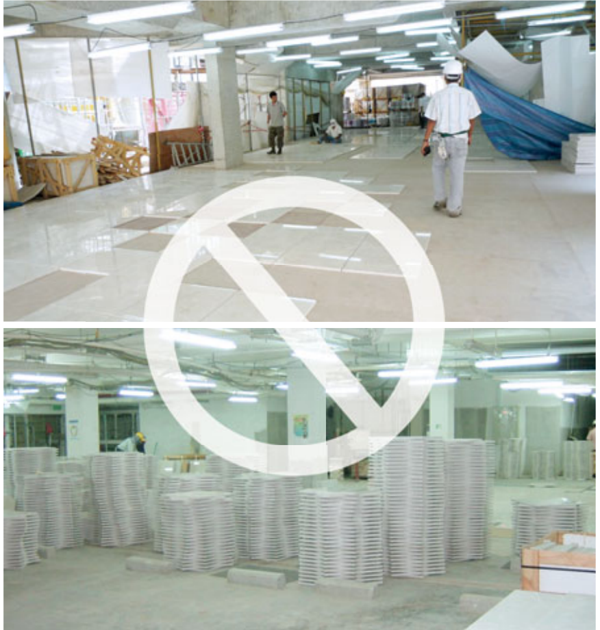
Fig. 1.8 – Dry lay requires additional manpower and sufficient space for segregation and storage.
