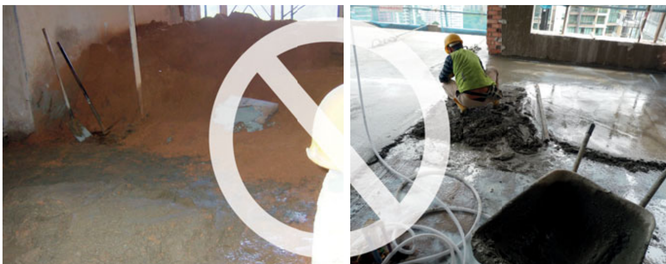
Fig. 5.9 – A typical conventional floor screeding process using cement-sand mortar.
