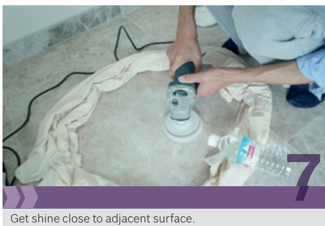
Fig. 9.2 – Sequences in marble rectification using epoxy fillers.
