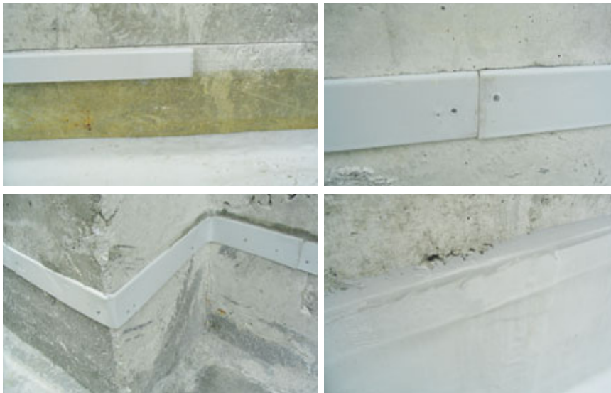
Fig. 12.10 – PVC coated strips for perimeter terminations.
