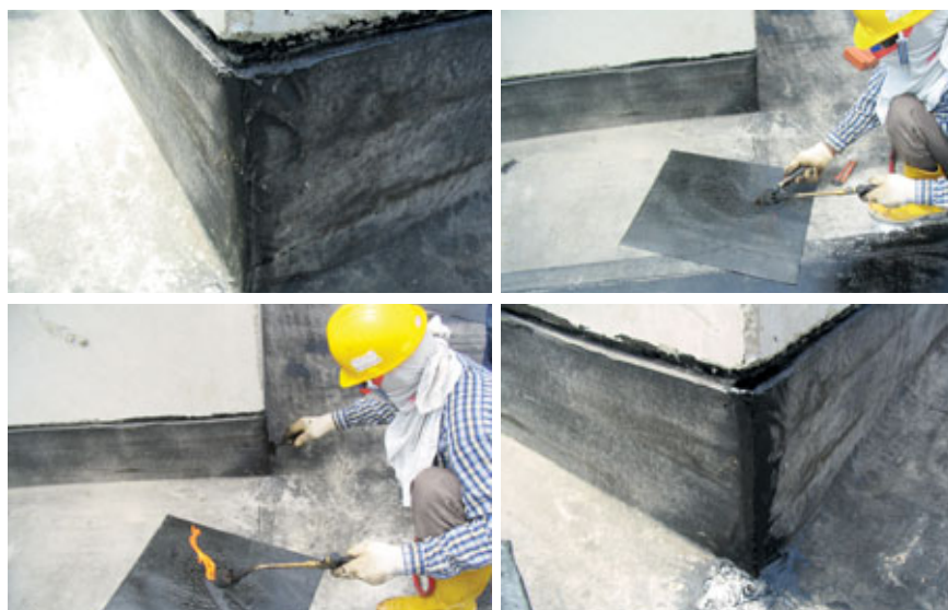
Fig. 12.7 – Overlapping and sealing at corner.
