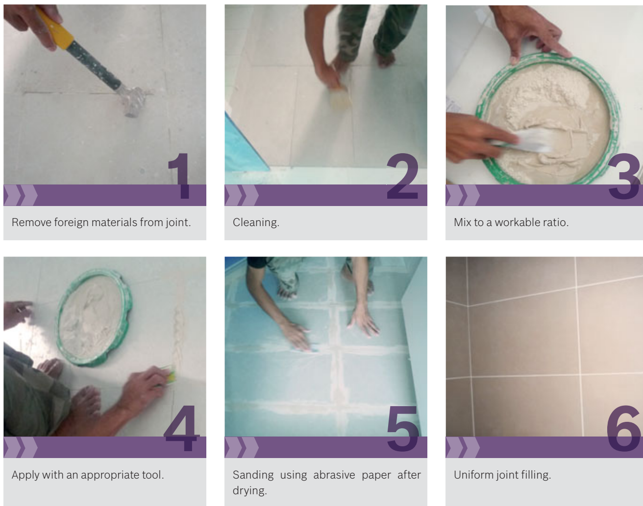
Fig. 6.2 – Application of grout in ceramic tiling.
