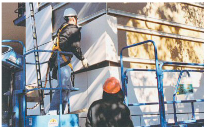
Fig. 4.2 – Lightweight panels and mechanical fastening installation expedite erection.
