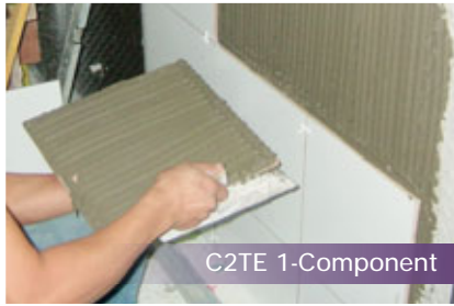
Fig. 5.5 – Tiles with low water absorption on a rendered substrate.
