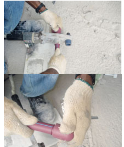
Fig. 13.10 – Fusion welding expedites connection process.
