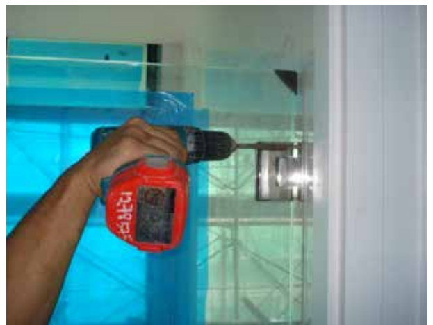
Replacement of shower screen
