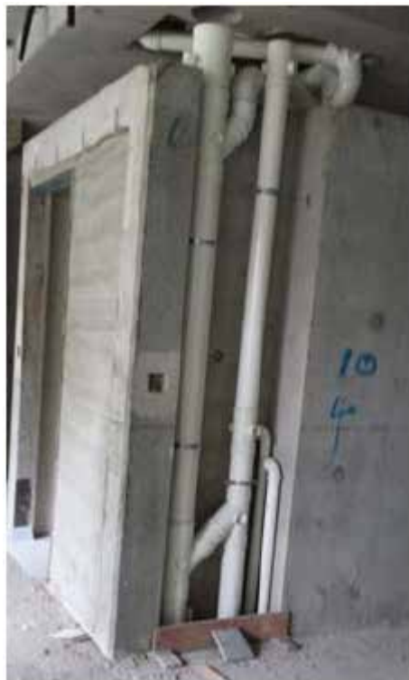
Example of an accessible stack pipe shaft
