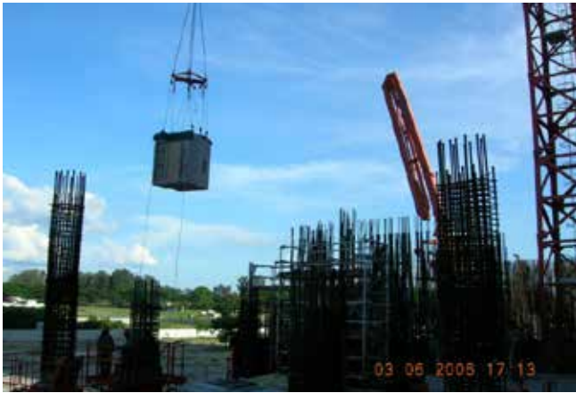
Hoisting of PBU
