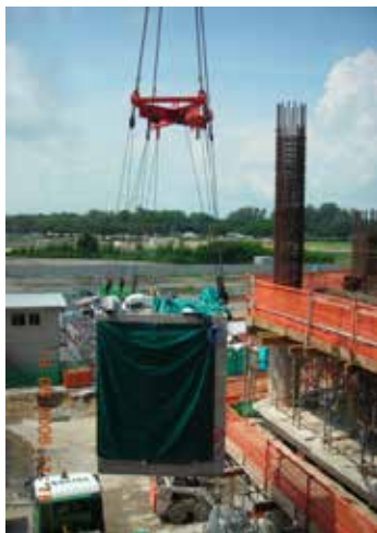
Protection (to remain) during hoisting
