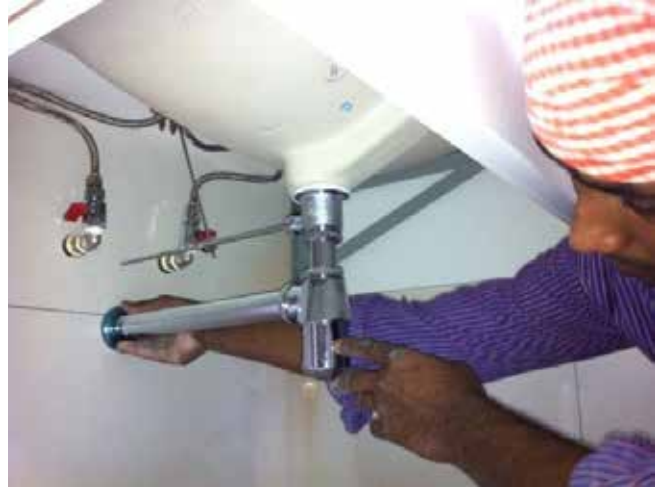
Replacement of M&E piping
