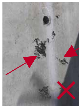
Demoulding defects
