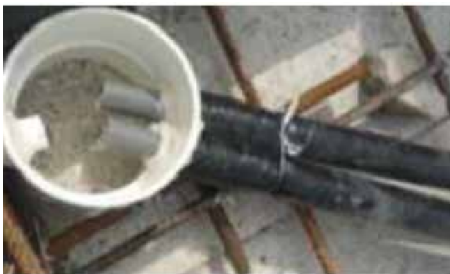
Cast-in air-con drain pipe
