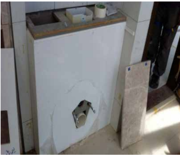
Horizontal connection to WC pedestal
