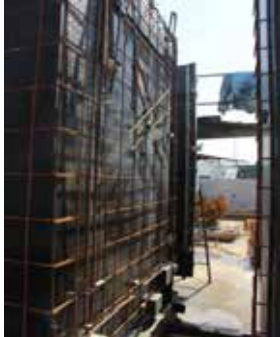
Install reinforcement bars
