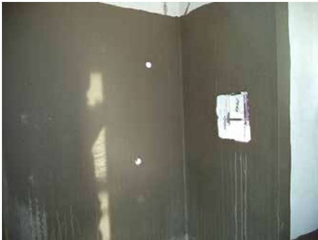
Waterproofing system must be tested before receiving architectural works
