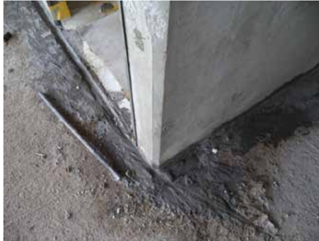
Grouting to gap between slabs (for double slab system)
