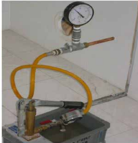
Pipe pressure test
