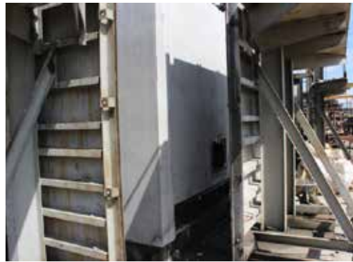
Demoulding & curing
