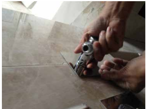
Connection of shower mixer tap on wall
