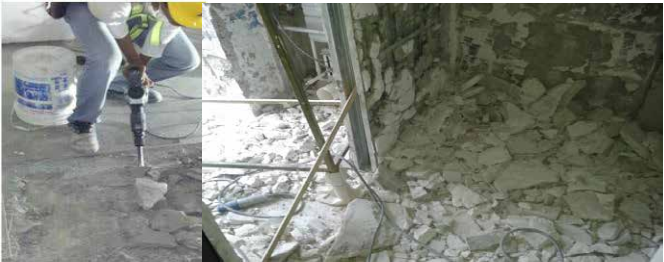
Use of breaker to hack tiles during renovation
