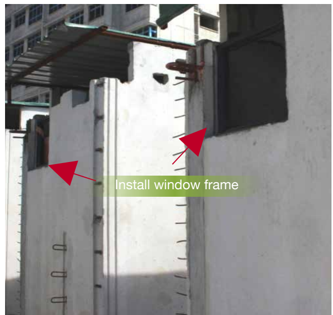
Door and window frame installation
