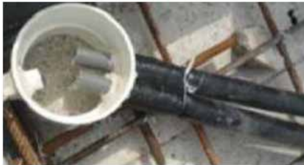
Cast in air-con drain pipe
