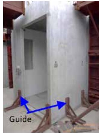
Positioning PBU (double slab system)
