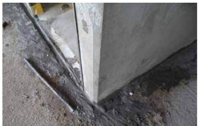
Grouting (double slab system)
