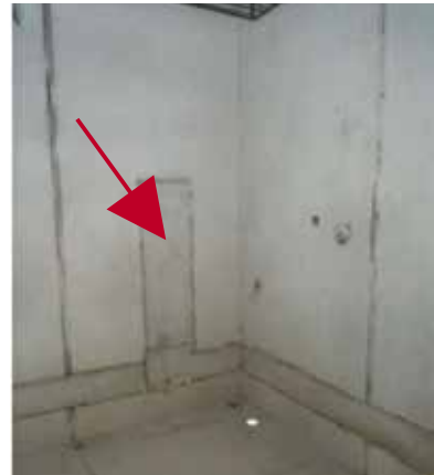
Recesses/block-outs provided for services
