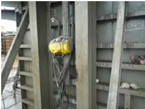
Use of vibrating system to achieve concrete uniformity
