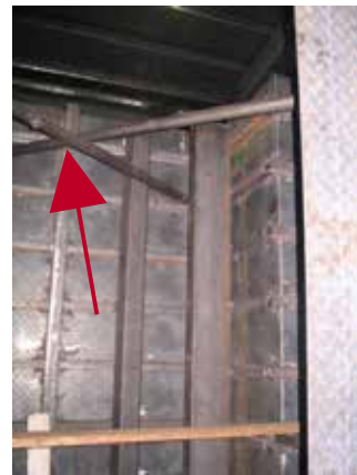
Props to formwork
