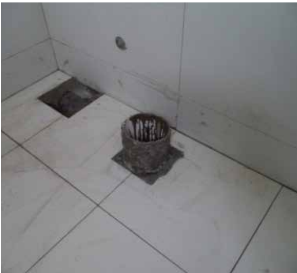
Vertical connection to WC pedestal
