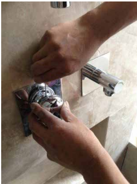
Replacement of shower mixer tap
