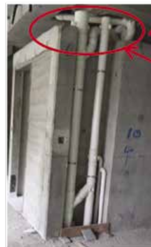
Example of vertical soil stack accessible from within dwelling unit
