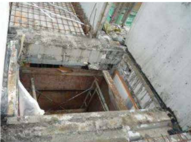
Perimeter beams for seating PBU
