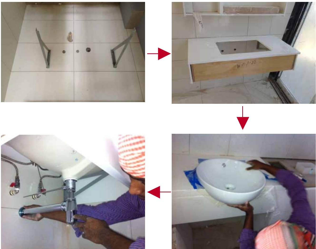
Connection and installation of wash basin
