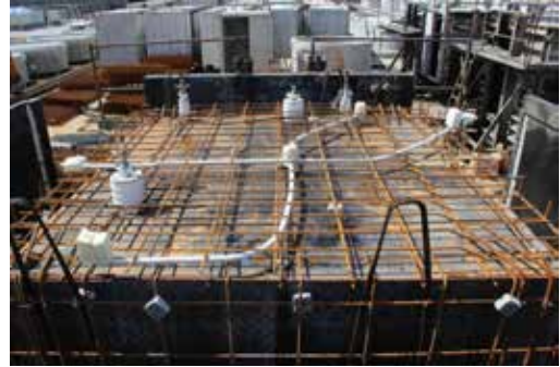
Install M&E embedded services
