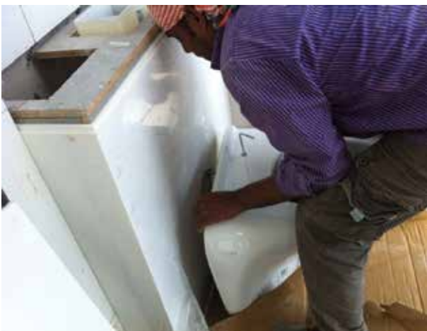
Replacement of sanitary ware
