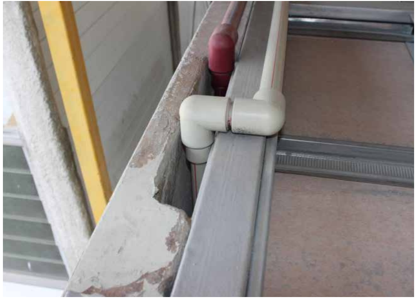
M&E concealed services routing through precast block-out
