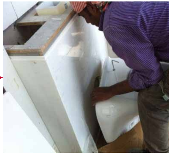
Horizontal connection to WC pedestal
