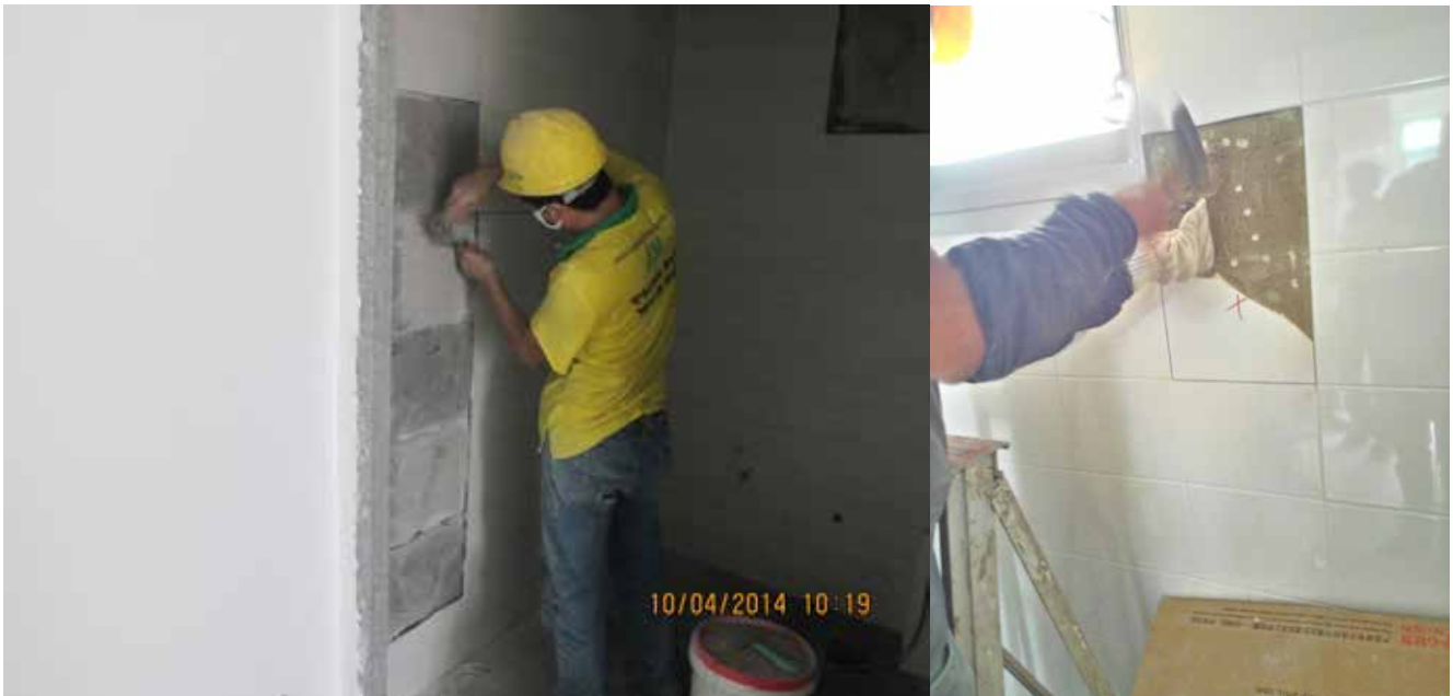
Hammer and chisel method used for replacement and maintenance work
