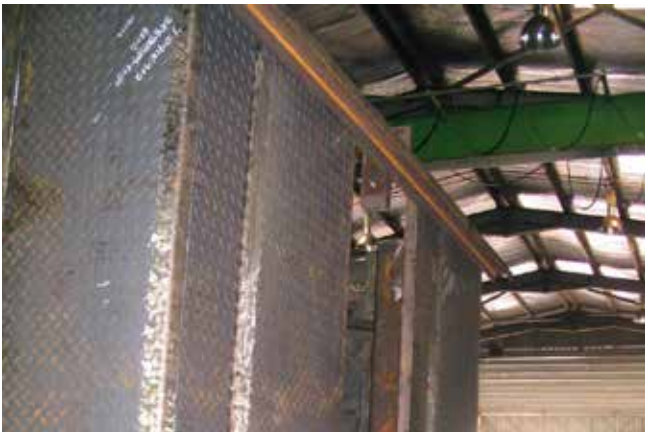
Use of checker plate formwork
