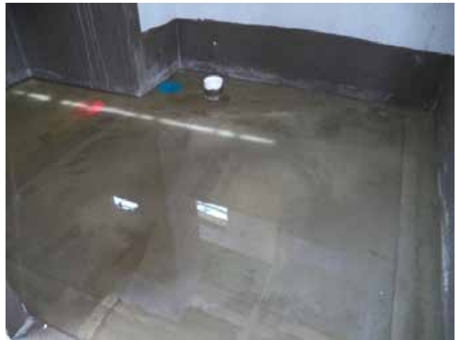
Waterproofing system must be tested before receiving architectural works
