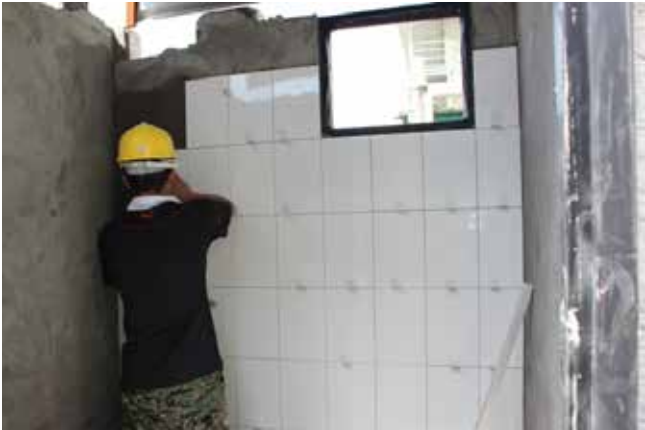
Tiling works installation
