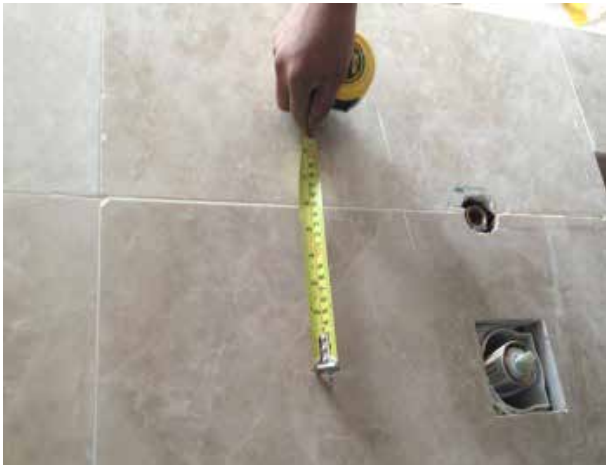
Connection of shower mixer tap on wall
