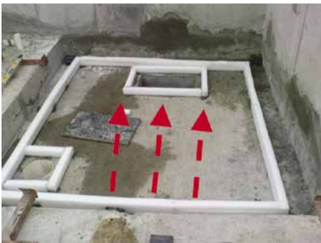
Structural design of the secondary slab has to incorporate a gradient to an outlet at the lowest point for drainage.
