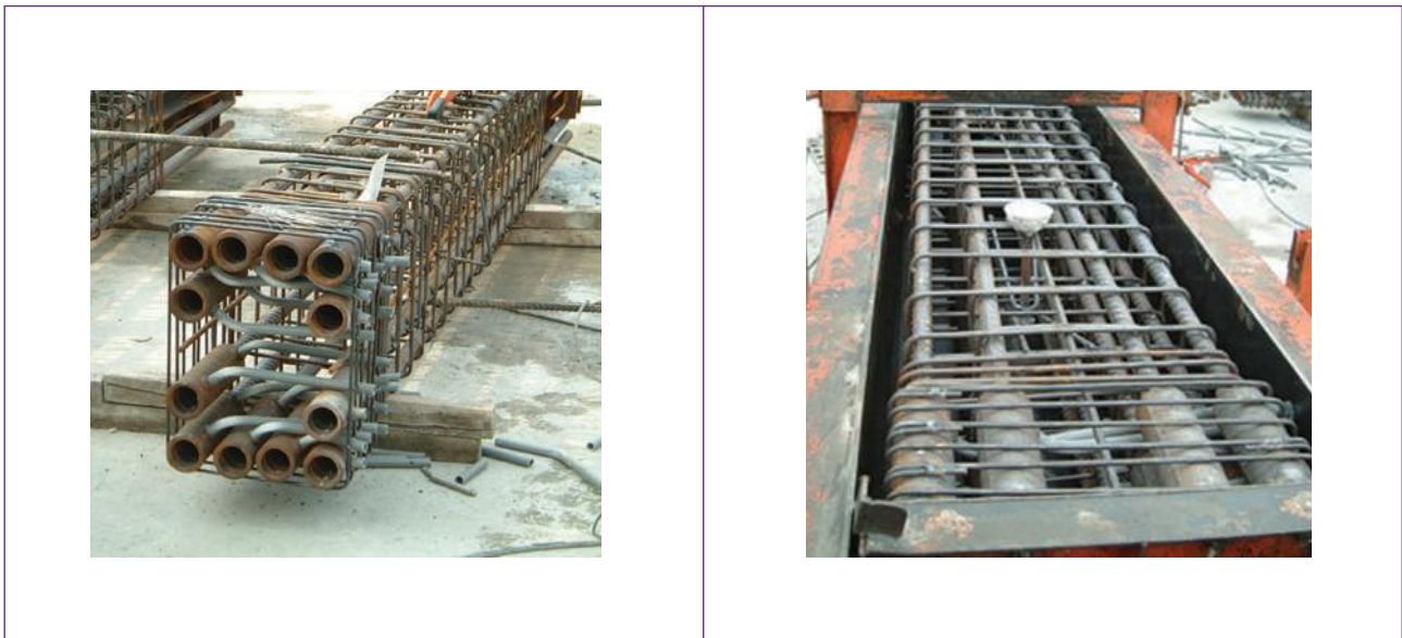
Figure 2.5 Use of splice sleeve system in place of long projecting reinforced bars
