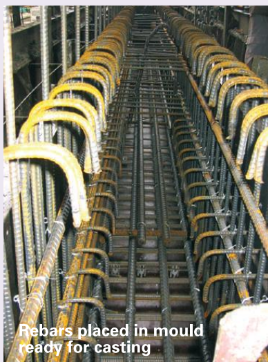
Placing the beam cage to the mould
