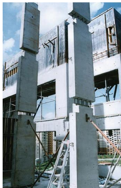
Figure 2.2 Multi-tier columns
