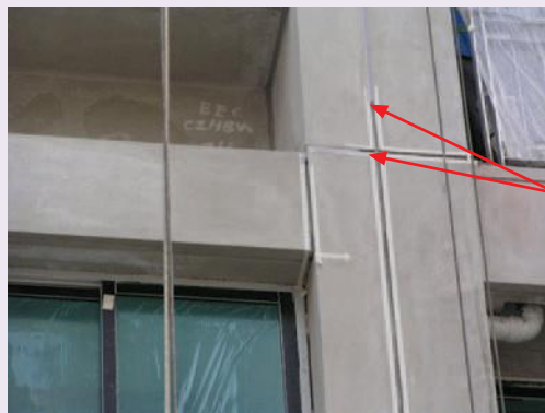
Consistent joint gap to for proper sealant or grout installation
