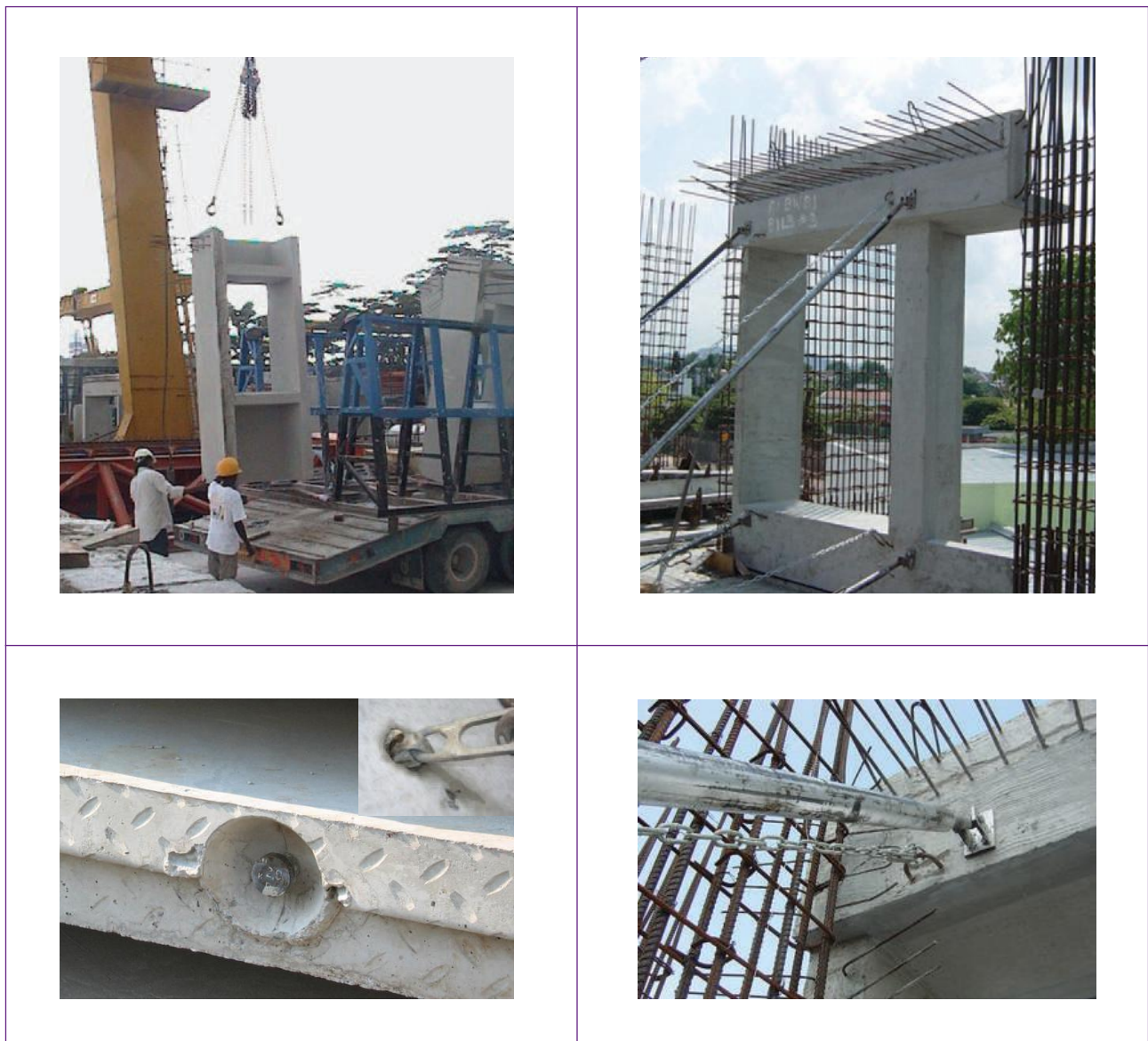
Figure 2.10 Lifting and handling devices are required to facilitate the erection process
