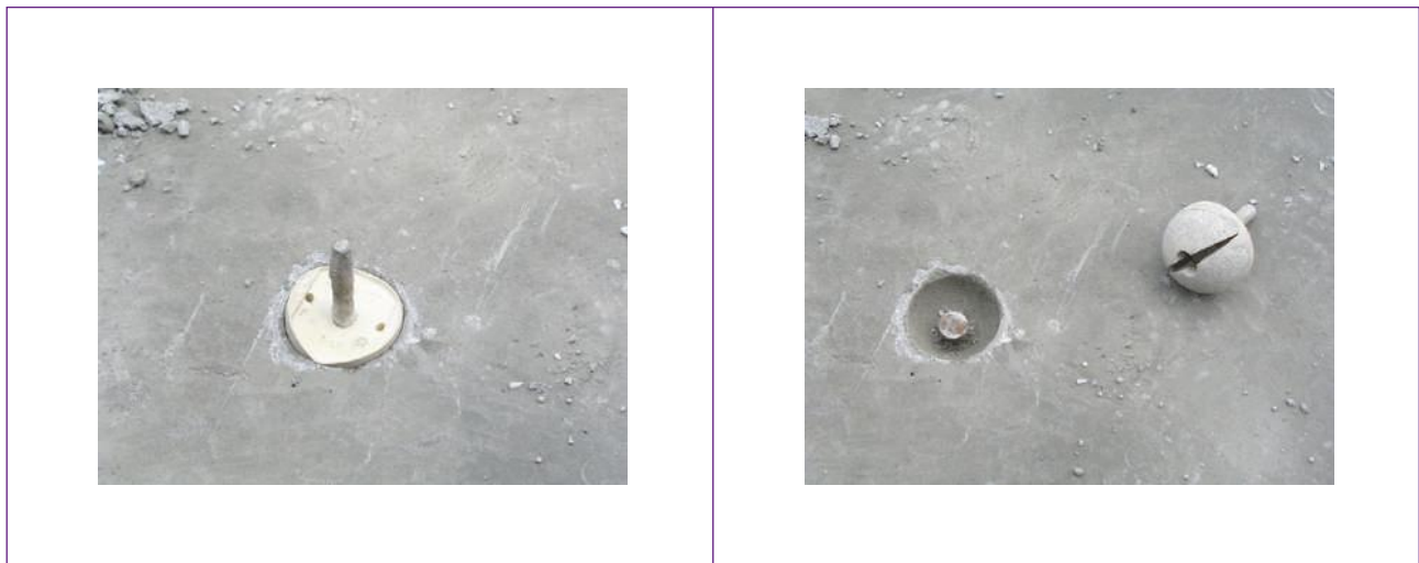
Figure 2.12 Provision of lifting anchor with recess former for better finishes
