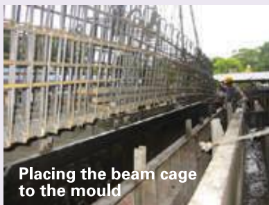
Beam reinforcement cage
