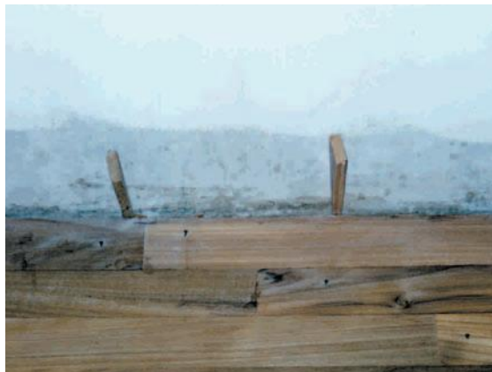
Expansion gap at the perimeter of room
