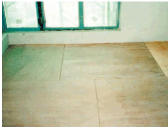
Layout of plywood sub-base in a staggered manner
