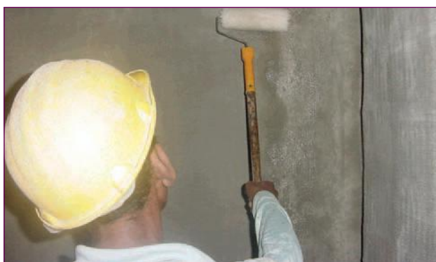
Dampen wall surface with wet roller
