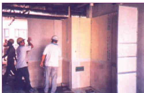
Figure 2.4: Prefabricated finished walls separately lifted and assembled on site
