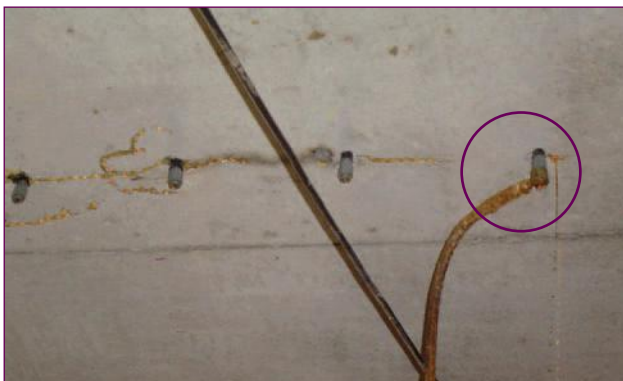
g) Grouting in progress
