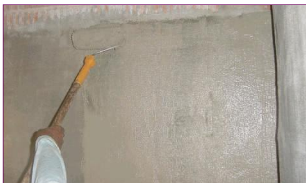
Roller application to wall
