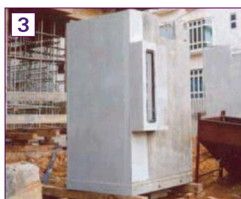
3 Precast concrete bathroom with pre-finished concrete external wall
