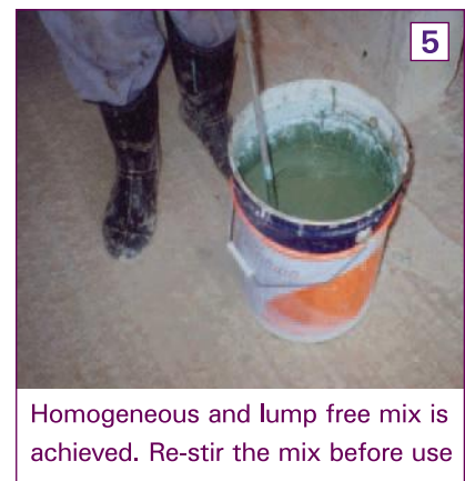
Figure 6.4: Mixing of 2-component waterproofing products
