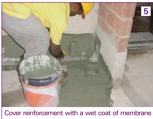
Figure 6.6: Application of waterproofing membrane around wall-floor junctions
