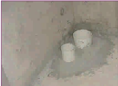
Figure 5.6: Fillet installed around pipe penetrations
