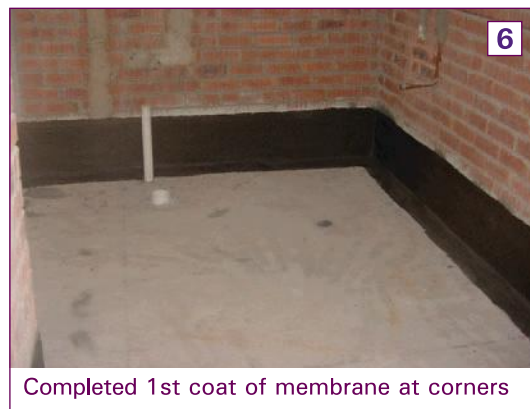
Figure 6.6: Application of waterproofing membrane around wall-floor junctions
