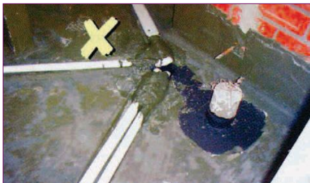
Poor arrangement of pipes
