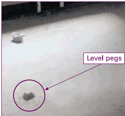
Figure 7.5: Level pegs
