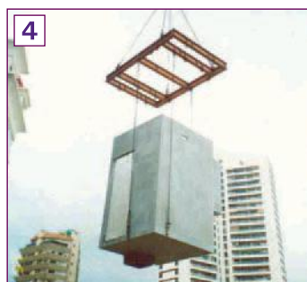
4 Hoisting of precast bathroom
