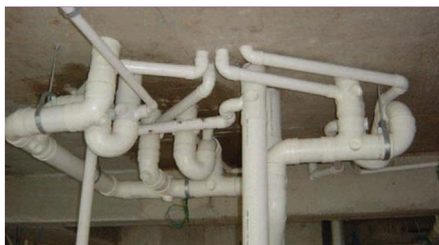
Recommended arrangement of pipe connections below the slab
