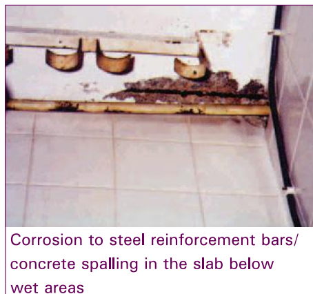
Figure 8.2: Common defects arising from leaks
