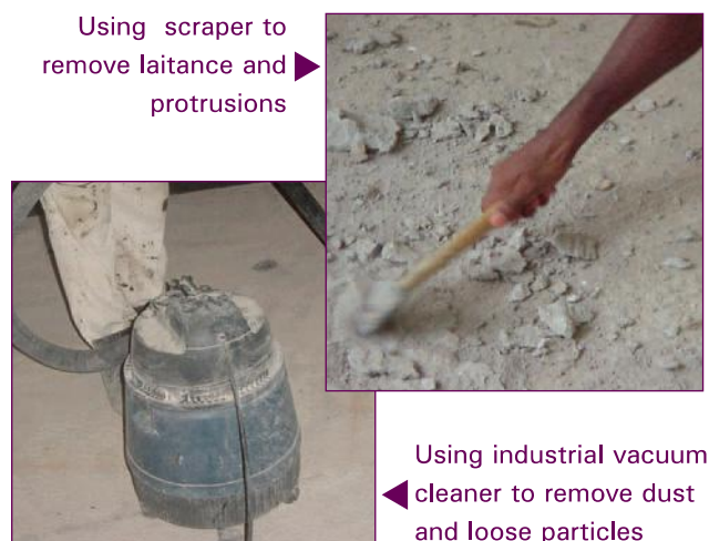
Figure 5.3: Examples of concrete surface cleaning methods
