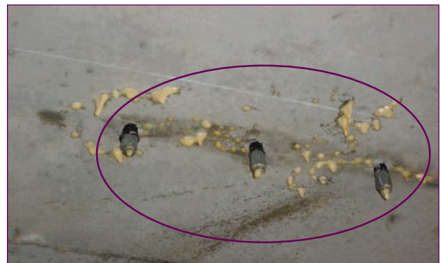
h) Fully grouted crack line
