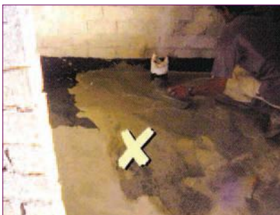
Figure 6.2: Apply using steel trowel
