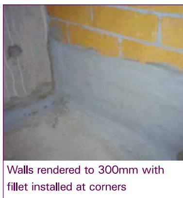
Figure 5.4: Surface preparation to brickwalls and internal corners
