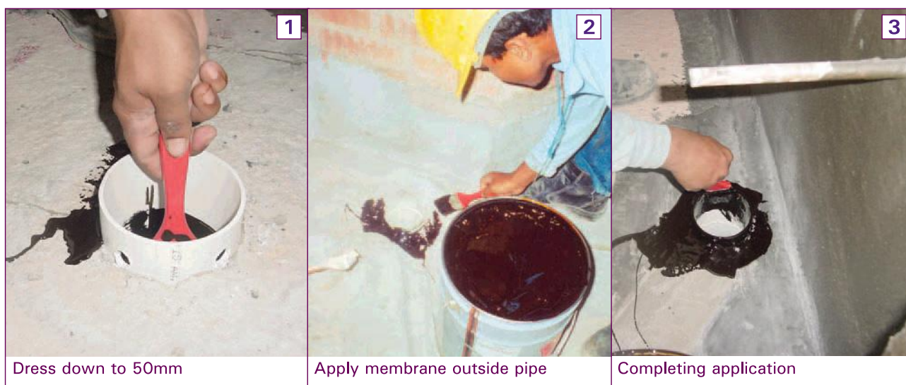
Figure 6.8: Application of membrane at floor outlet
