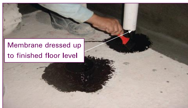
Figure 6.7: Application of membrane at pipe penetrations
