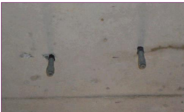
e) Nozzles inserted along crack line
