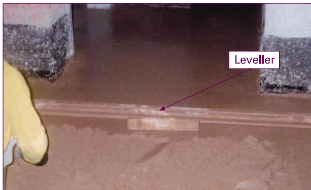
Figure 7.6: Screeding in progress
