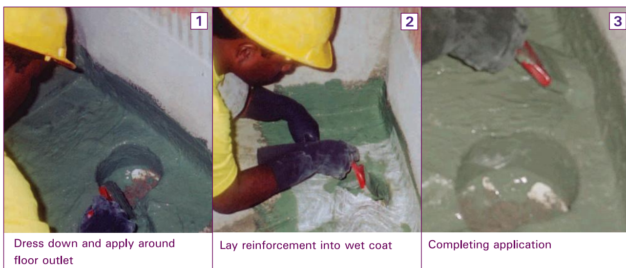
Figure 6.9: Application of membrane at floor outlet (with reinforcement)
