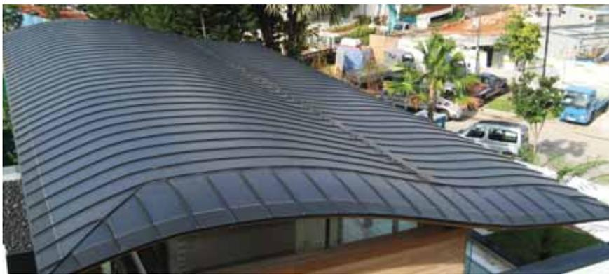
[Figure 17] Flexible amorphous silicon laminates glued to a curved metal roof (Sentosa Cove).
