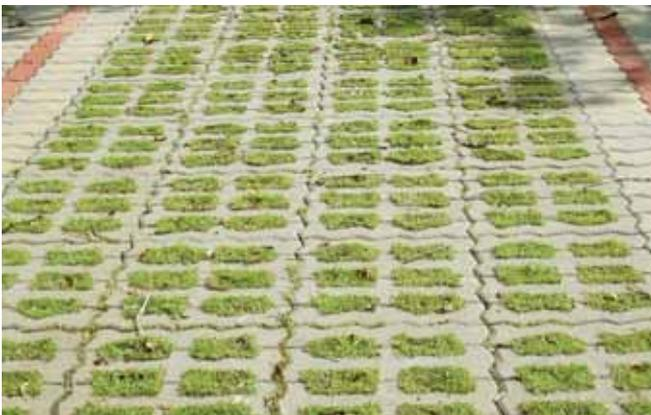
*[Figure 4] Open grid carpark paving.*
