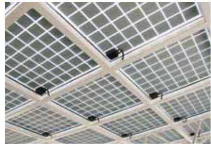
[Figure 15] Crystalline silicon BIPV modules integrated into a skylight canopy (Savannah Condo).
