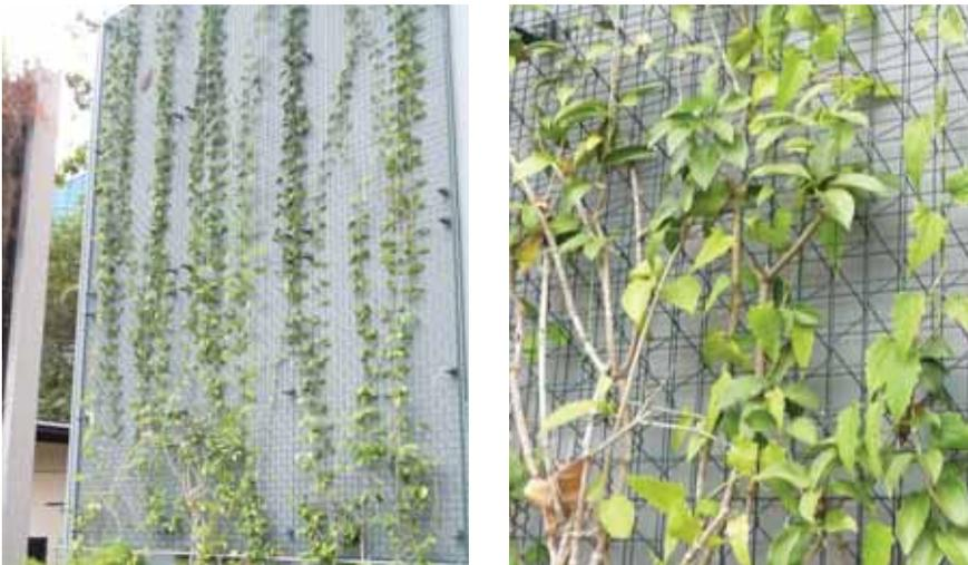
[Figure 9] The modular trellis panel system (left) and its close up (right).
