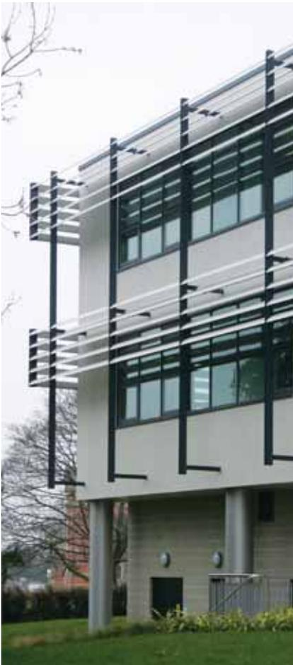
There have been design schemes that considered venting air-conditioning through this cavity but the quantities involved would increase energy to pull fresh air into the building. Furthermore, the energy spent to dehumidify this heated air would more than offset the savings from the reduced heat load.
