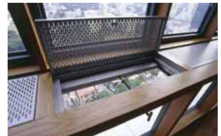
[Figure 21] Monsoon windows allow wind movement into the unit without allowing rain to penetrate into the unit.
