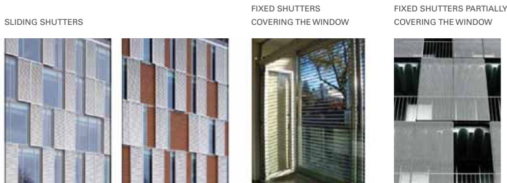
[Figure 3] Different types of shading devices.
