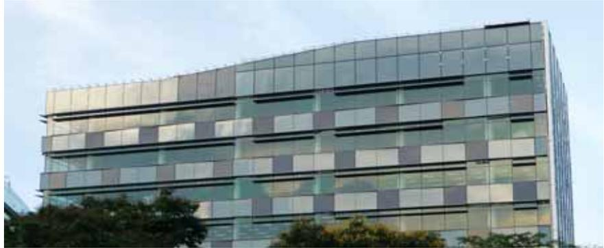
[Figure 14] Amorphous silicon BIPV modules (dark squares) integrated into a façade (No. 7 Tampines Grande).
