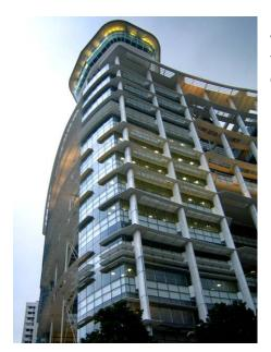
For the façade, prefabricated, unitized curtain walling was adopted for the majority of the floors, which delivered high quality finishes with good construction speed.
