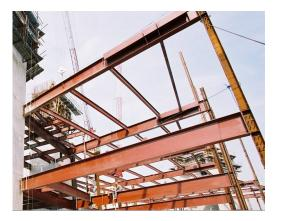
A transfer steel plate girder was provided at the third and fifth storey to provide column free space for the ground floor atrium.
