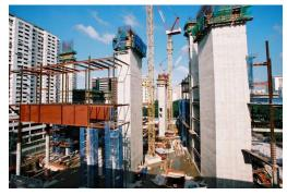
For the project, fire safety engineering was implemented to reduce the large amount of fire proof material to be used on steel structure. As one of the first structures in Singapore to have its composite steel structure designed using performance-based fire safety engineering, the design does not rely on strict adherence to prescriptive building codes.
