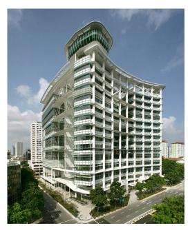
The superstructure is designed with steel structure and metal decking. No temporary scaffolding was required to support the slab during construction. The metal deck acted as the temporary formwork and at the same time as the permanent slab, thus providing quick access for the construction of slab.
