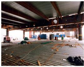
For the typical floor, the structural system adopted comprised a steel framed construction with beams spanning the full 26m span in one direction and secondary beams at the transverse direction. The floor was made up of 130mm thick Bondeck composite deck. This composite steel-concrete form system was efficient system where the steel decking acted as a formwork and also served as slab reinforcement to the concrete in the composite slab.
