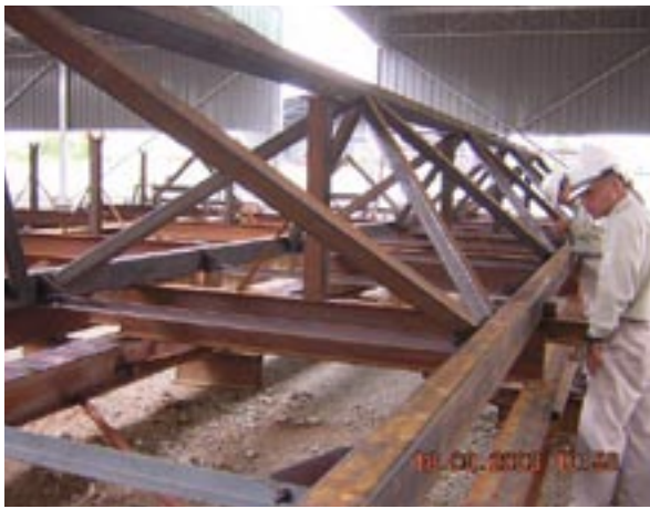
Cold formed hollow sections used at Changi Airport Terminal 3 roof structures
