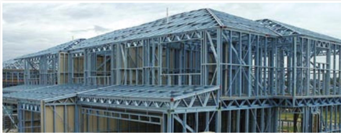
Light gauge steel frame used in the construction of landed houses
