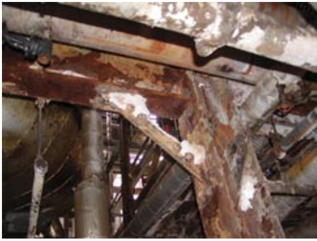
Corroded steel sections
