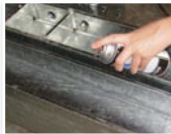
Stage 3: Repair uncoated areas using zinc thermal spray or zinc rich primer
