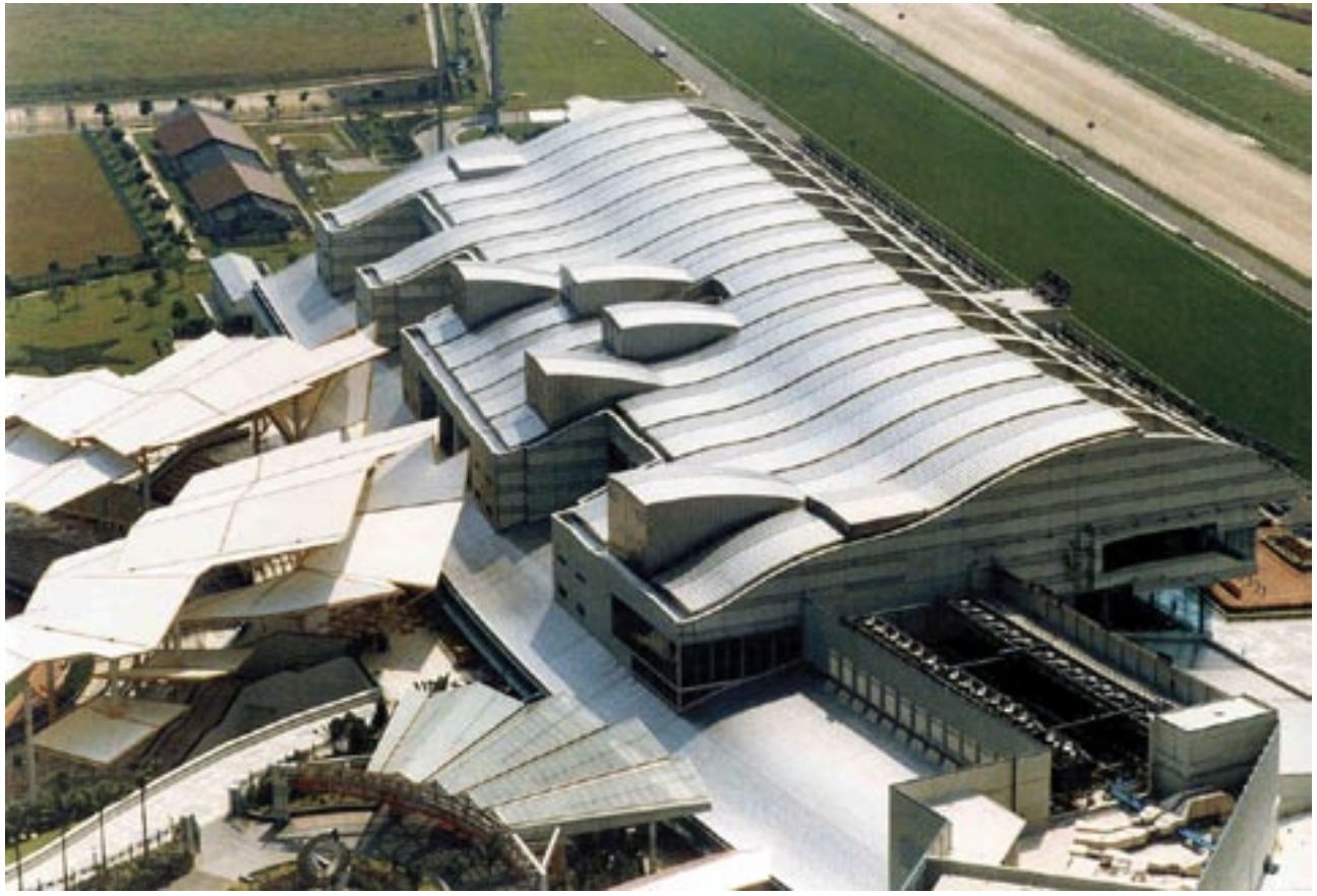
Stainless steel is rarely used for structural steel but used mostly for roofing, claddings and other internal applications. Photo of Kranji Racecourse taken by Chadwick Technology
