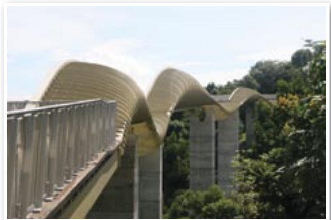
The steel sections at the Henderson Waves are coated with a polysiloxane topcoat
