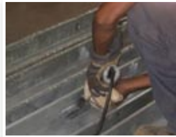
Stage 2: Surface to be repaired is cleaned by grinding
