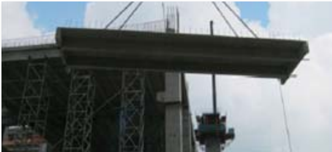
Pic.36 DOUBLE T-SLAB PRECAST BEING HOISTED UP FOR INSTALLATION
