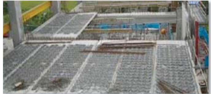
Pic.35 COBIAX HALF PRECAST SLAB AFTER PLACING ON THE BEAMS AND READY TO RECEIVE CONCRETE TOPPING UP
