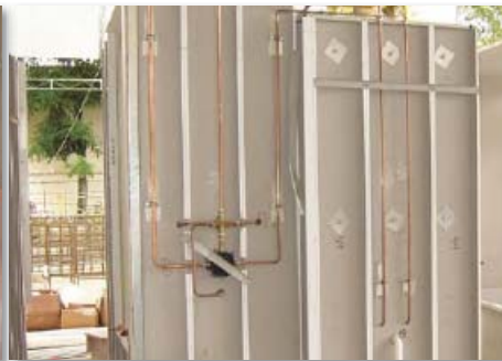
Pic.8.5 METAL PANELS MOUNT ON WALL TILES
