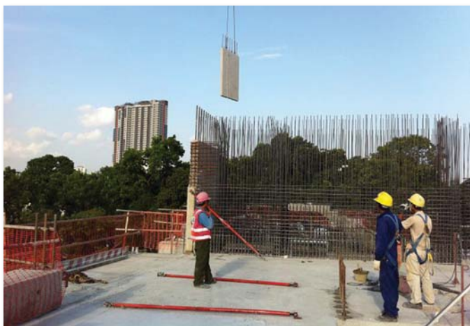
Pic.23 LIFTING OF PRECAST WALL
