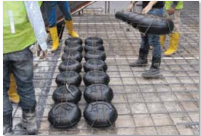
Pic.19 INSTALLATION OF COBIAX MODULES
