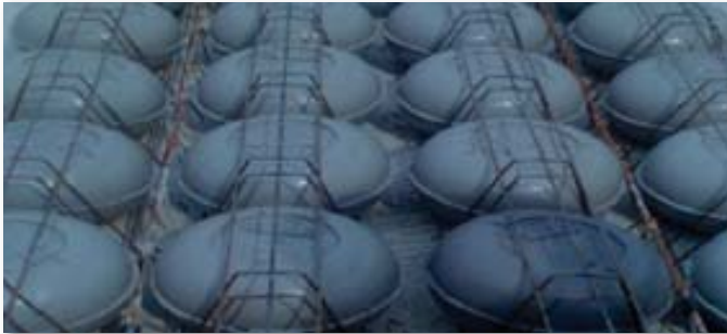
Pic.34 POSITIONING OF COBIAX MODULES
