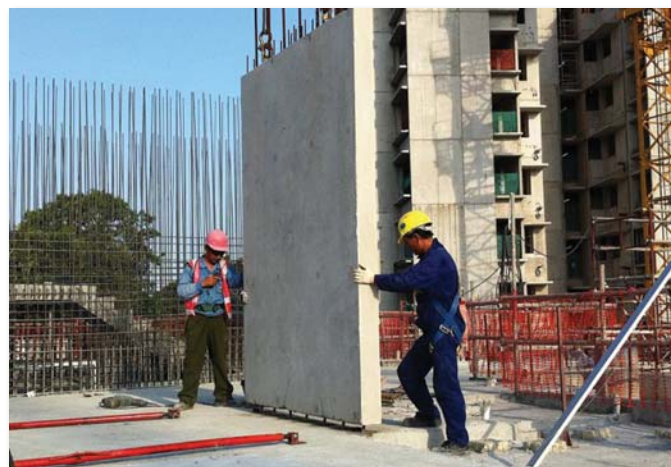
Pic.24 POSITIONING OF PRECAST WALL
