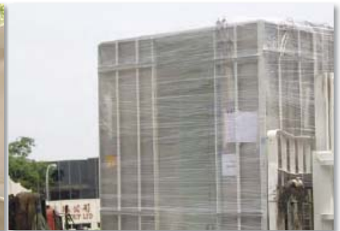
Pic.8.6 METAL PANELS MOUNT ON WALL TILES
