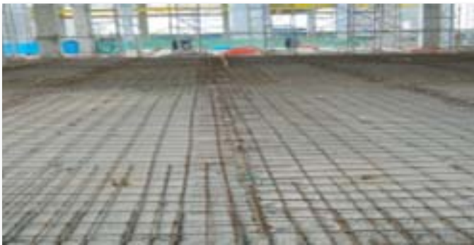
Pic.38 DOUBLE T-SLAB PRECAST REBARS INSTALLATIONS AND READY TO RECEIVE CONCRETE TOPPING UP
