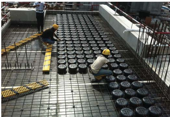
Pic.21 LAYING OF COBIAX IN PROGRESS
