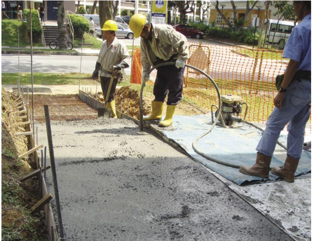
Figure 20. HDB Walkway being cast with Eco-concrete
