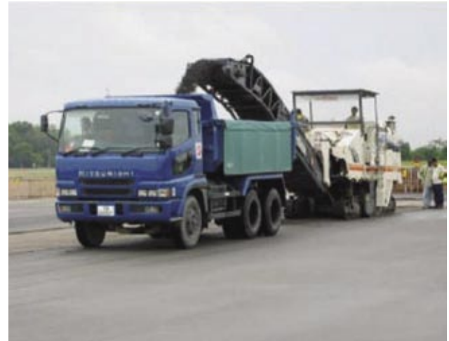
Figure 14. Milled waste from resurfacing of roads
