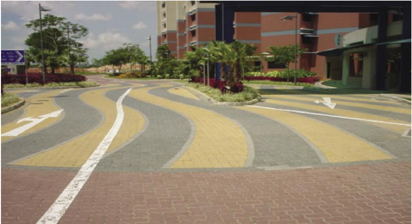
Figure 27. Concrete pavers at residential area
