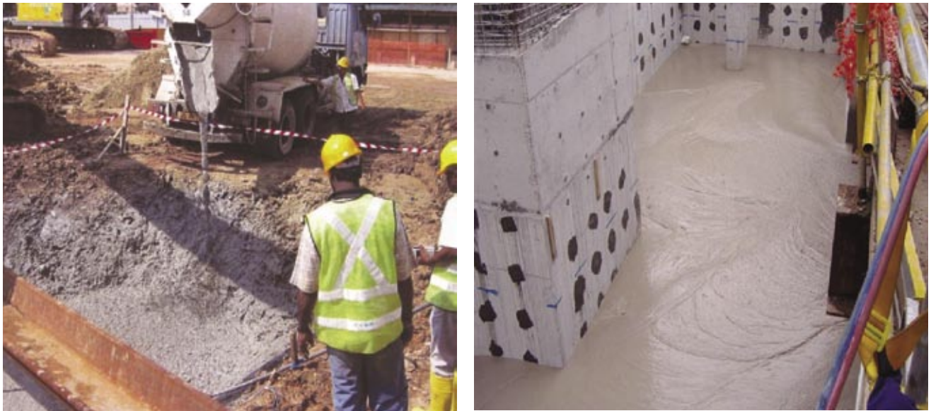
Figure 35. Self-compacting, highly flowable liquid soil
