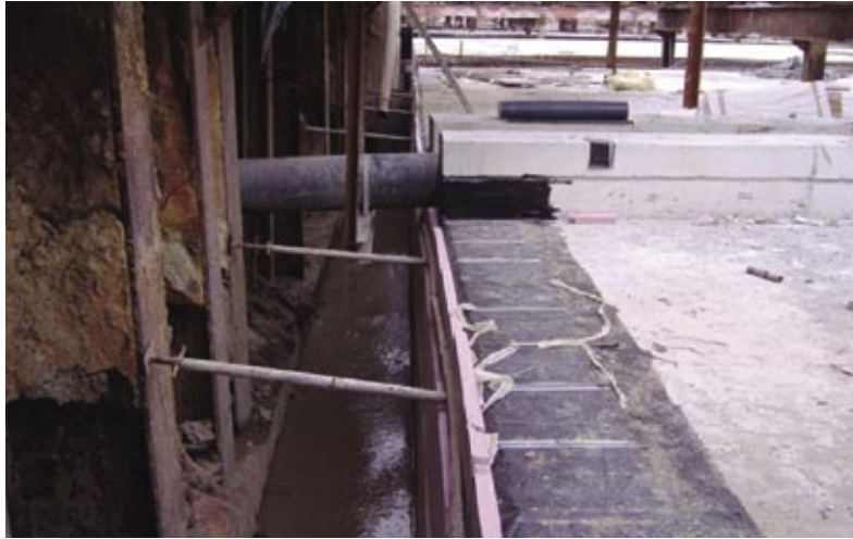
Figure 36. Support between sheet pile and tunnel wall
