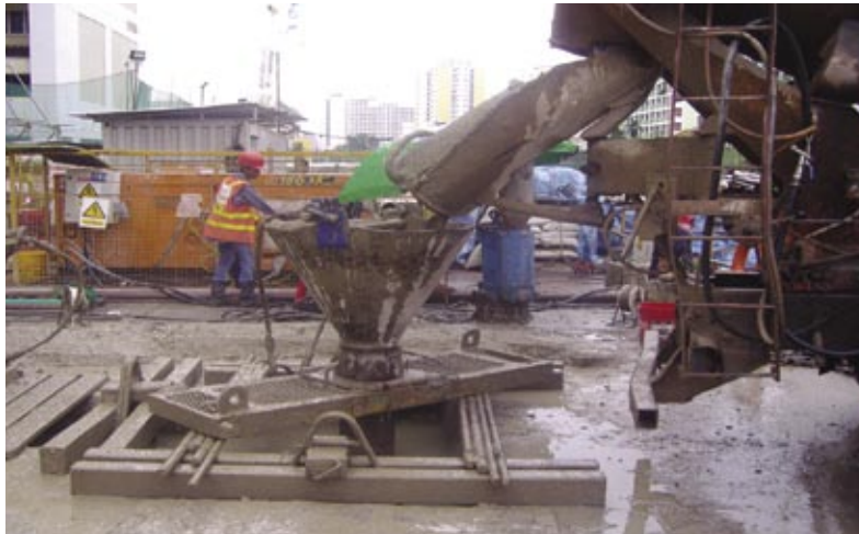
Figure 37. Filling up diaphragm walls from the top with liquid soil
