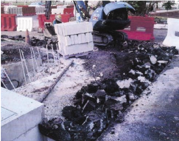
Figure 13. Asphalt pavement machine-milled by breaker
