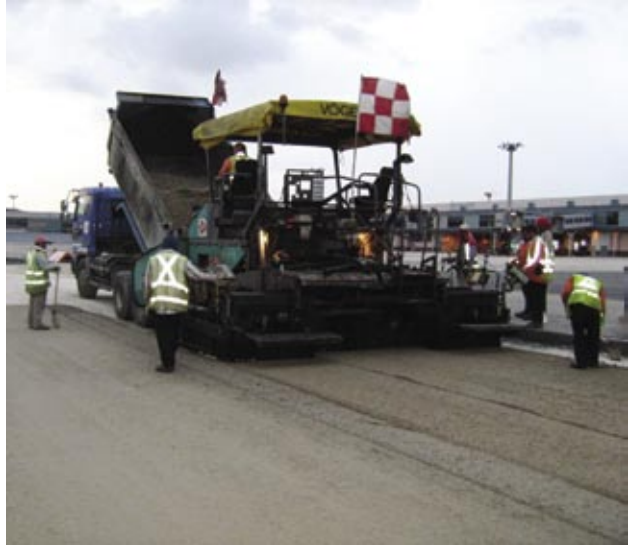
Figure 30. Paving of the base course with RCA for taxiway
