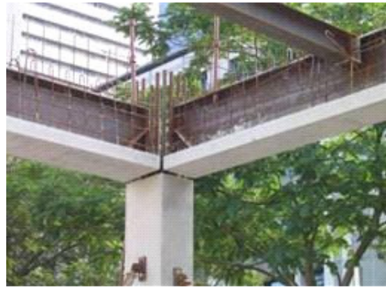
Prefabricated composite columns and beams
