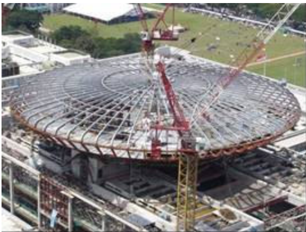
Aerial view of the shell roof
