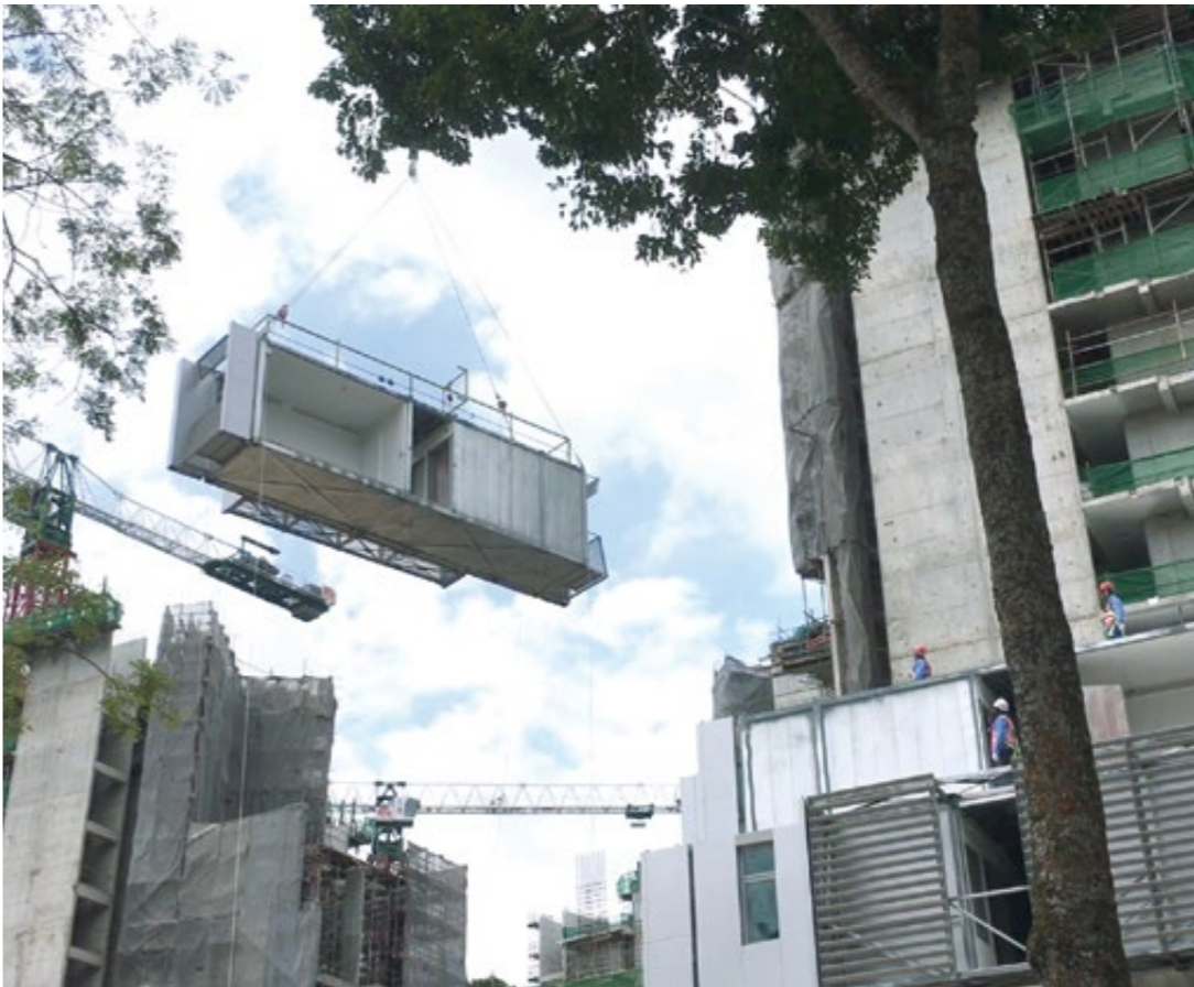
Prefabricated Prefinished Volumetric Construction is an example of DfMA technology
