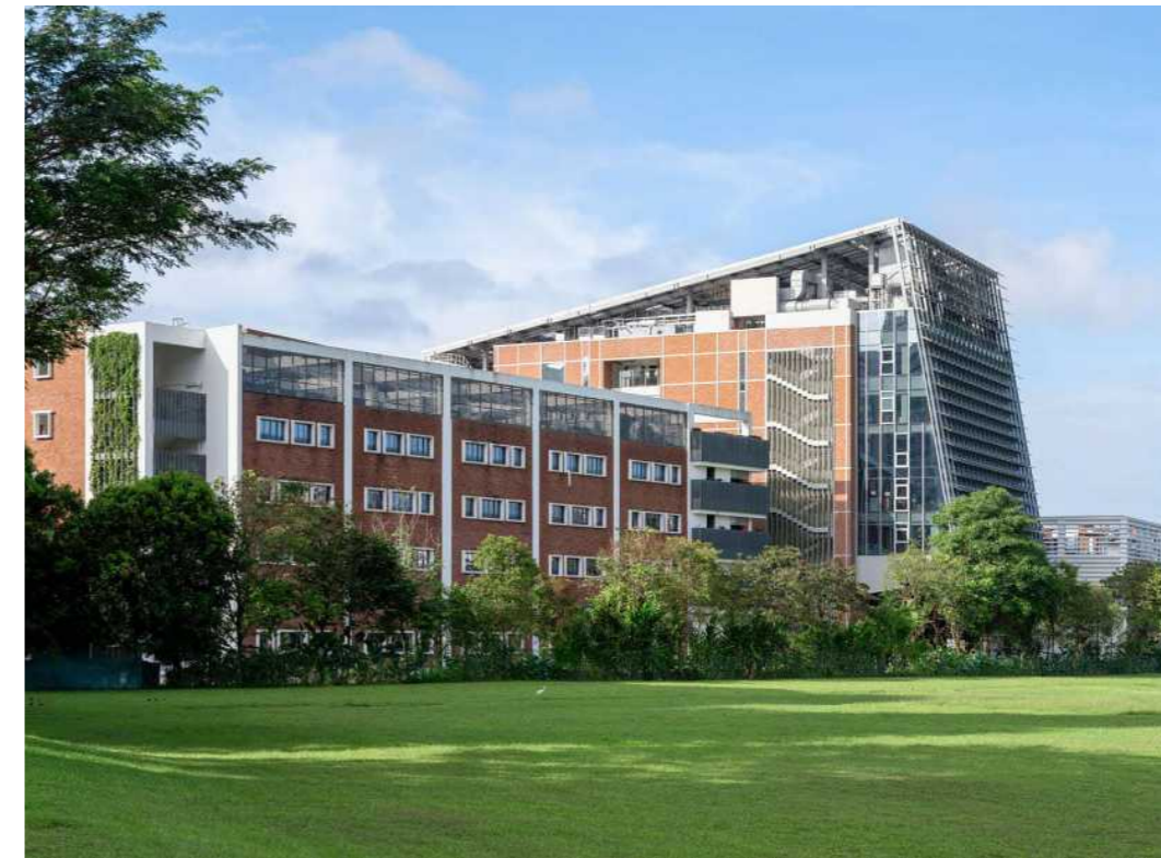
The Dulwich College (Singapore) demonstrated good DfM and incorporated smart features from the design stage, such as an Integrated FM platform with a unified dashboard for asset performance and operations.
