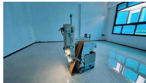
BEAMP alumnus Fabrica AI secured a commercial contract for their automated floor tile grouting robot to be deployed at a construction project.
