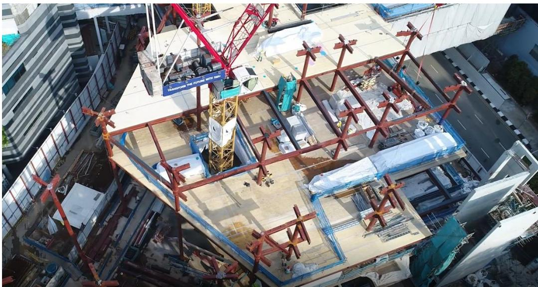
Er. Kam and the project team also had to overcome the challenge of constructing a two-storey link building over Fort Canning Link carriageway which had to be temporarily closed for the building works to take place. The project team had to erect the structure quickly and safely, while minimising disruptions around the area. This was accomplished using a similar hybrid steel-CLT slab solution. As such, the
