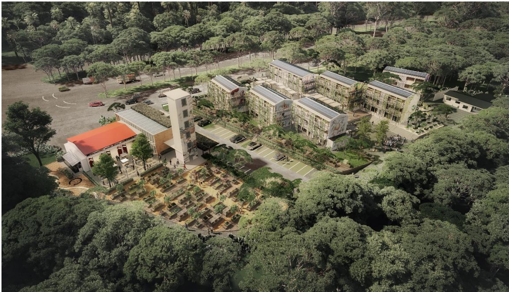
An aerial view of the former Bukit Timah Fire Station community node with a mix of lifestyle, food, educational and entertainment offerings, as well as generous public spaces © Homestead Holland Pte Ltd
