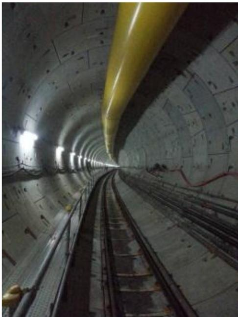
Steel Fibre Reinforced Concrete (SFRC) bored tunnel precast segmental lining was adopted for the Land Transport Authority Downtown Line Stage 3 project.
