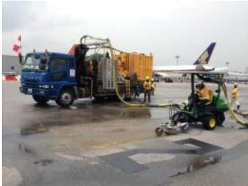
Using the water blasting method, the firm is able to remove pavement markings without the need to grind and damage the road surface.
