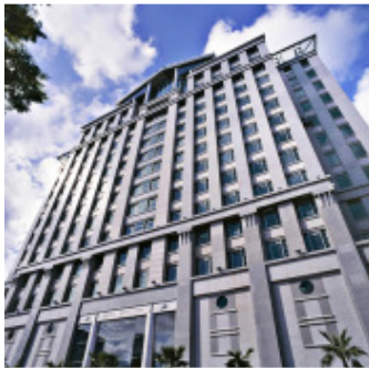
Bugis Junction Towers, Platinum, 2014
