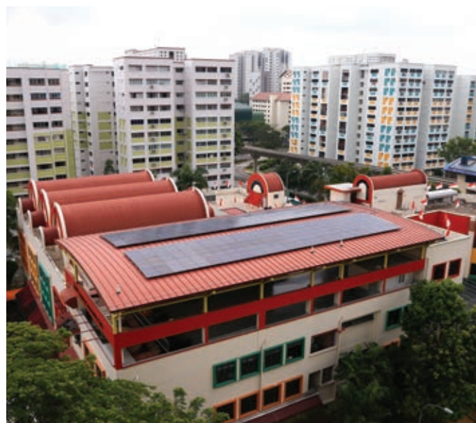
Figure 12: Solar panels helped to provide 20% of energy required by Bukit Panjang community centre.
