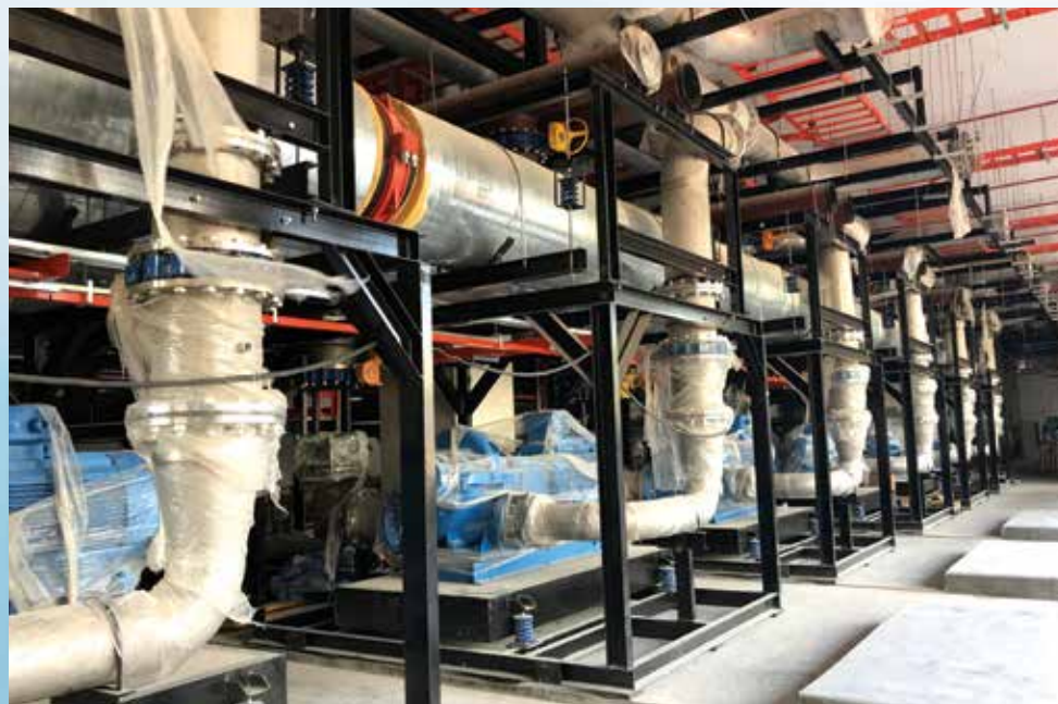
An example of header and pump modules in the chiller pump room
