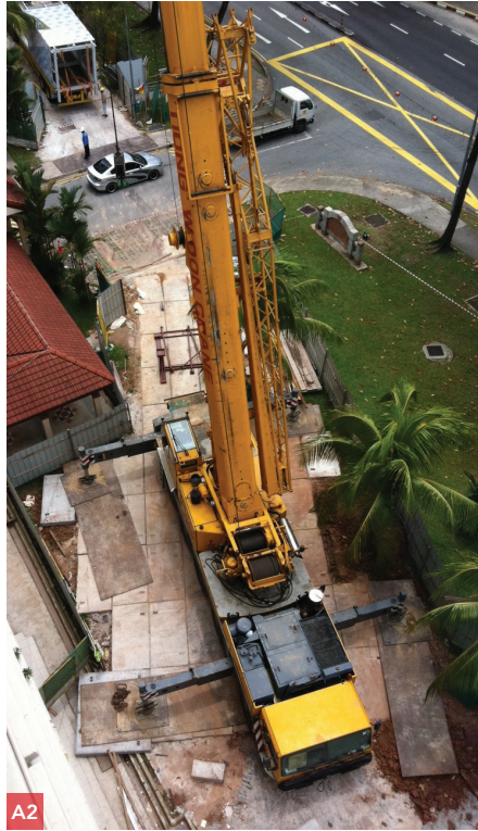
A1 & A2. Application of precast concrete panels for site access in HDB - LUP Project Photo courtesy of Teambuild Engineering & Construction Pte Ltd
