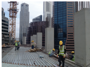
Above. Construction of CapitaGreen Photo courtesy of Takenaka Corporation
