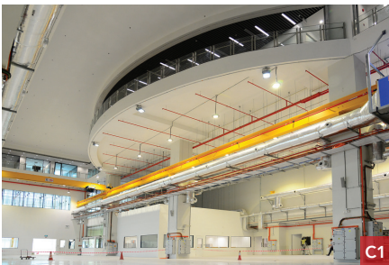
A1 & A2. Integrative Design Process B. Low energy fume hood Photo courtesy of JTC Corporation C1 & C2. ARTC Stratified cooling Photo courtesy of Advanced Remanufacturing and Technology Centre, in partnership with Nanyang Technological University
