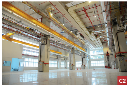
A1 & A2. Integrative Design Process B. Low energy fume hood Photo courtesy of JTC Corporation C1 & C2. ARTC Stratified cooling Photo courtesy of Advanced Remanufacturing and Technology Centre, in partnership with Nanyang Technological University
