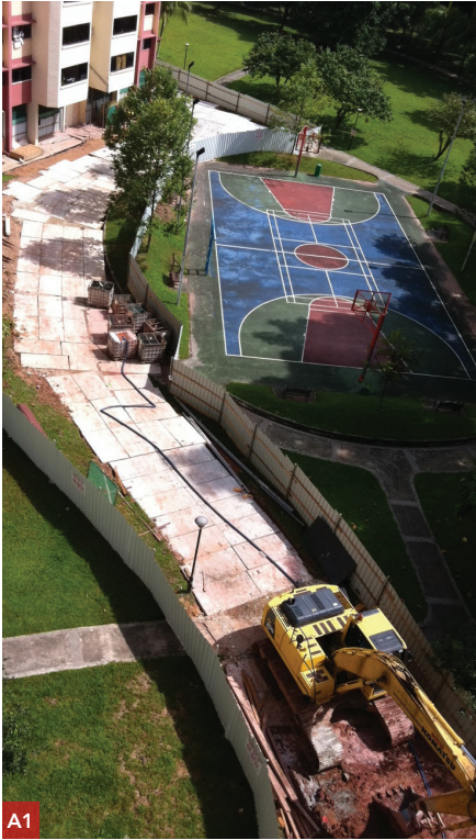
A1 & A2. Application of precast concrete panels for site access in HDB - LUP Project Photo courtesy of Teambuild Engineering & Construction Pte Ltd
