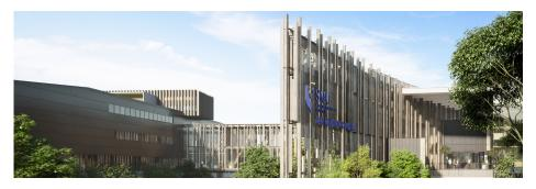
Tahir Foundation Connexion (TFC) is envisaged to be the first large-scale Mass Engineered Timber [MET] development in the city centre, as well as the first on-site Net Zero Energy Building (NZEB) with its energy demands entirely generated by the photovoltaic system located within the same building. The TFC building also boasts many green features and technologies to facilitate the attainment of Green Mark Platinum and WELL building standards.
