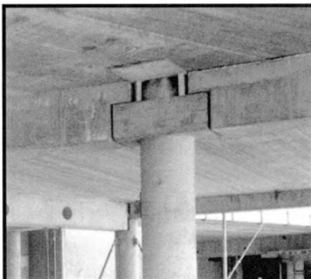
Figure 5.42 Half Joint Column/Beam Connection
