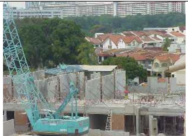
Figure 12.2 Use of 50-tonne crane for hoisting
