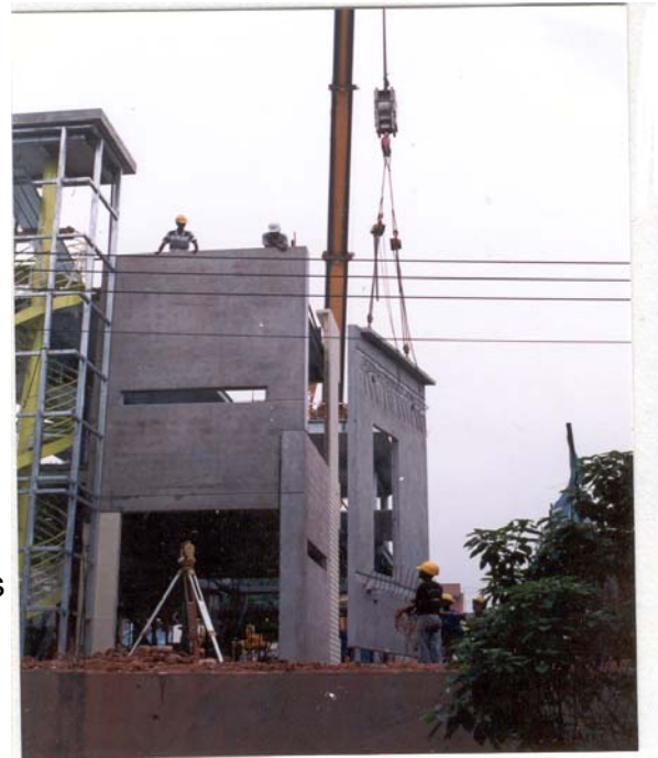
Figure 8.3 Installation of precast facade walls to beams
