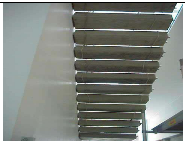
Figure 11.14 Cantilevered precast treads
