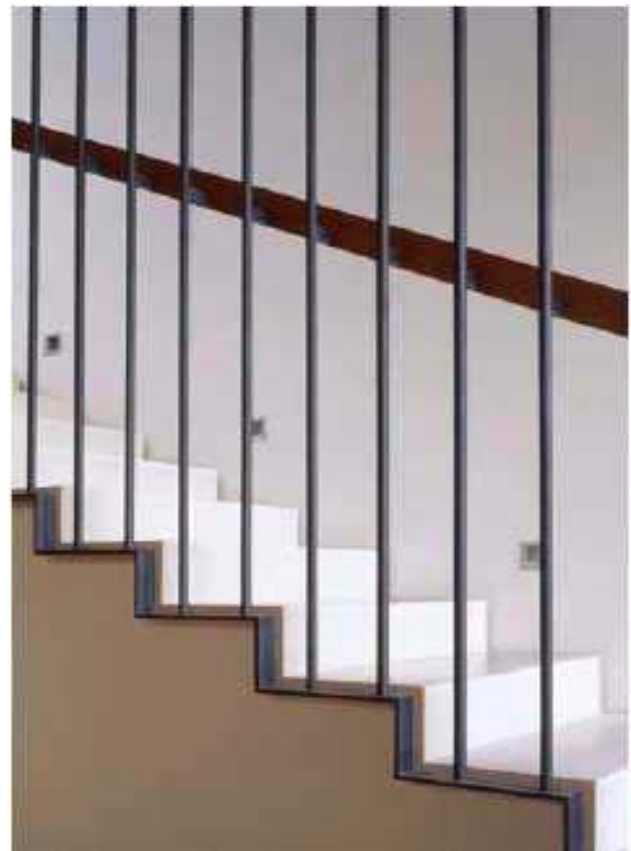
Figure 11.16 Steel stringer beams with steel treads
