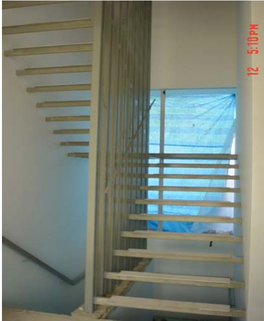
Figure 11.19 Steel plates supported on vertical steel channels
