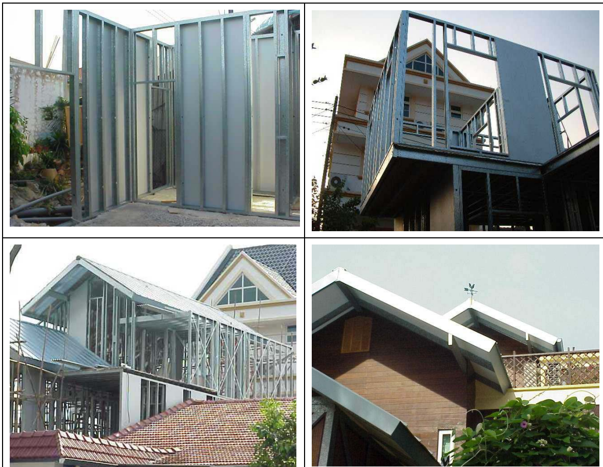
Figure 10.1 Construction of lightgauge steel frame
