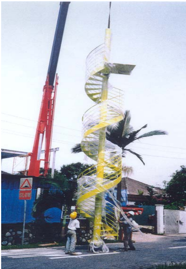
Figure 11.21 Prefabricated spiral staircase
