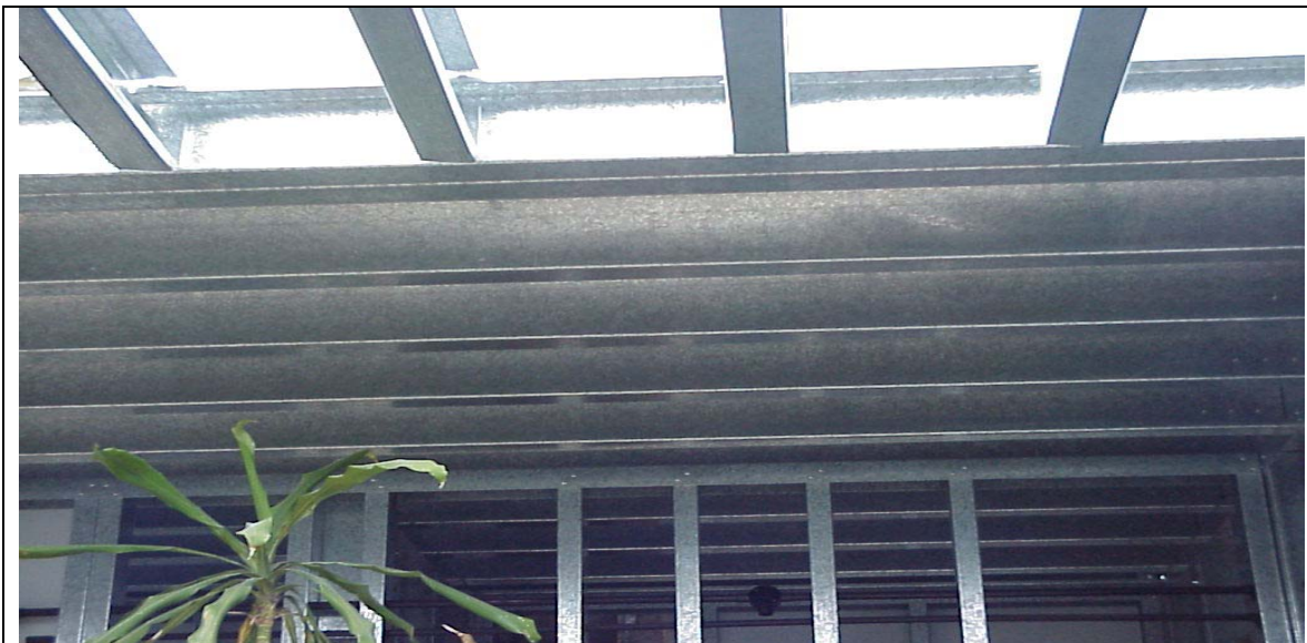
Figure 10.2 Installation of floor joist and wall studs
