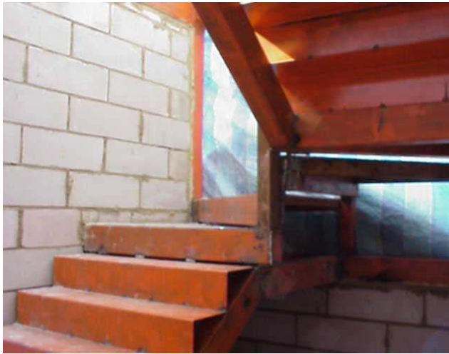
Figure 11.15 Steel plate forming treads and rises
