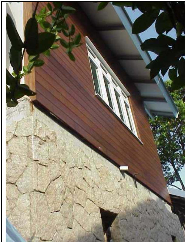
Figure 12.9 External cladding to fibre board walls
