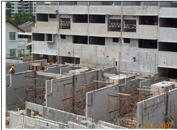
Figure 12.1 Erection of precast walls and planks
