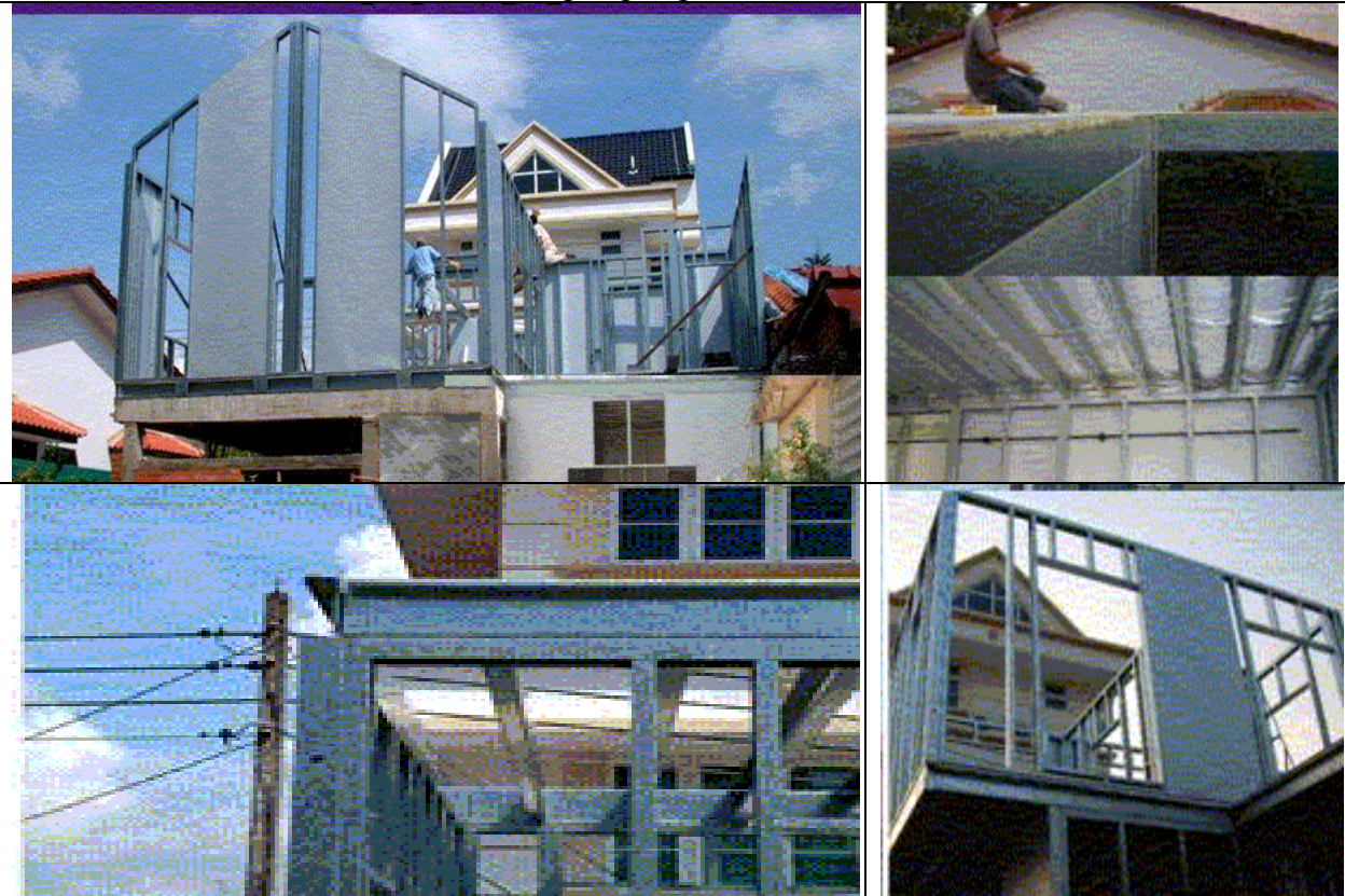
Figure 12.12 Construction of 2 nd storey
