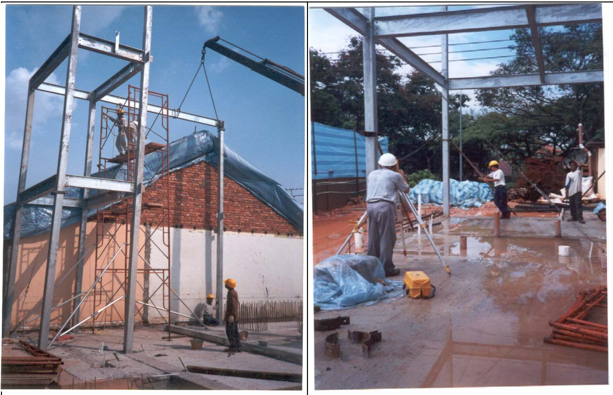
Figure 8.1 Erection of steel column and beams - Temporary bracing was required to ensure verticality of steel columns when bolt connections from beams to columns were tightened.
