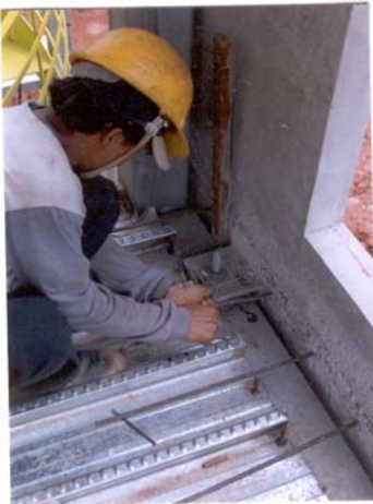
Figure 8.4 Fastening of connection
