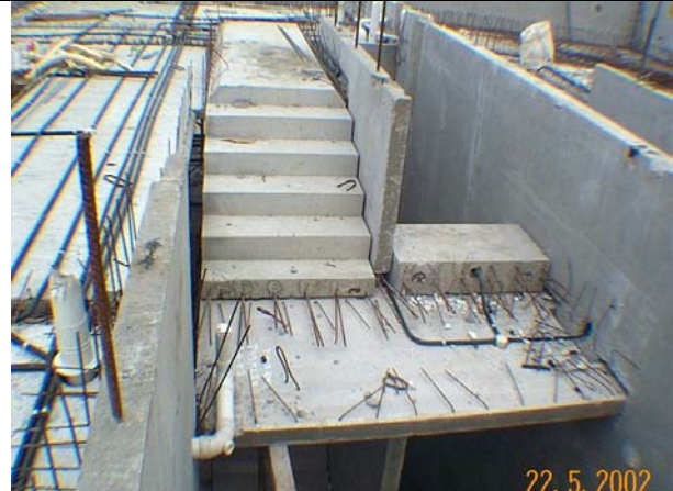
Figure 4.4 Preparation for casting of landing slab to precast staircase
