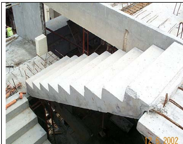
Figure 11.13 Precast Flight
