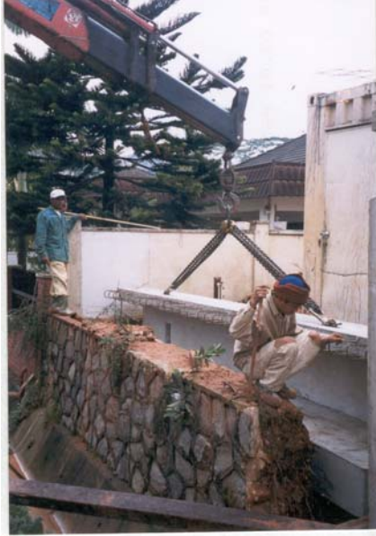
Figure 11.7 Installation of wall base
