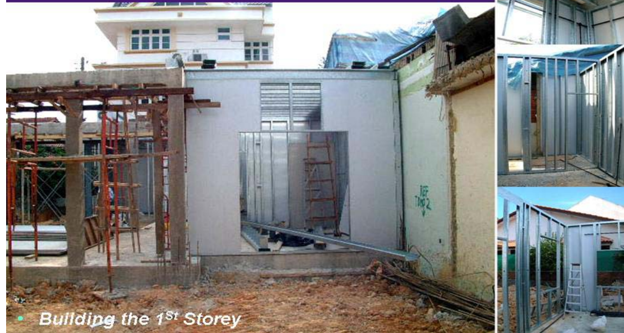
Figure 12.11 Construction of first storey. Only the front panel used CIS construction, all other areas used light gauge steel frames
