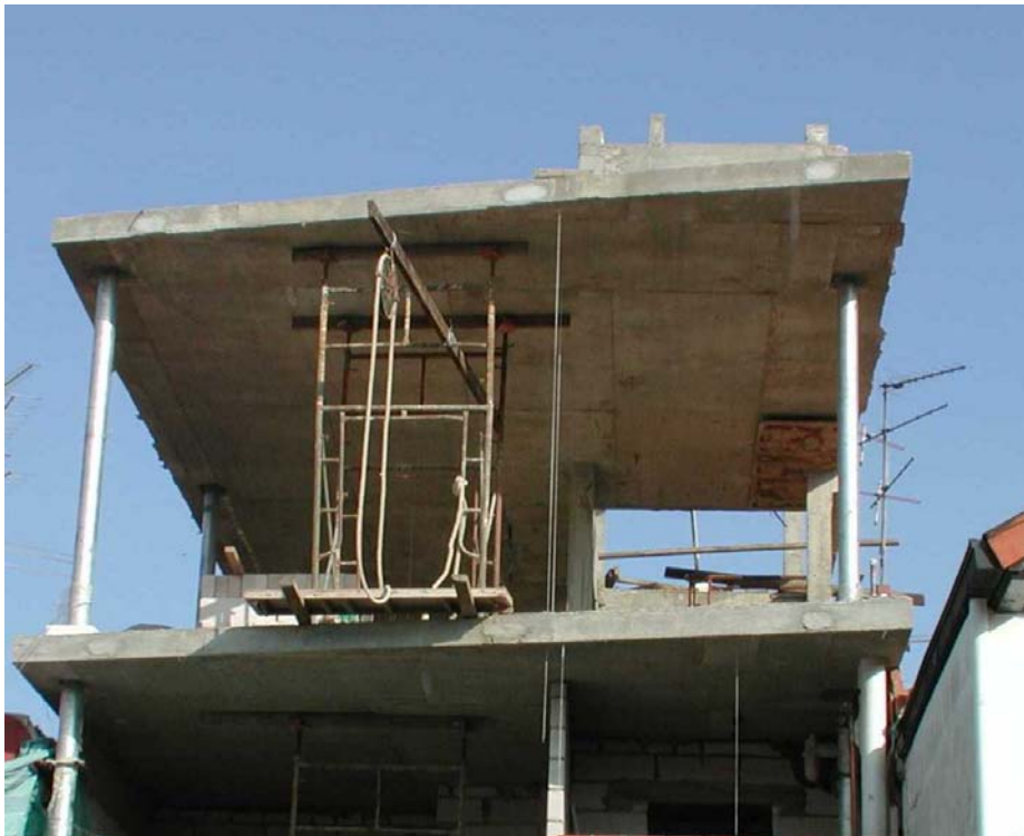
Flat plate system with circular steel column
