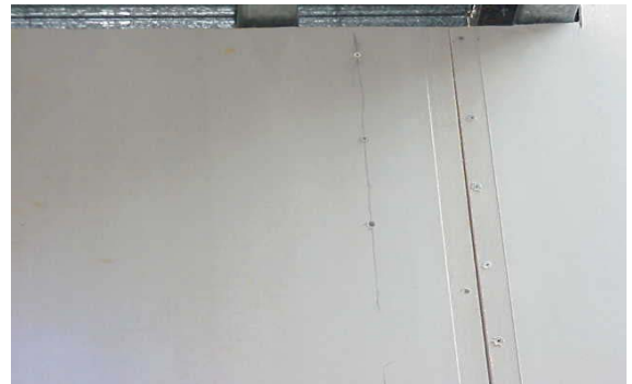
Figure 10.7 Plasterboard is screwed into position to complete the wall installation
