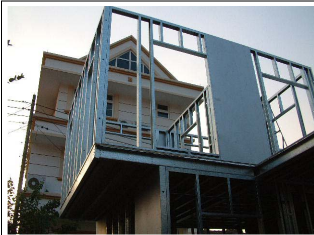
Figure 12.8 Light-gauge Steel Frame
