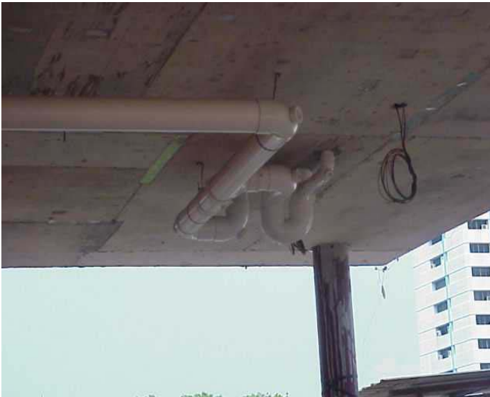
Figure 6.3 Services through slab with provision for opening
