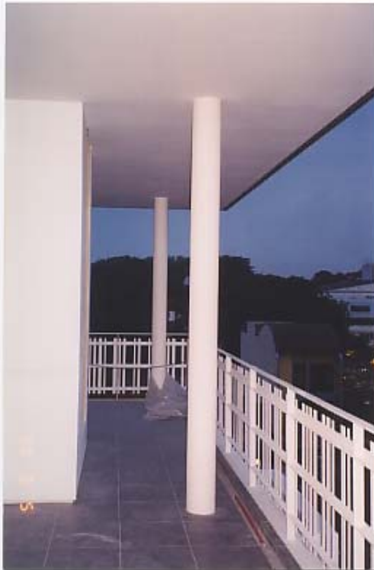
Flat plate system with circular columns
