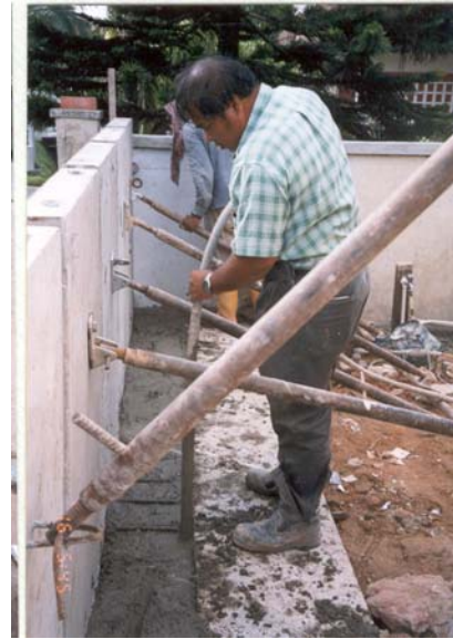
Figure 11.8 Precast walls are placed and propped
