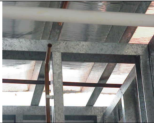
Services can be suspended from steel frames
