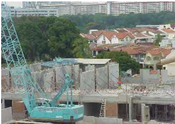
Figure 2.1 Use of 50-tonne crane for hoisting
