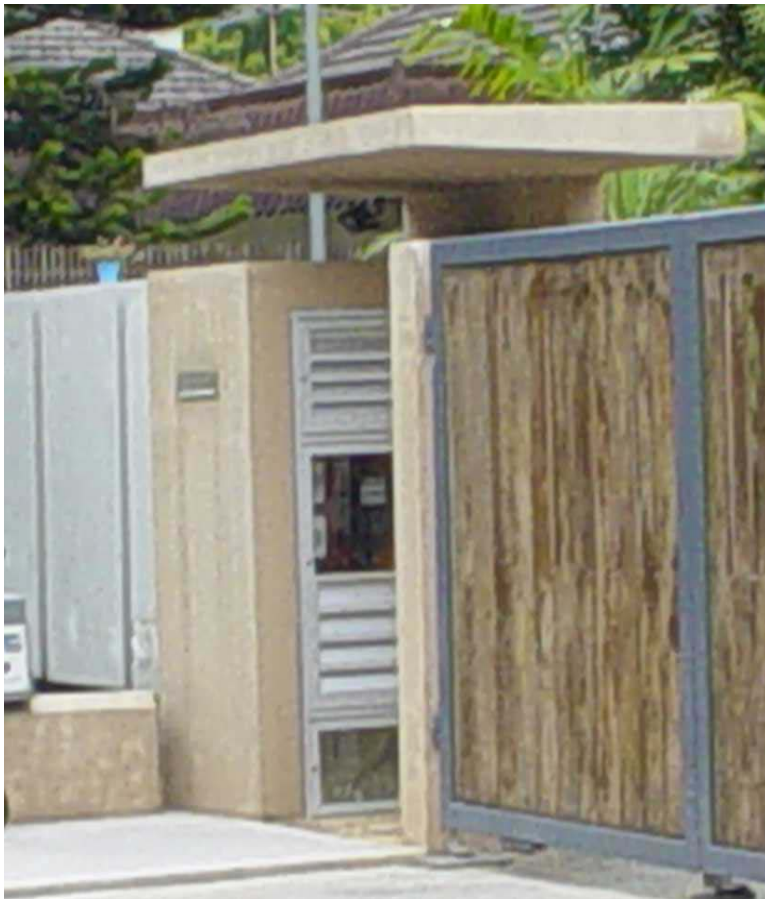
Completed precast meter chamber
