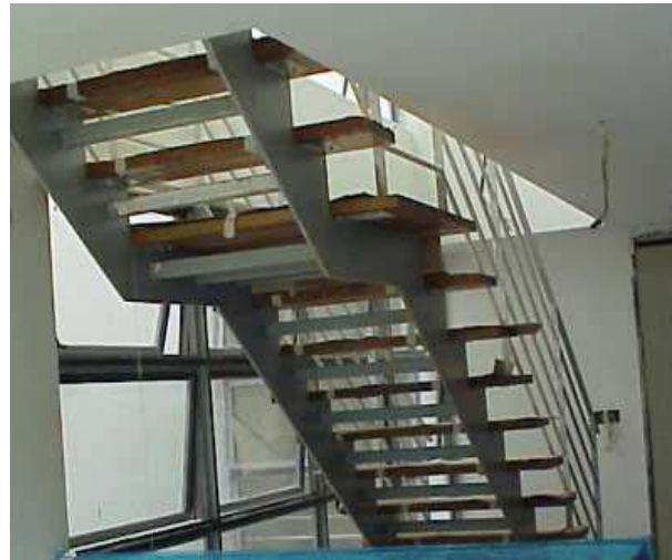
Figure 11.16 Steel stringer beams with steel treads
