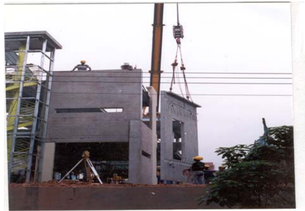
Figure 2.2 Hoisting of precast facade
