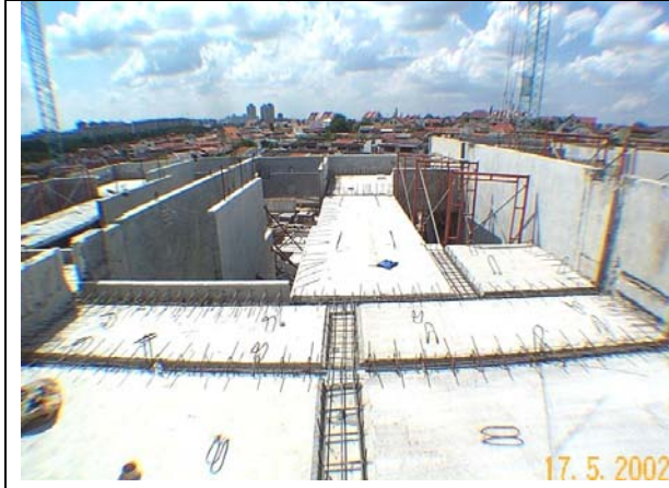
Figure 4.1 Precast walls are propped before casting of joints – proper planning is required for perfect alignment
