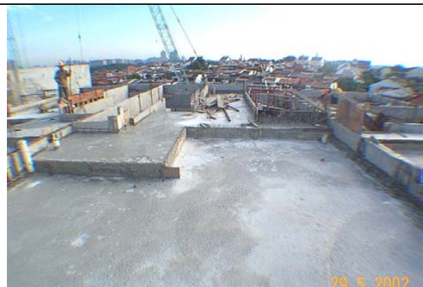
Figure 4.6 Concreting to topping
