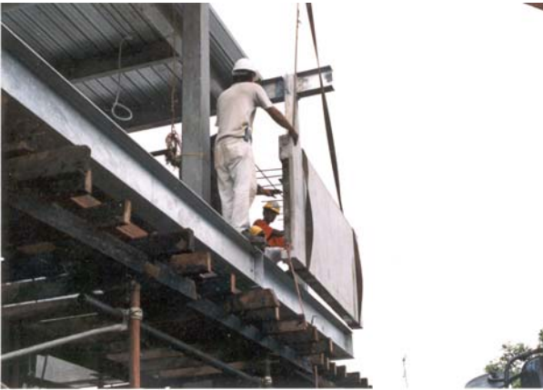
Figure 8.3 Installation of precast facade walls to beams
