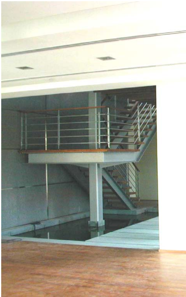
Figure 11.17 Steel plates supported by centre column
