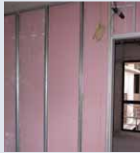
Install plasterboard to one side
