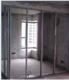
Install metal studs
