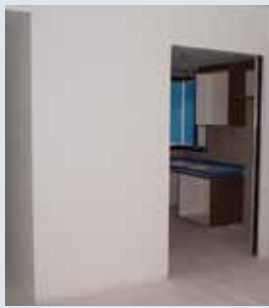
Apply paint and install fixtures to walls
