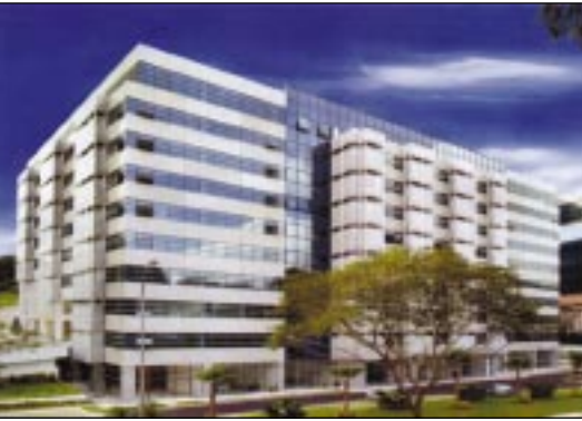
E-Centre @ Redhill features a predominantly precast structure, walls and other components.
