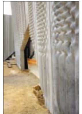
Deep profiled pattern on the exposed face of precast wall Images courtesy of : Photocall Australia
