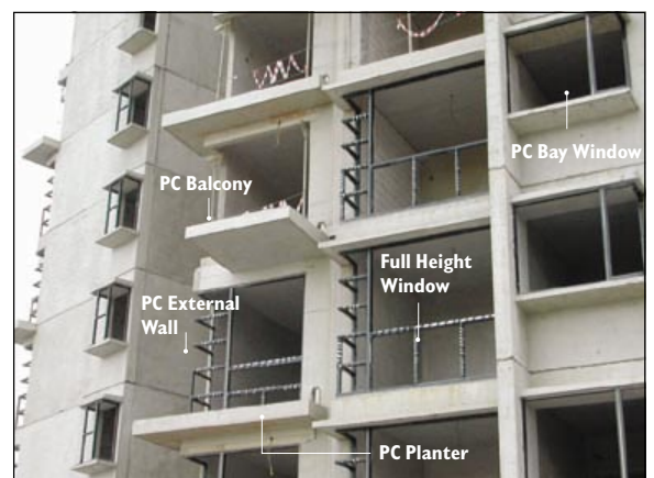
Park Green at Sengkang (above and below) features dual objectives - a contemporary clean-cut design as well as high buildability (below)
