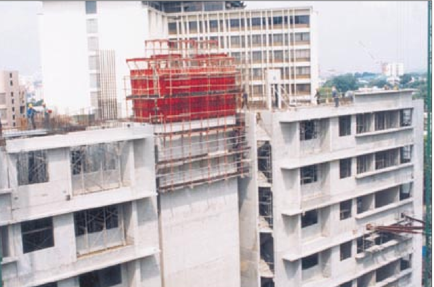
Installation in progress - precast facade, plank and household shelter
