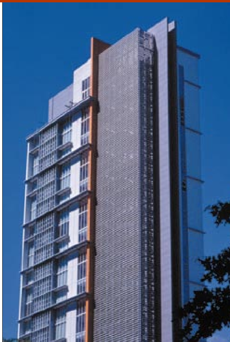
Expression of planes at roof level and wrapping of main staircase in aluminium screen
