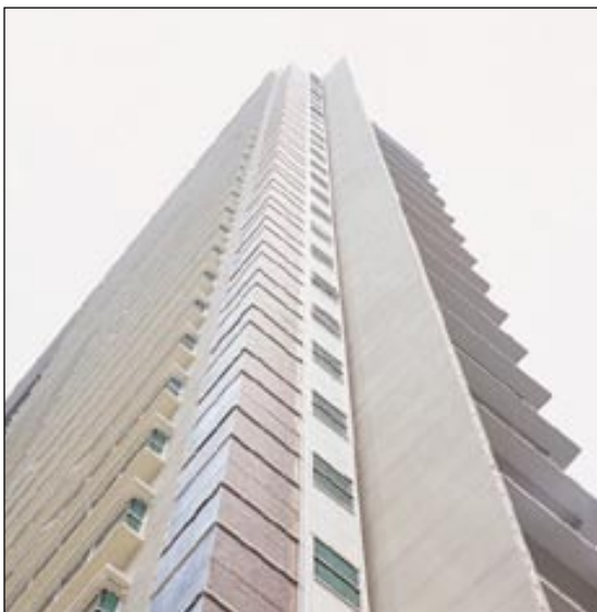
Achieving flatness of the wall through precast wall system
