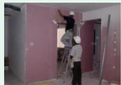
Installation of the Boral Impact Panel system at the Savannah CondoPark
