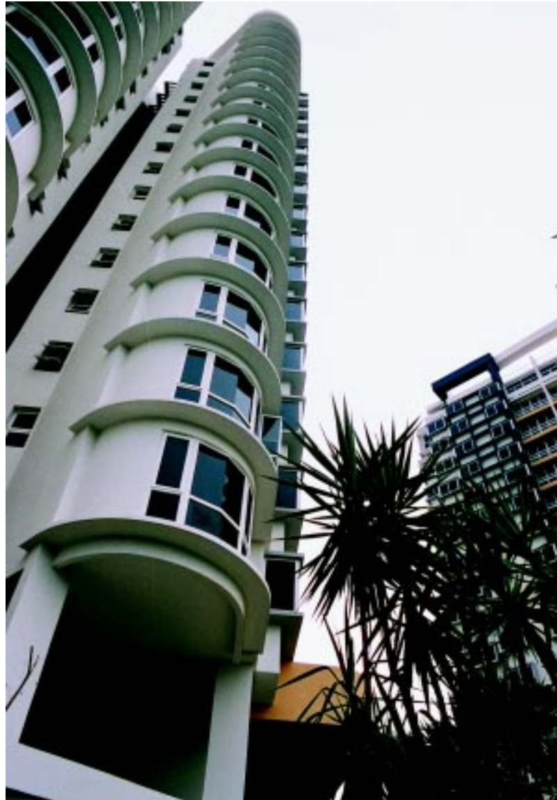
Close-up of precast curved facade
