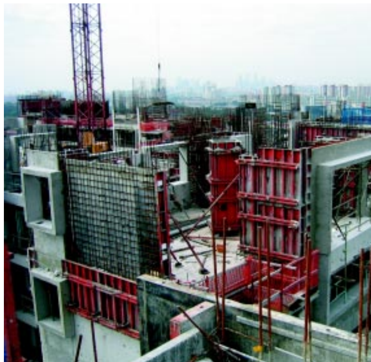
Integration of precast and cast in-situ construction
