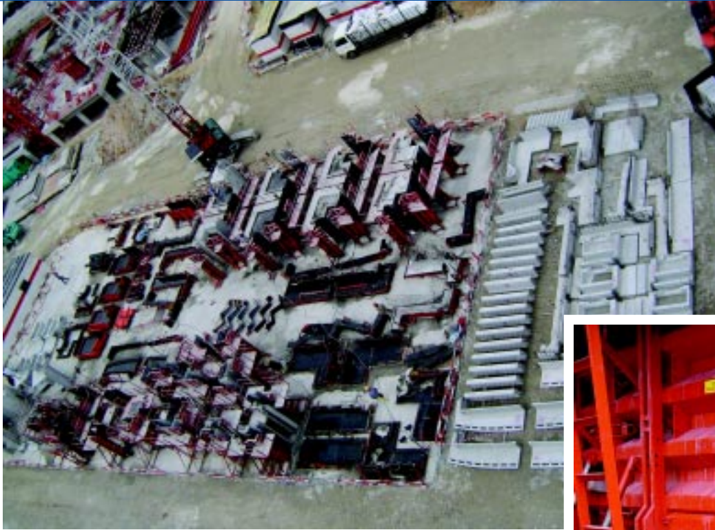
Site precasting in a factory-like setting at the Savannah CondoPark
