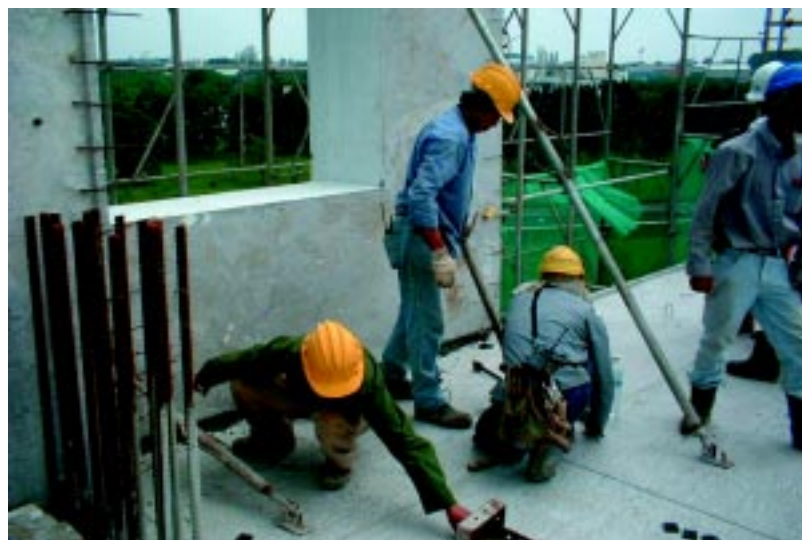
Propping of precast facade
