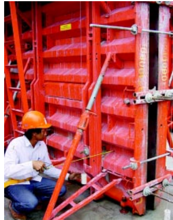
The distinctly coloured system formwork used by Dragages
