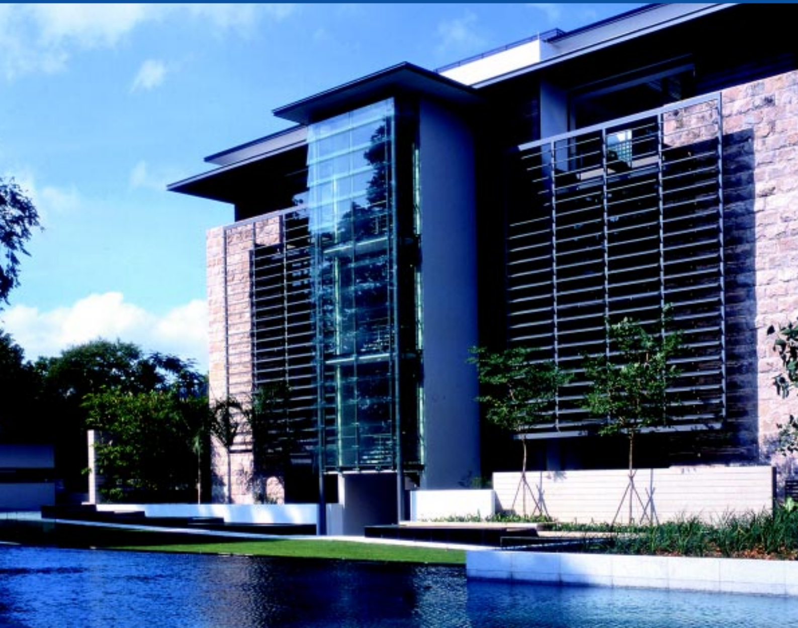
Precast beam, sunshade, parapet and A/C ledge are some of the precast components used at The LadyHill
