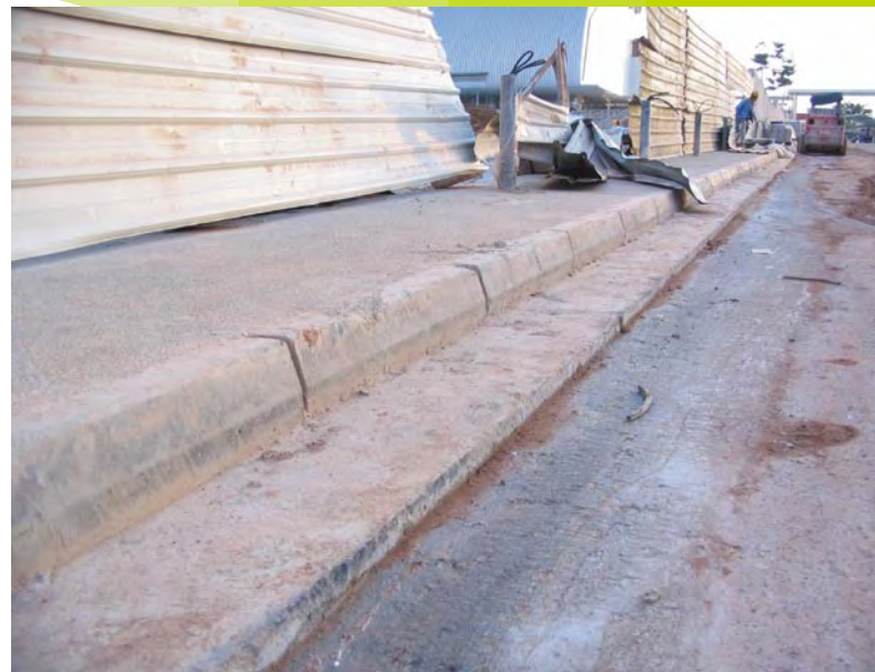
Installation of recycled road kerbs leading to the Sports Hall
