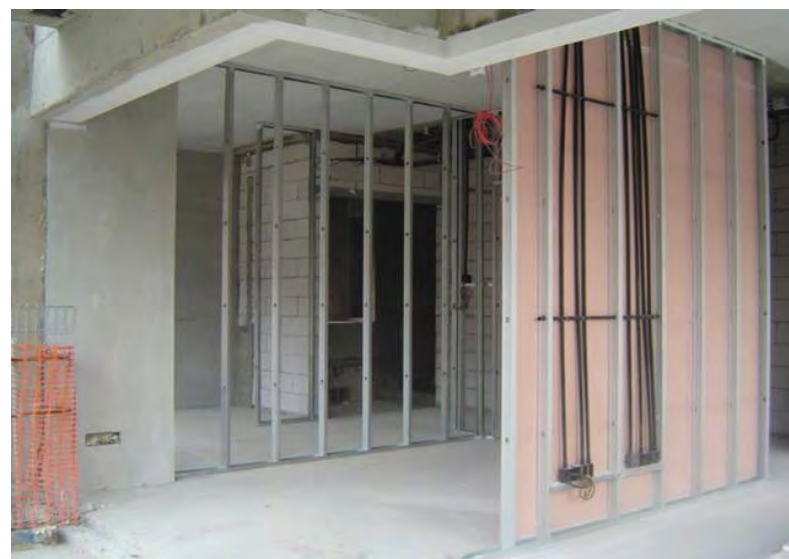
Installation of drywall partitions in living room & bedroom
