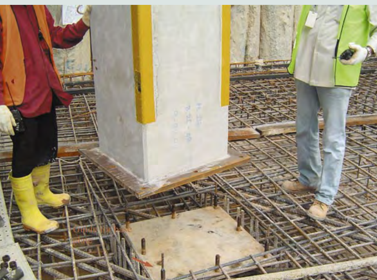
Guiding precast column into position
