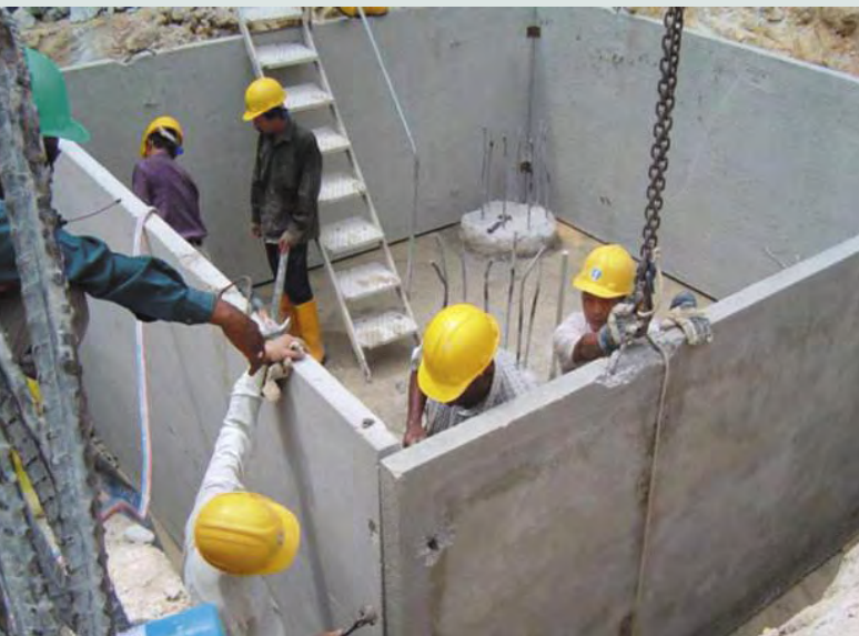
Installation of precast formwork for pile cap
