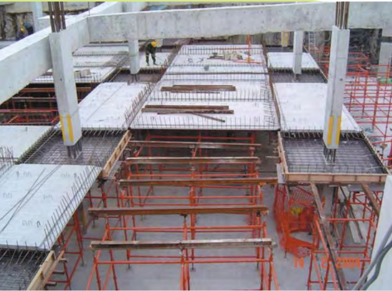
Using precast planks to form flat slab
