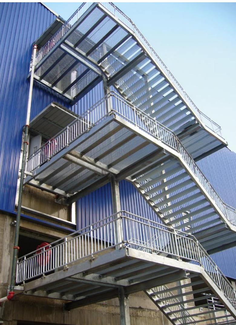
Prefabricated steel staircase and handrail for external emergency escape staircase
