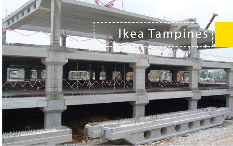
**Extensive use of precast structural components**
