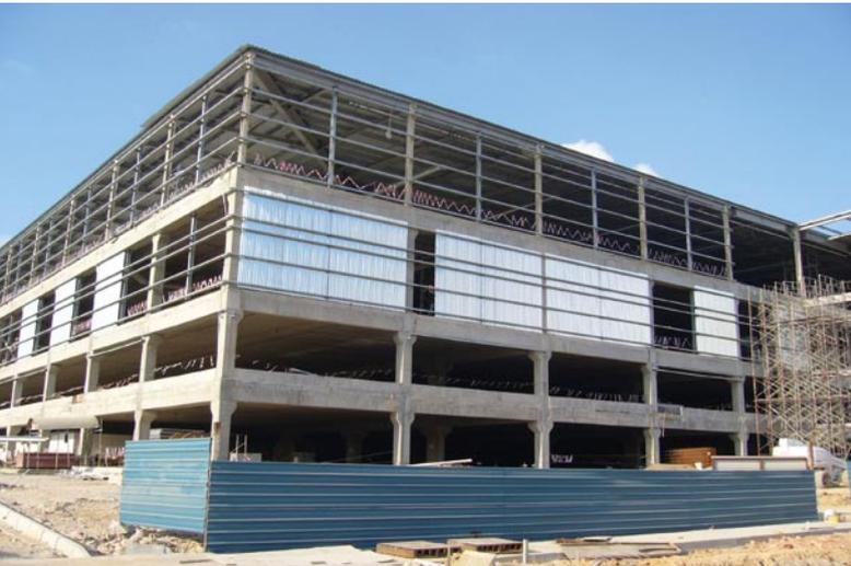
**Precast and prefabricated steel column/girder system**
