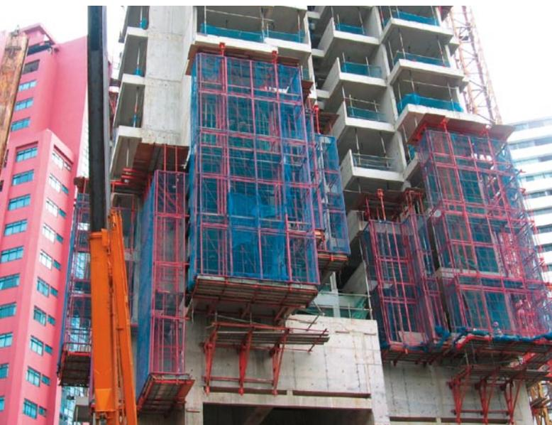
**An in-house multi-tiered hanging cage was used for all the external architectural works to free the ground level for access.**
