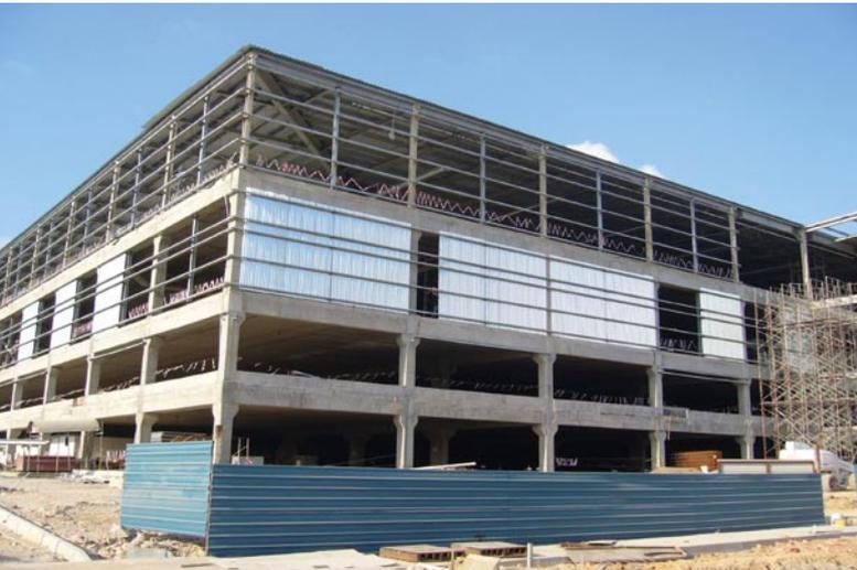
**Precast and prefabricated steel column/girder system**
