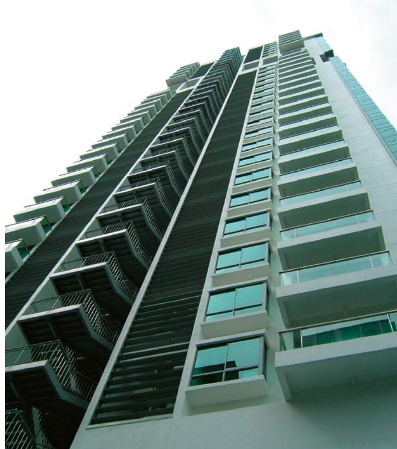
**The use of steel for the external staircase allowed for the off-site assembly of its components and a better control of its finish and overall quality**
