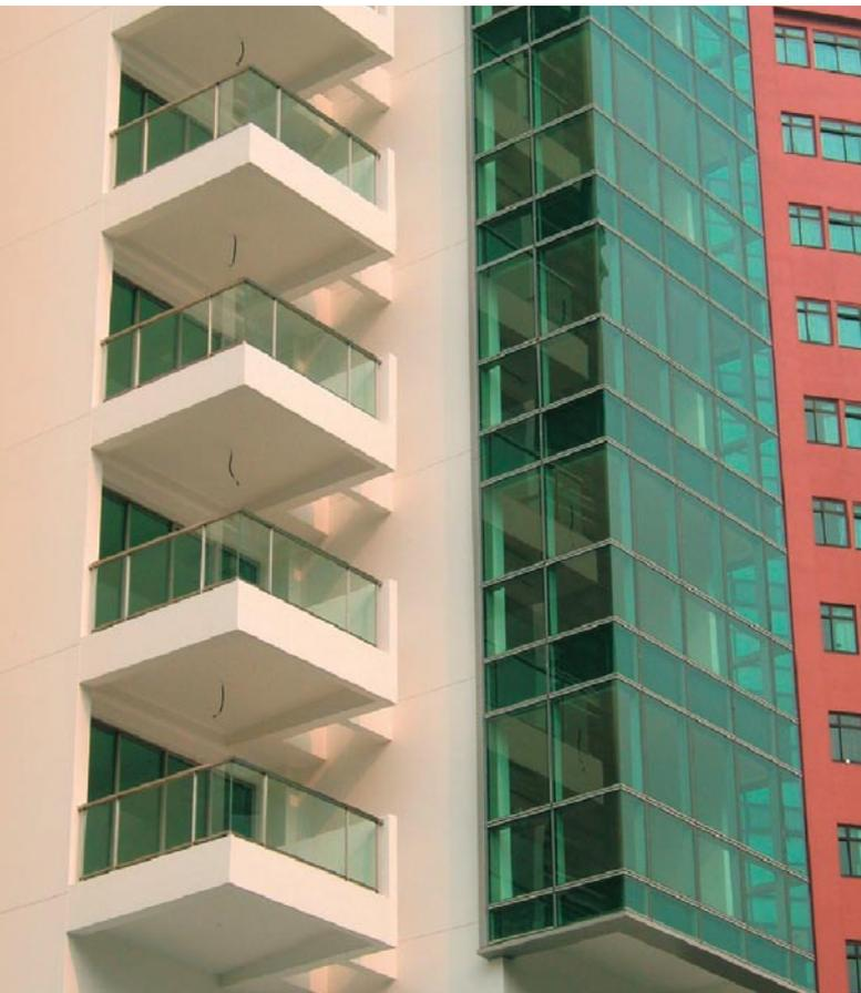
**Laminated tempered glass railing with stainless steel framing were extensively used in balconies and planter boxes**
