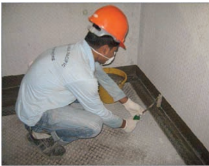
3. Laying of waterproofing system to floor and wall
