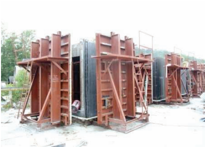
1. Casting of concrete shell
