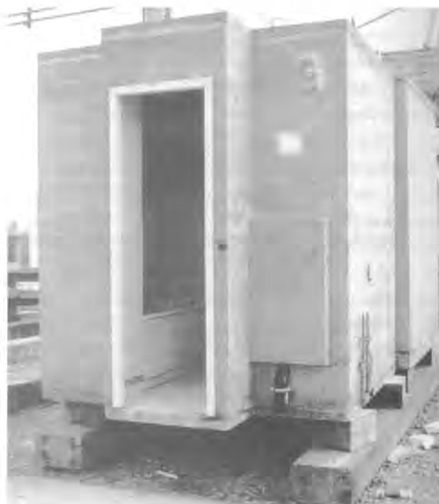
Figure 1 : Precast Concrete Cell with Finished Floor and Walls.
