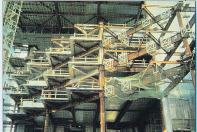
Column to Beam Connections
