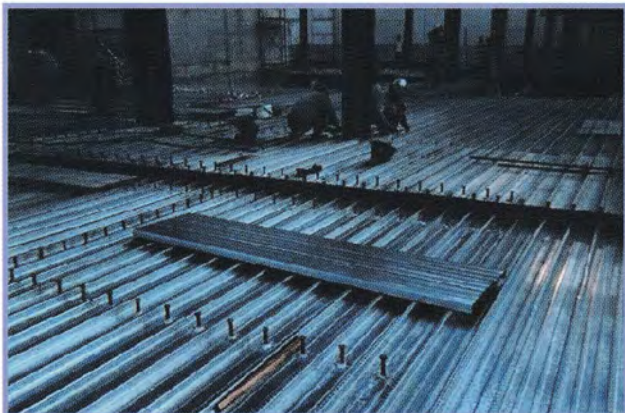
Shear Studs Welding on Metal Decking and Top of Steel Beam
