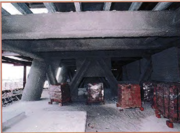
Inclined Column and Outrigger Trusses at the Mezzanine Fl.
