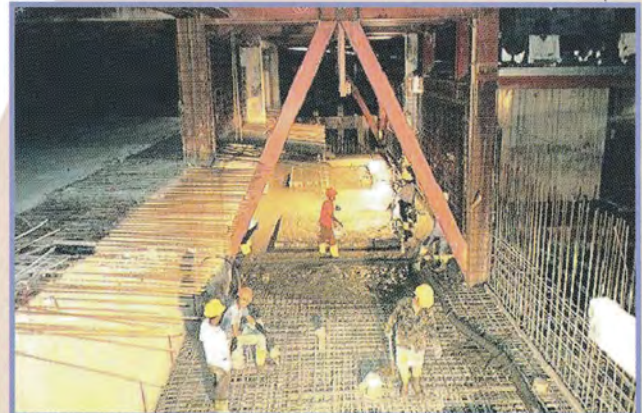
Inverted K-Frame and Casting of Floor Slab
