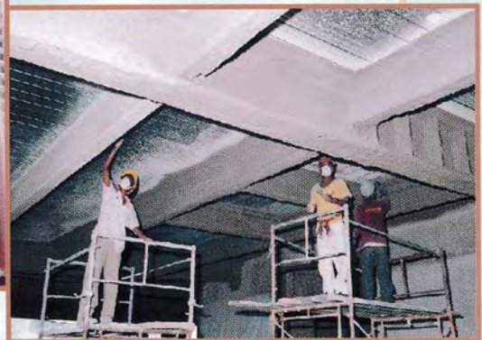
Cleaning of metal deck after Fire Spray at 23 rd Fl.
