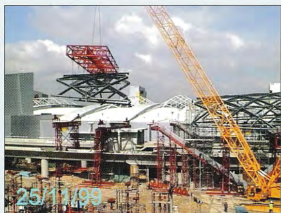
Lifting of Assembled Module
