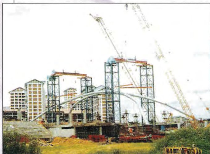
Erection of Arch Roof
