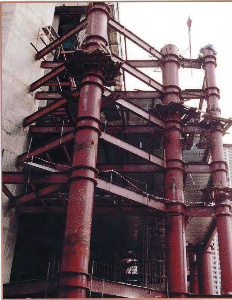
Steel Tube Column Erection with Connecting Beam at Cecil St. Side.
