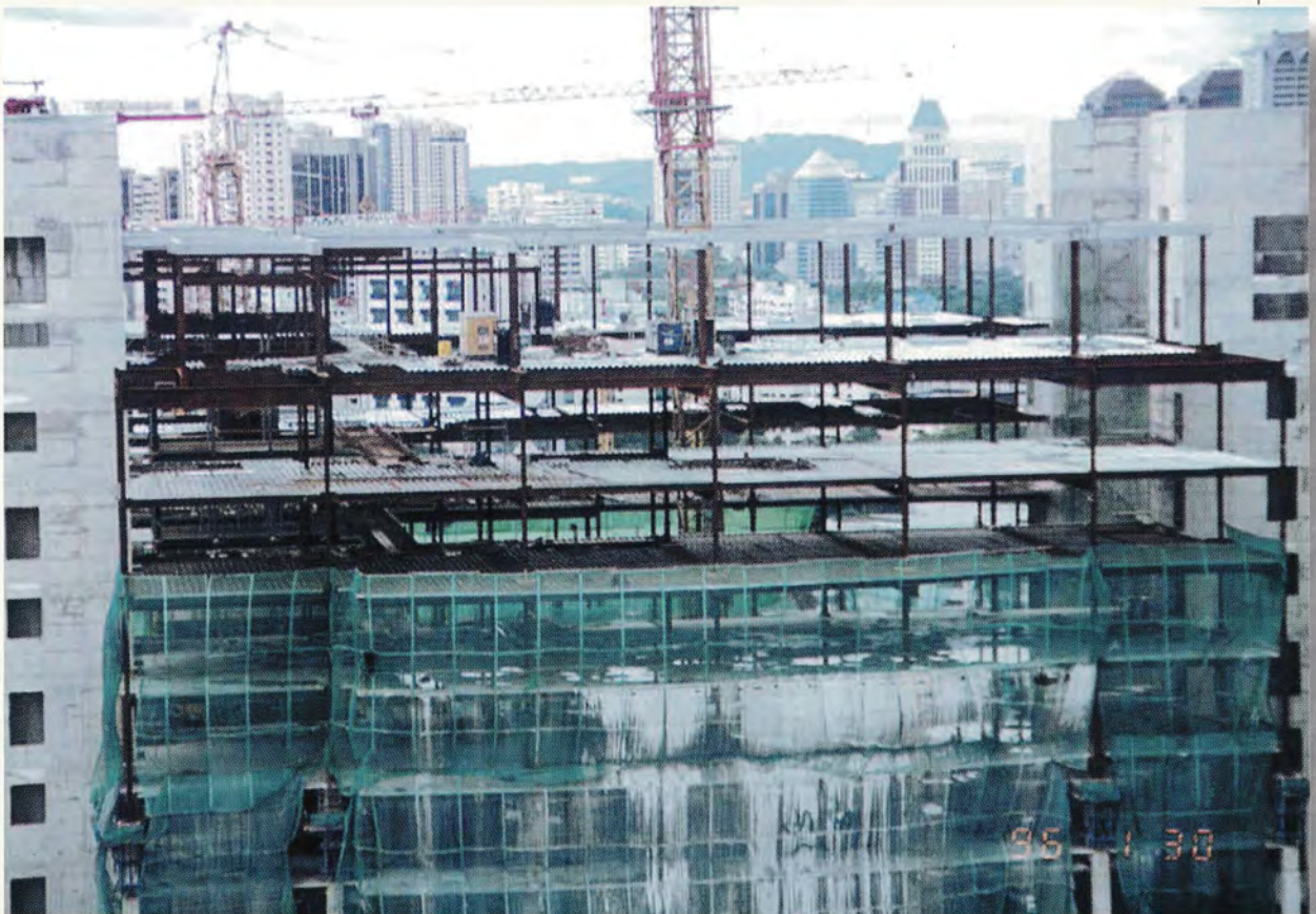
Composite construction with steel decking used as permanent formwork.
