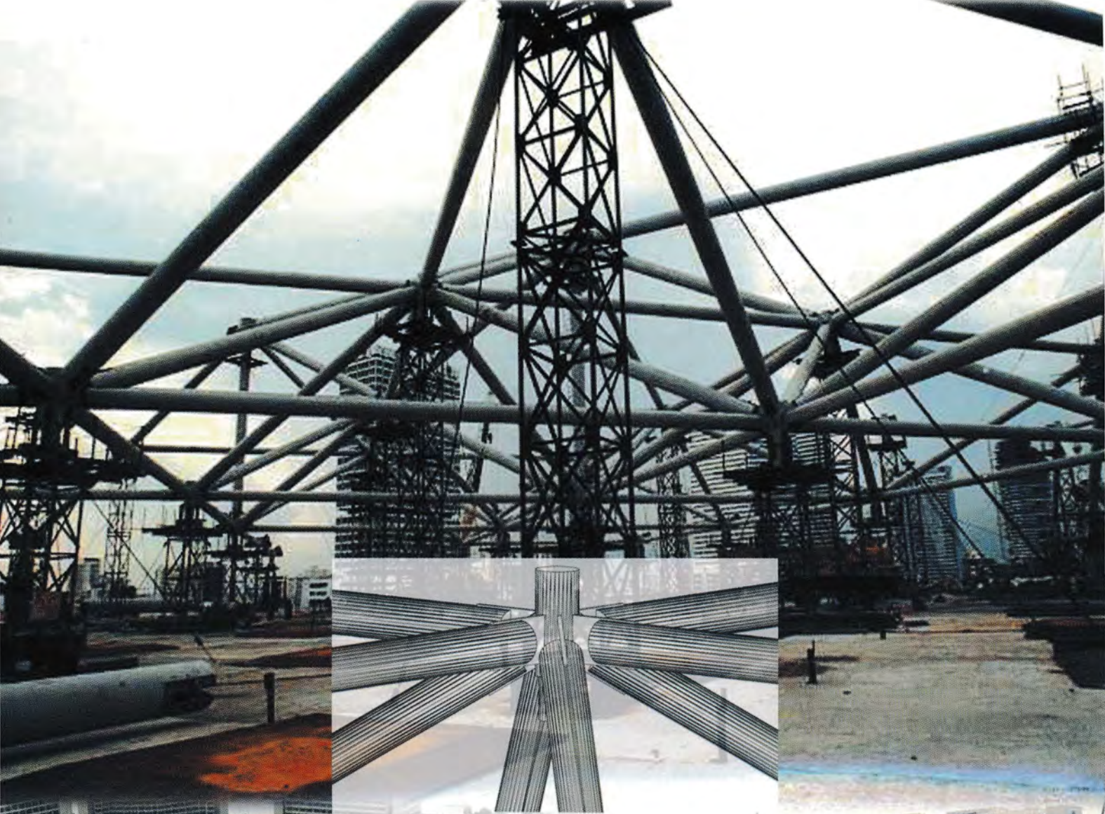
Tubular Members Connecting to a Node
