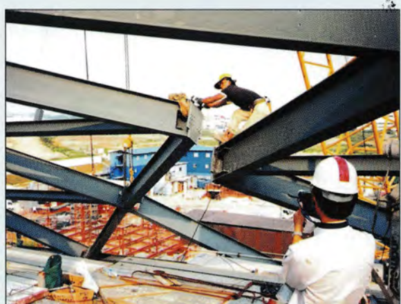
Bolting at Module connections
