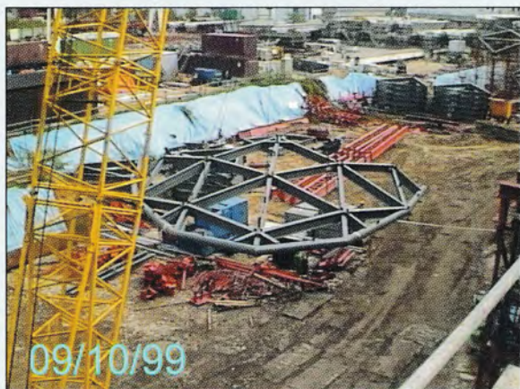
Fabricated Diagrids
