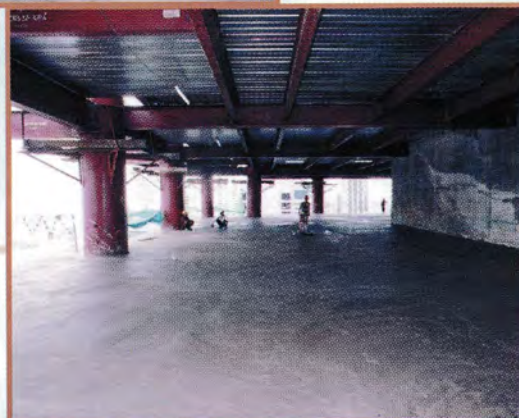
Power coating Finish on Surface of Concrete.
