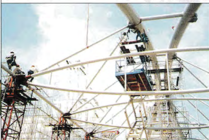
Lifting of Sports Hall in Progress
