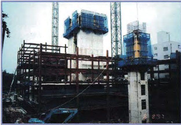
Steel Framework with Core Walls
