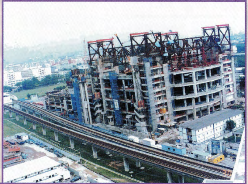
Assembling of the sport hall structure on the roof top
