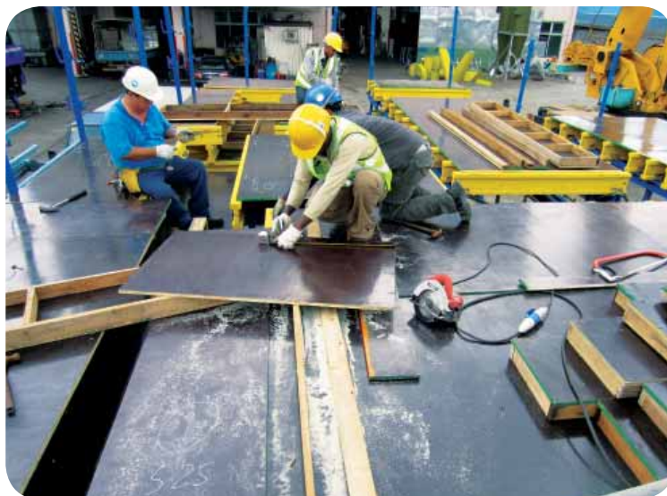
Placing of infill panel
