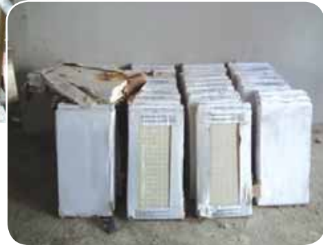
Placing of tiling materials near working area
