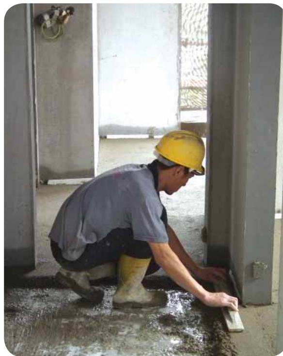
Finishing screed with wooden float
