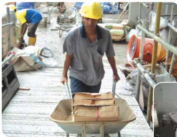
Transporting tiling materials to working area
