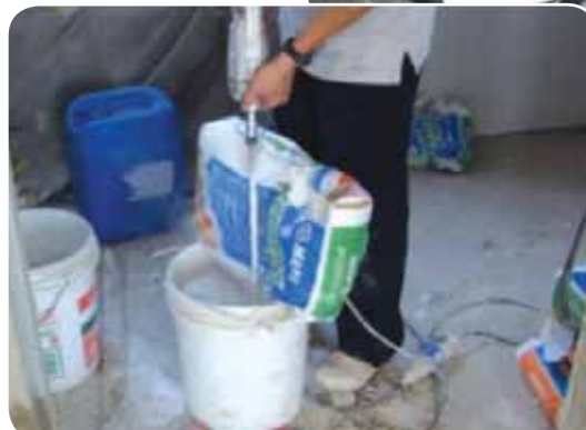
Mixing the tiling adhesive in accordance to the manufacturer's instruction menu
