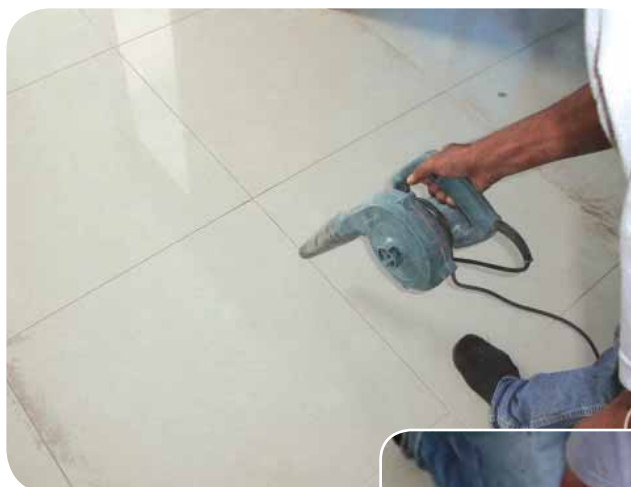
Removing of dust trapped between tile joint
