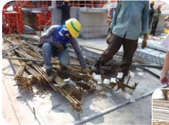
..... Sorting of re-bars to ensure the correct size and quantity are in order
