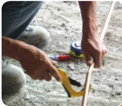
Cutting of water pipe to required length
