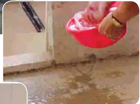
..... Damping screed surface to reduce suction.
