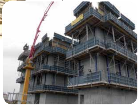
Concrete Placing boom
