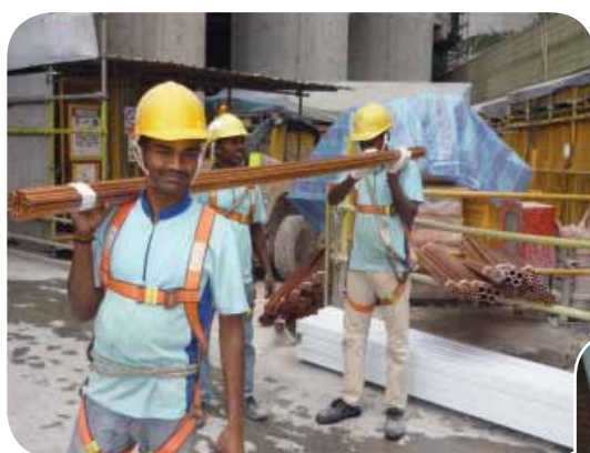
Transporting piping materials to working area
