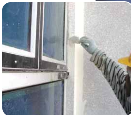
Painting to edges using brush
