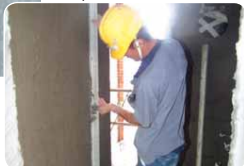
Plastering of wall for even and rough surface to receive the tiles.
