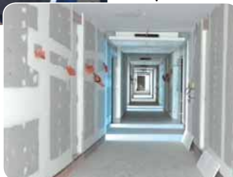
Completion of drywall
