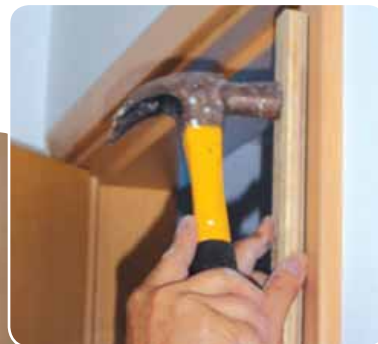
..... Installing the architrave around door frame (if any)
