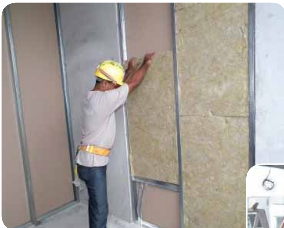
Installing insulation between panel (M&E work is excluded from the drywall trade.)
