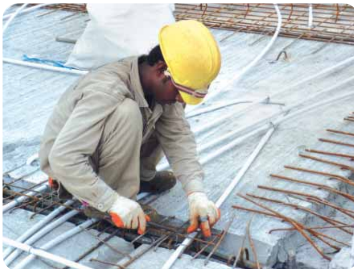
..... ..... Securing of conduits to re-bars
