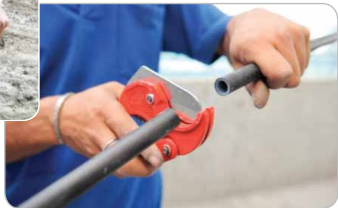
Cutting of PEX pipe
