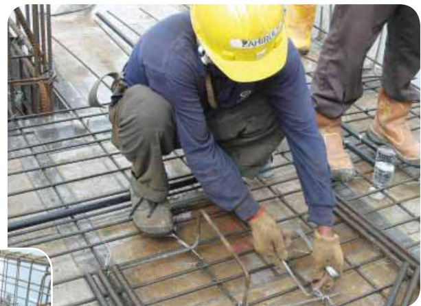
..... Fixing of re-bars using hand tool
