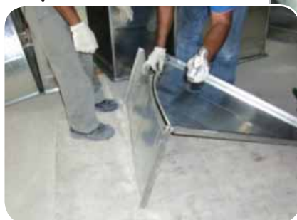
Marking and cutting of ductwork to shape
