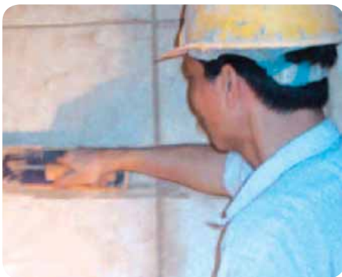
..... Spreading grout with a soft trowel
