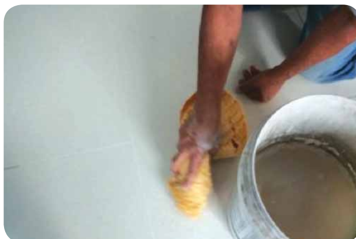
Cleaning of tile to remove stain or other residue
