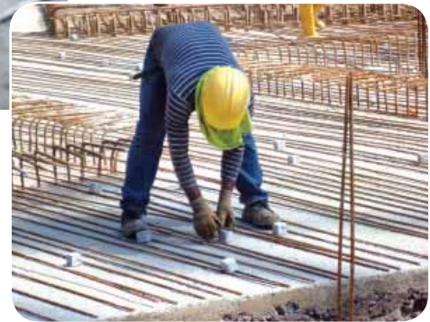
..... Placing of concrete spacer
