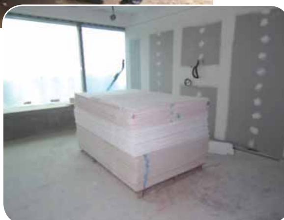
..... Placing of ceiling materials at working area
