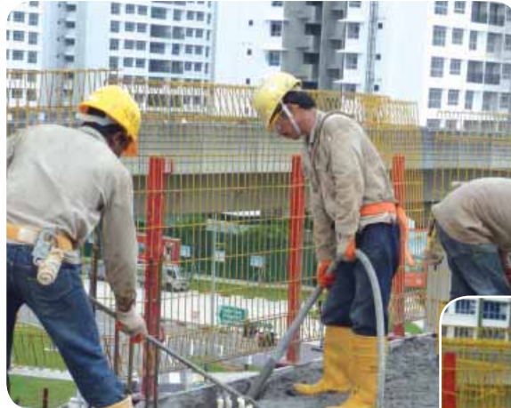
Spreading of concrete with shovels
