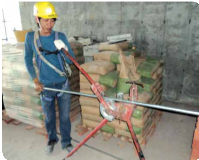
..... Bending of electrical conduit in-progress
