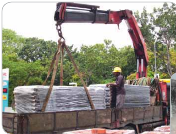
Transporting door materials to working area
