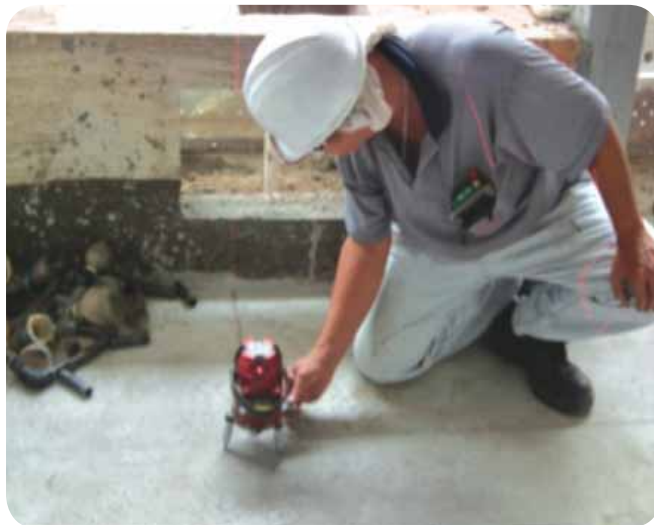
Setting out tile lines on screed
