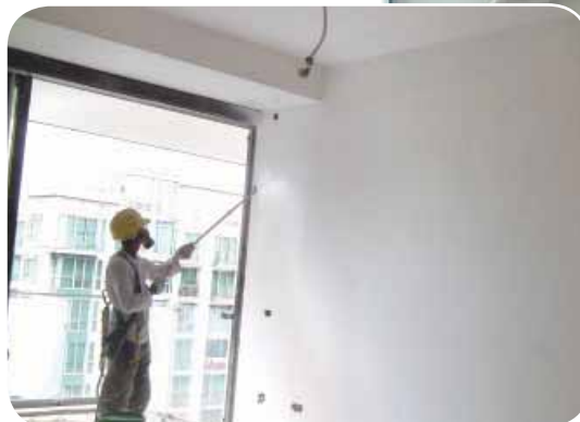
..... Application of sealer coat by spray
