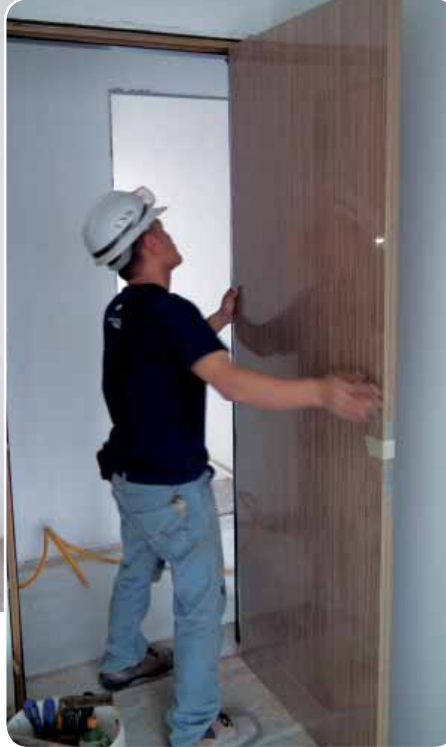
..... Installing of door panel
