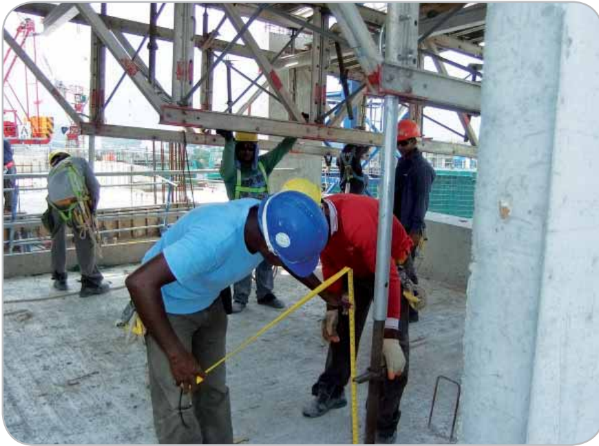
Checking and adjusting the level of the table formwork
