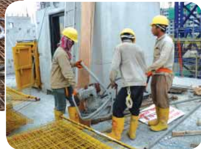
Preparation of concreting equipments and tools
