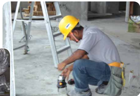
Setting out the position of the drywall at floor level
