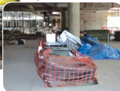
Placing of ducting materials near working area
