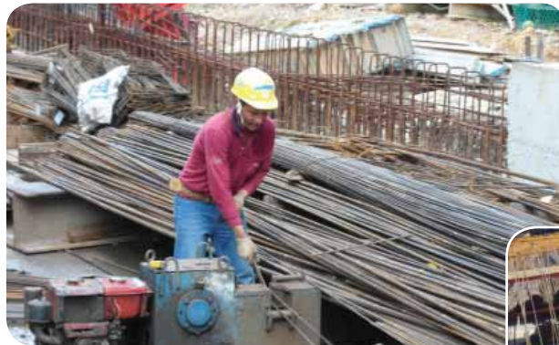
..... Cutting of re-bars to required length
