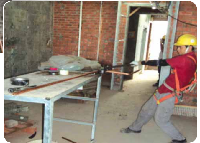
Bending of water pipe
