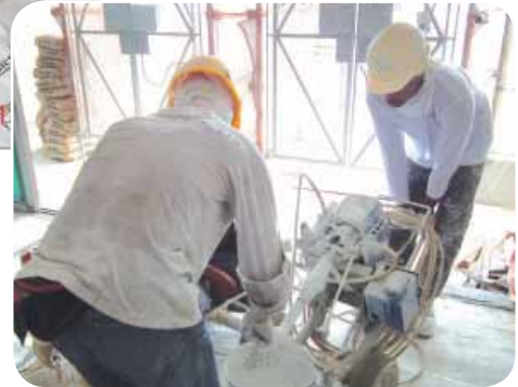
..... Setting up of spray painting equipment
