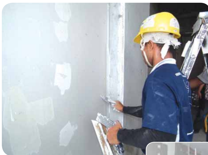
Sealing up the joint between plasterboard (Painting of wall is excluded from the drywall trade.)
