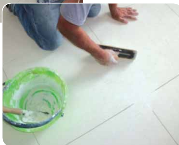
Pointing of joint between tile with colour grout
