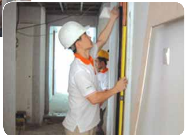
..... Installing of sub-frame
