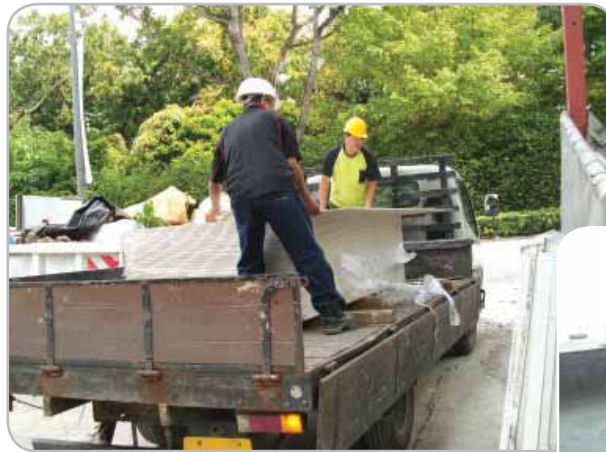
Transporting drywall materials to working area
