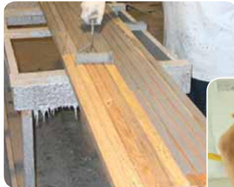
..... Treating surface of sub-frame
