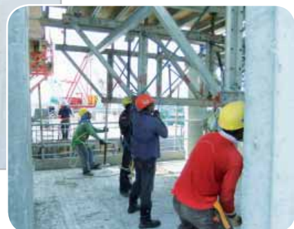
..... Positioning the table formwork
