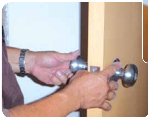
..... Installing ironmongery to the door panel
