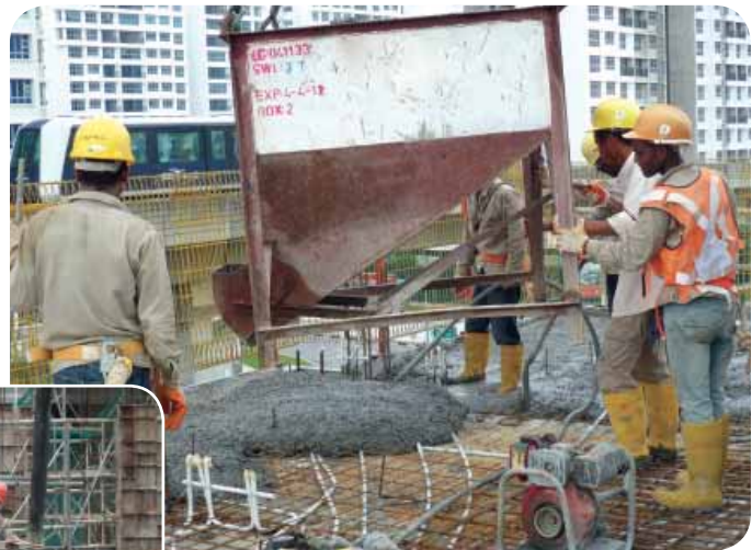
Placing of concrete using concreting bucket
