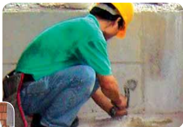
Setting out reference line in relation to wall alignment.
