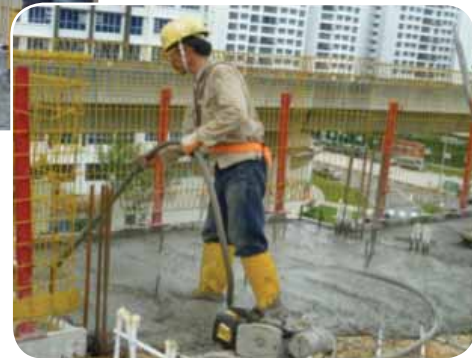
Compacting of concrete with a vibrator
