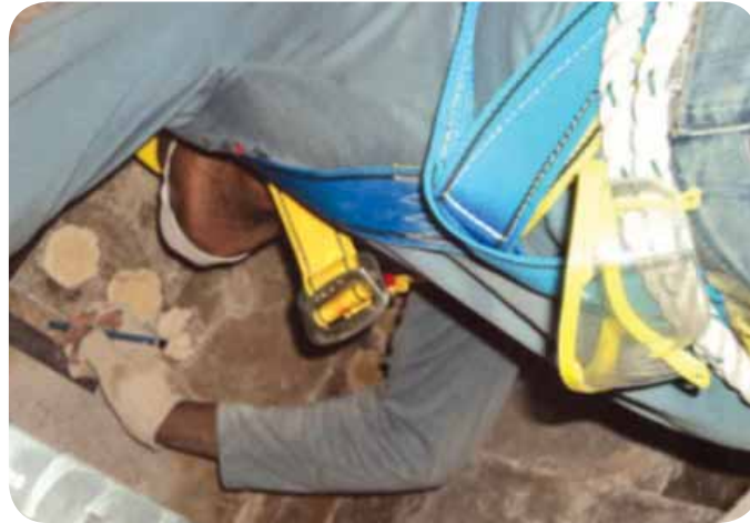
..... Marking of pipe routing
