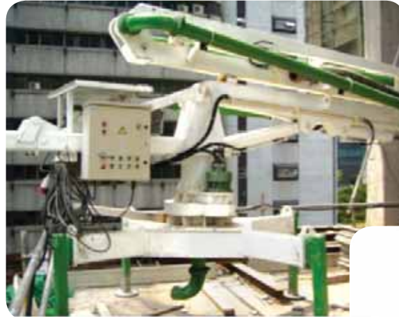
Rotary distributor for concreting work
