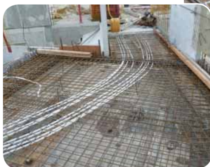
..... ..... Fixing of top reinforcements ..... and securing of conduits ..... to ensure they are firmly in ..... position before concreting
