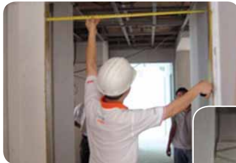
..... Verify the dimensions of the sub-frame opening
