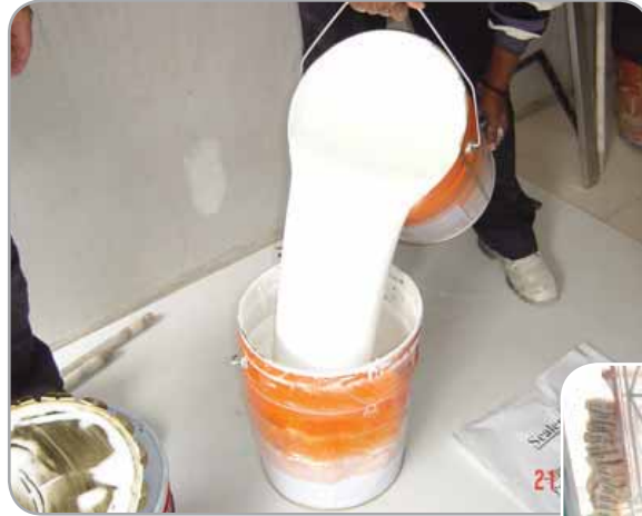
..... Mixing of paint manually
