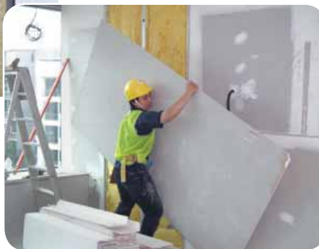
Installing second plasterboard
