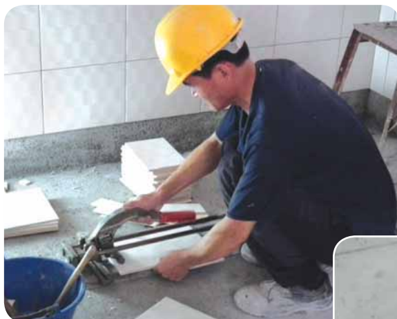
..... Cutting of tiles to required size
