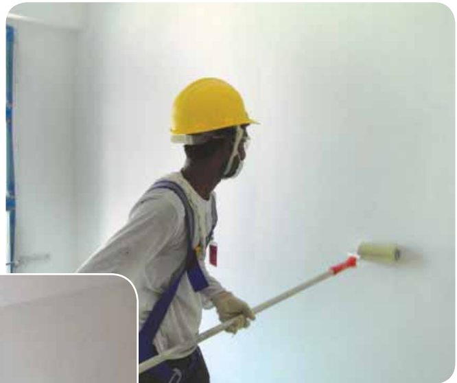
..... Application of sealer coat by roller
