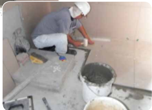
..... Tapping tile onto uniform position using a rubber mallet.
