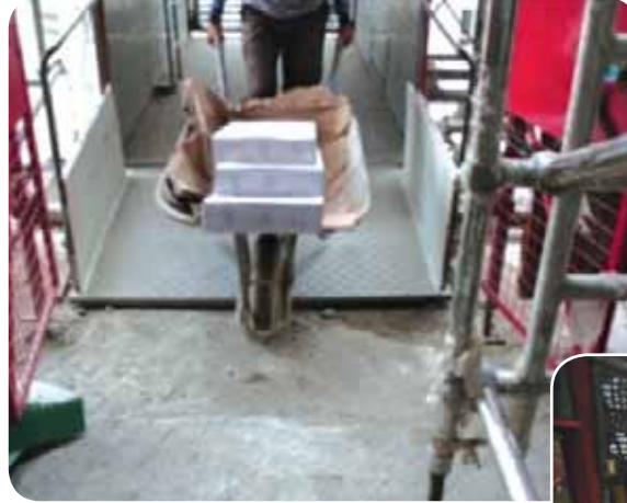
Transporting tiling material using wheel-barrow
