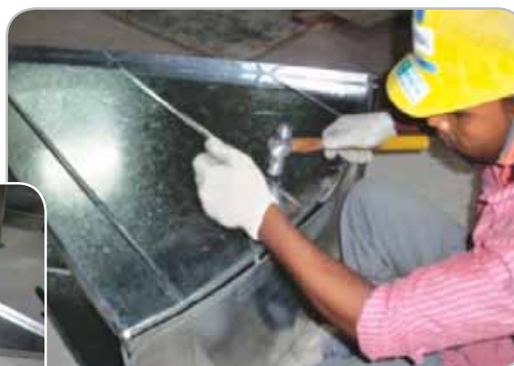
Bending and forming of ductwork section together
