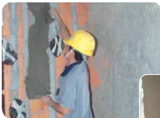
Patching up all concealed conduits, unwanted recesses and openings
