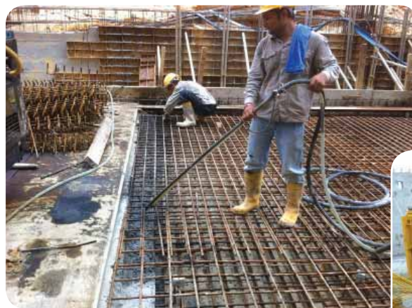
Clearing of debris from the concreting area
