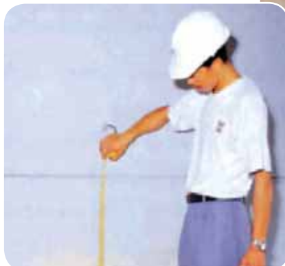
Checking the level of the substrate
