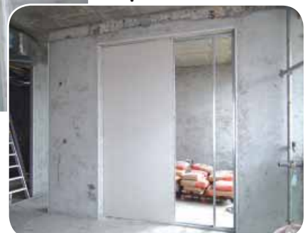
..... Installing plasterboard to one side of the framing
