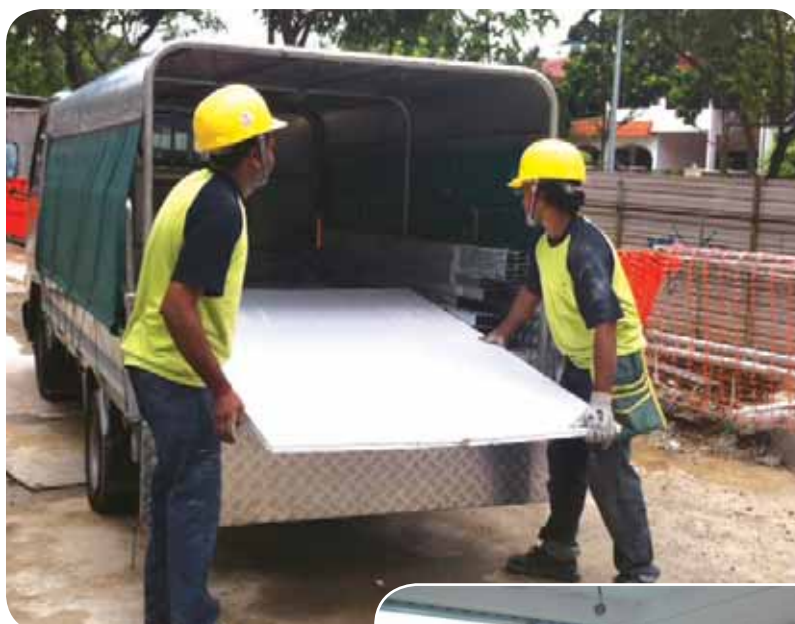
..... Transporting ceiling materials to working area
