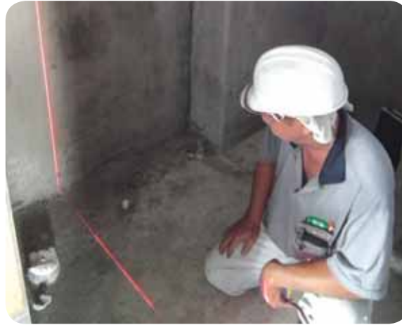
Setting out the position of the tiles and marking of reference line for tile laying
