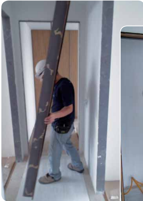
..... Installing of main frame
