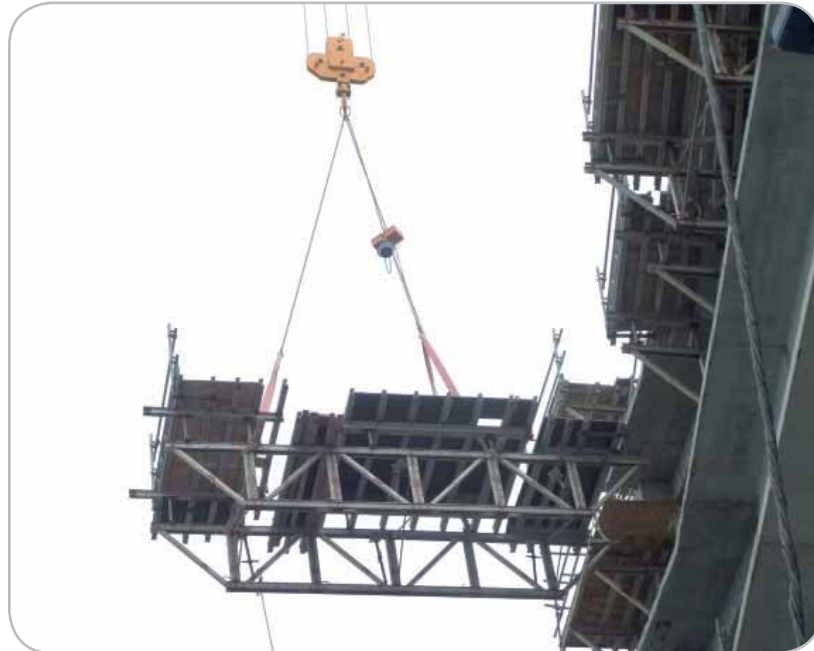
..... Lifting of table formwork by crane to the floor above.
