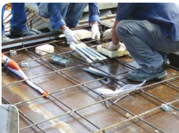
..... ..... Securing of conduits junction box
