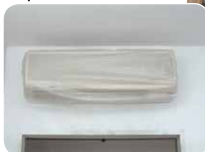
Protecting surfaces that are not intended to be painted.
