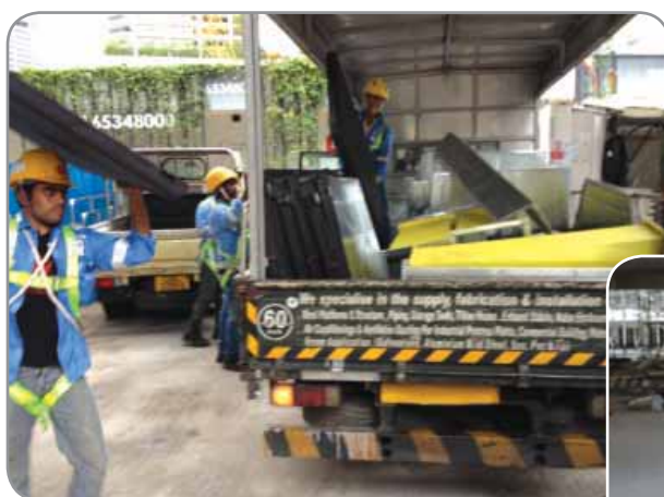
Transporting ducting materials to working area
