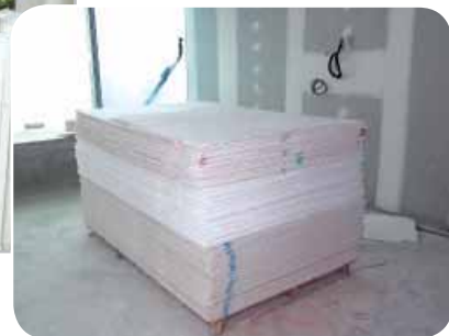
Placing of drywall materials near working area for easy accessibility
