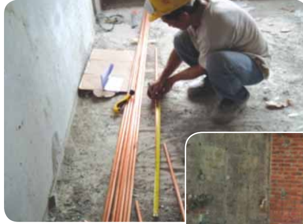
Measuring and marking on water pipe
