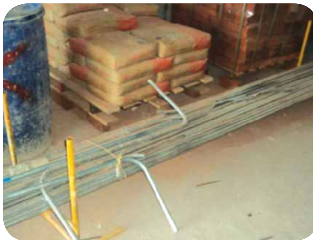
Placing of electrical conduits near working area
