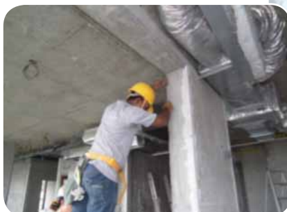
Transferring the floor marking to adjoining wall/column/ceiling
