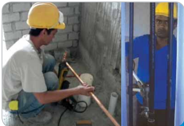
Jointing of water pipe by crimped connection
