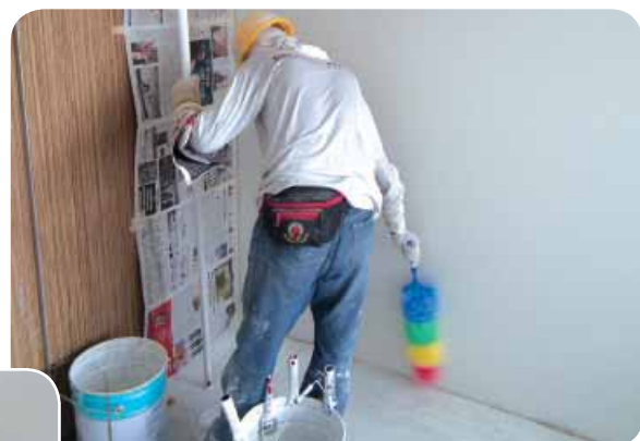
Cleaning to remove foreign and unstable matter
