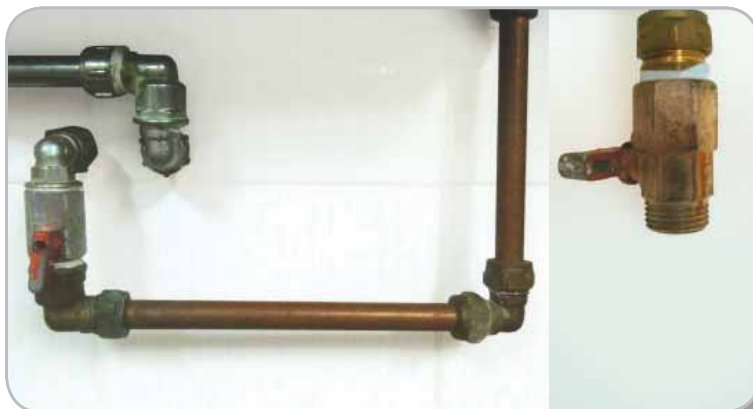
Joining of water pipe by threaded connection
