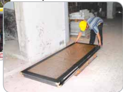
Placing of door frames and door panels near working area
