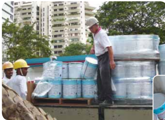
Transporting of painting materials to working area
