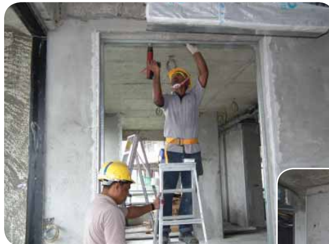
..... Installing the metal studs to form drywall frame
