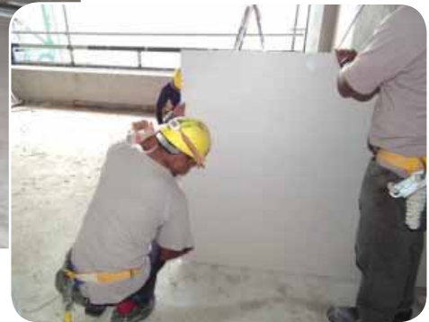
..... Marking out and cutting of the gypsum boards to actual size
