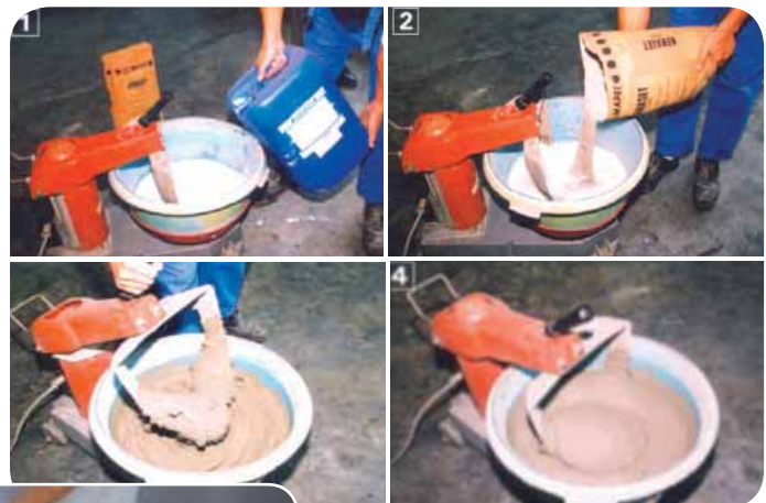
Mixing of cement mortar
