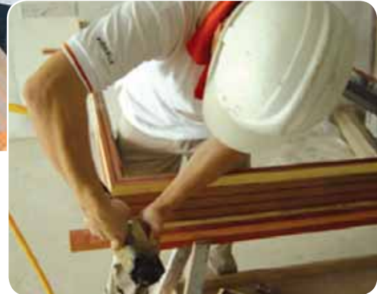
..... Treating surface of sub-frame
