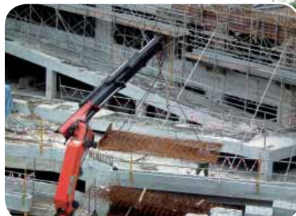
..... Transporting of prefabricated mesh to working area
