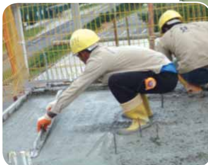
Manual levelling of concrete using trowel
