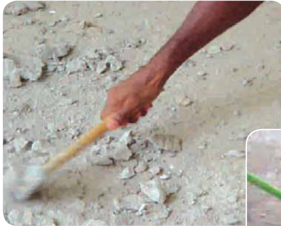
Removing concrete protrusion on the tiling area
