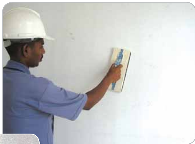
Intercoat preparation such as light sanding with fine-grade, preferably partly worn sandpaper can be used to remove nibs and adherent dust particles
