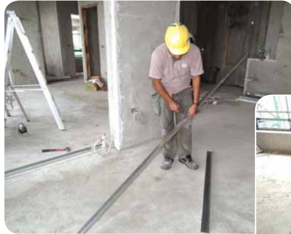
..... Cutting of metal studs to required size for drywall framing
