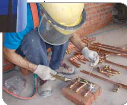
Jointing of water pipe by soldered connection
