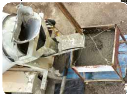
Crane and concrete bucket
