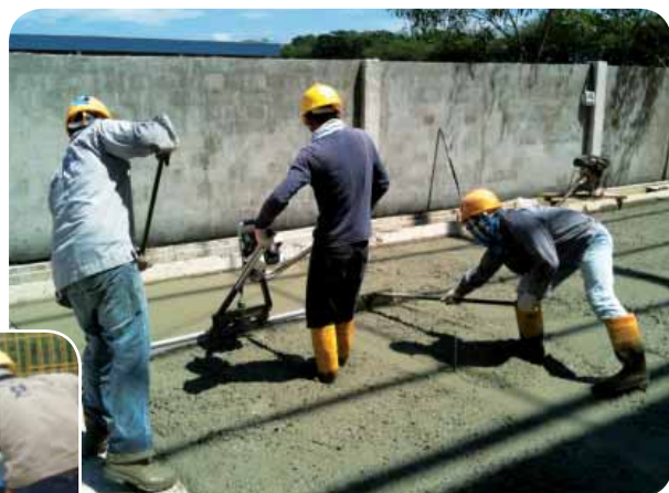
Mechanical levelling of concrete using vibrating screed leveller
