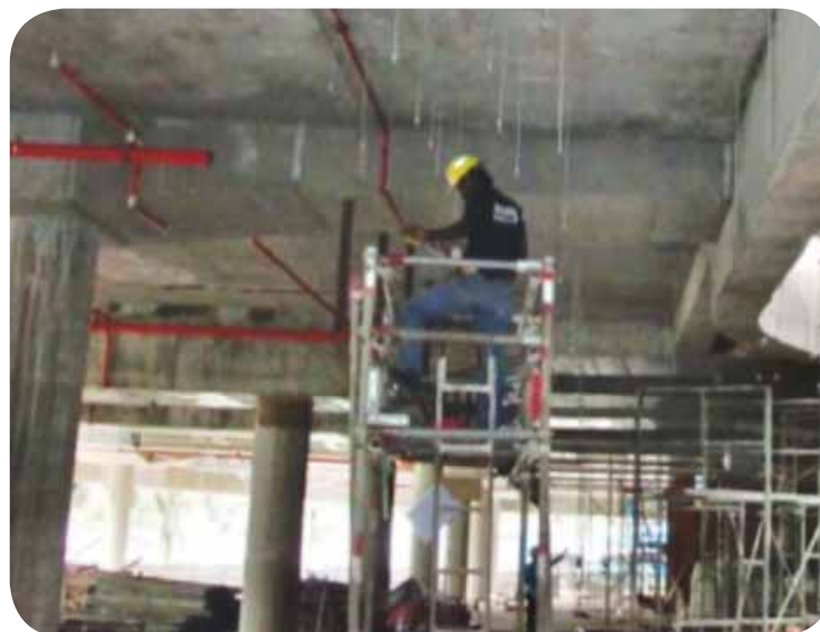
..... Setting the alignment and : fixing the hanger supports
