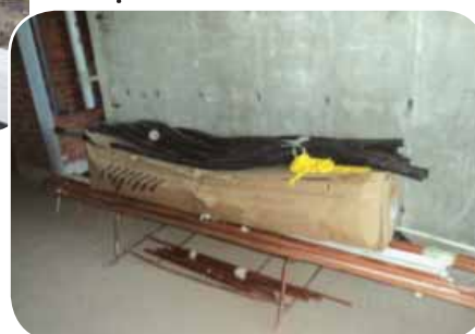
Placing of piping materials near working area
