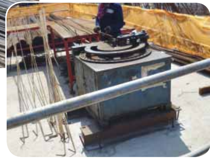
..... Bending of re-bars to required shape using bar bending machine
