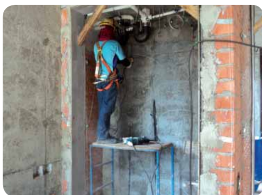
Hacking of grooves and opening (if necessary)
