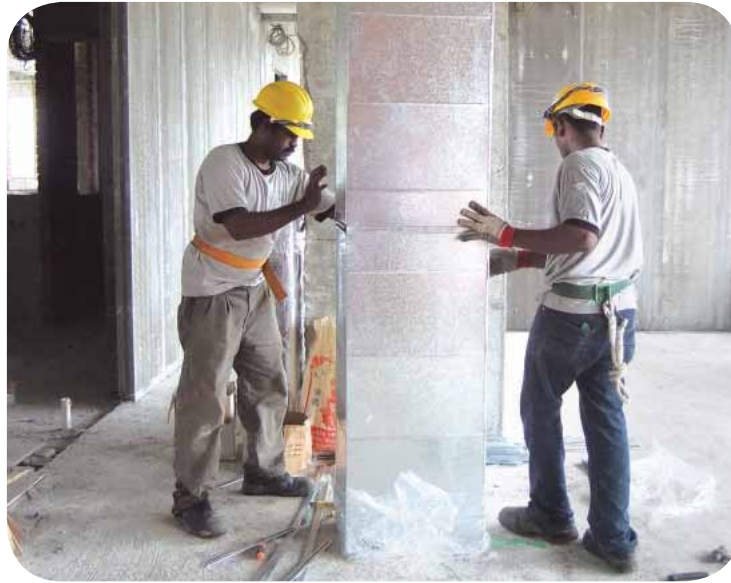
..... Assembling of duct : section
