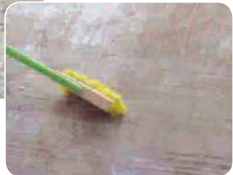
Cleaning concrete surface with broom
