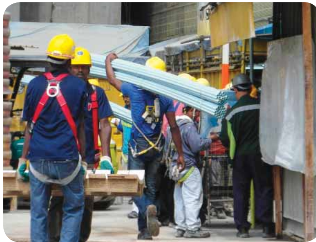
Transporting electrical conduits to working area
