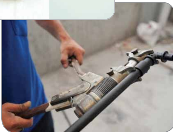
Joining of PEX pipe by pressed connection
