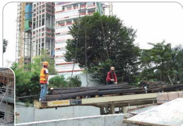
..... Transporting of re-bars to working area
