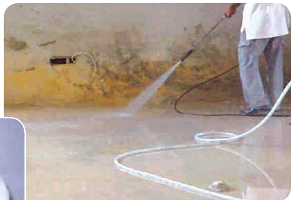
Cleaning concrete surface using water jet
