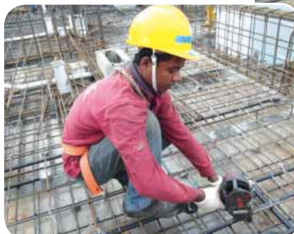
..... Fixing of re-bars using mechanical means
