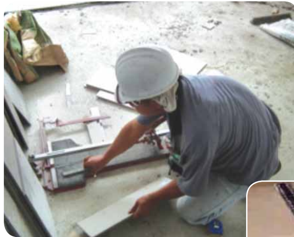
..... Cutting of tile to required size
