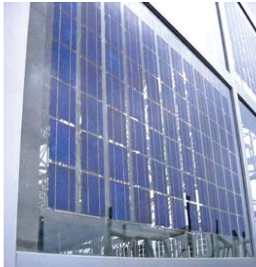
Figure 15. BIPV modules integrated into a façade
