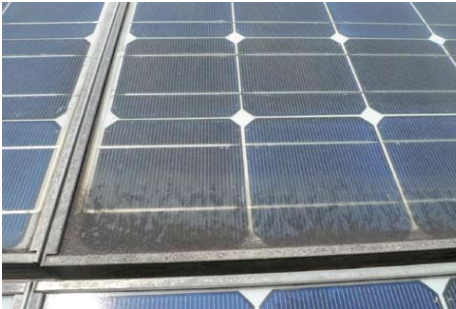
Figure 14. PV module frames trap dirt as water evaporates from a flat-mounted PV module
