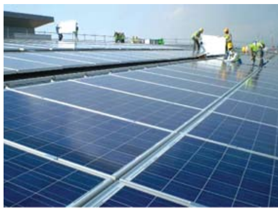
Figure A.6.3. Installing the REC modules
