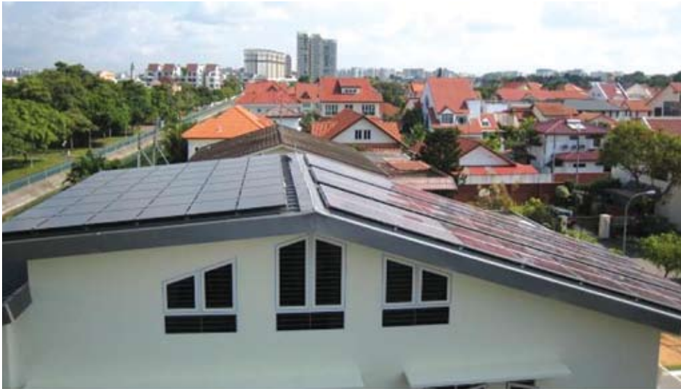
Figure A.7.1. Building roof with two types of PV module
