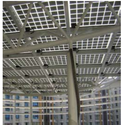
Figure 16. BIPV modules integrated into a skylight canopy
