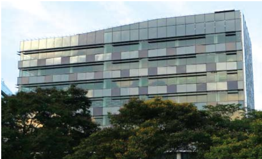
Figure A.8.1. 6kWp BIPV façade on Tower 2
