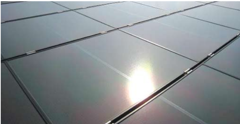
Figure A.7.2. West roof flank with micromorph PV modules
