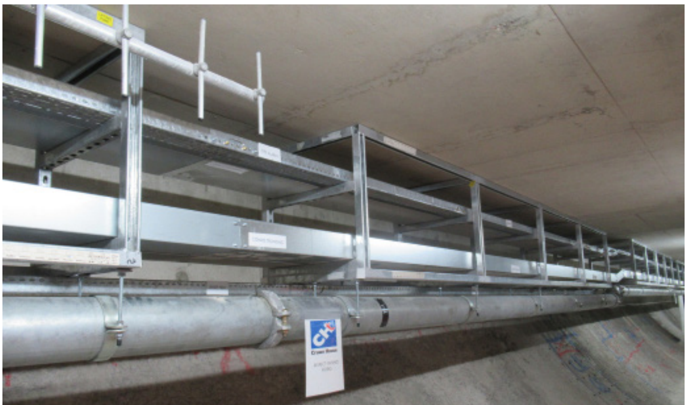
Figure 18 (Top): Prefabricated modules in the services tunnel. (Photograph courtesy of Laing O'Rourke)
