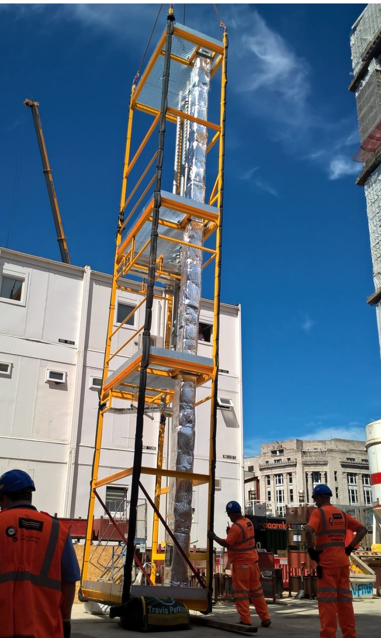
Figure 5: Lifting of vertical riser module (Photograph courtesy of Laing O'Rourke)
