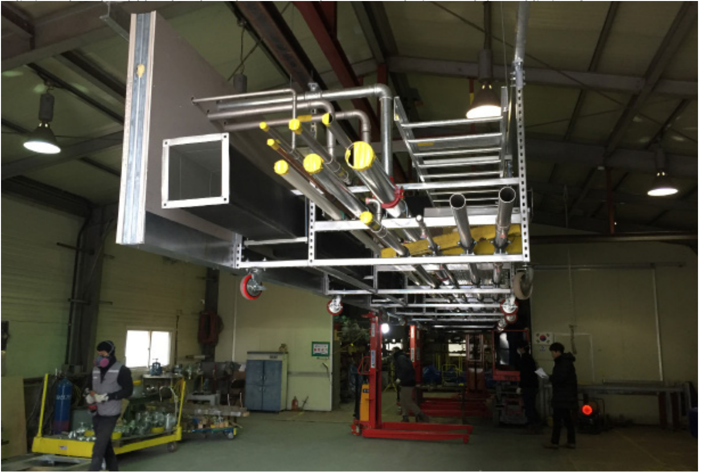
Figure 15: In Korea, prefabricated MEP modules are connected on the floor at the job site and lifted as a complete module for final installation. Synchronised wireless jacks are used to maintain alignment when lifting the module. (Photograph courtesy of Hyundai Engineering & Construction Pte Ltd)
