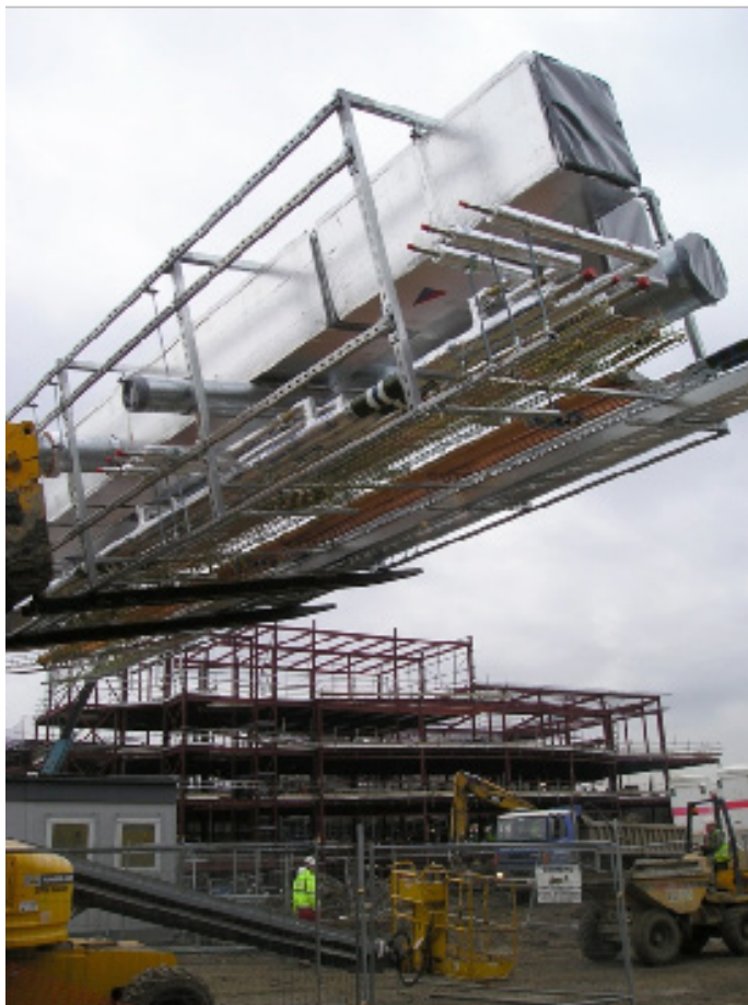
Figure 14: Lifting of modules on site. (Photograph courtesy by DSG Modular)
