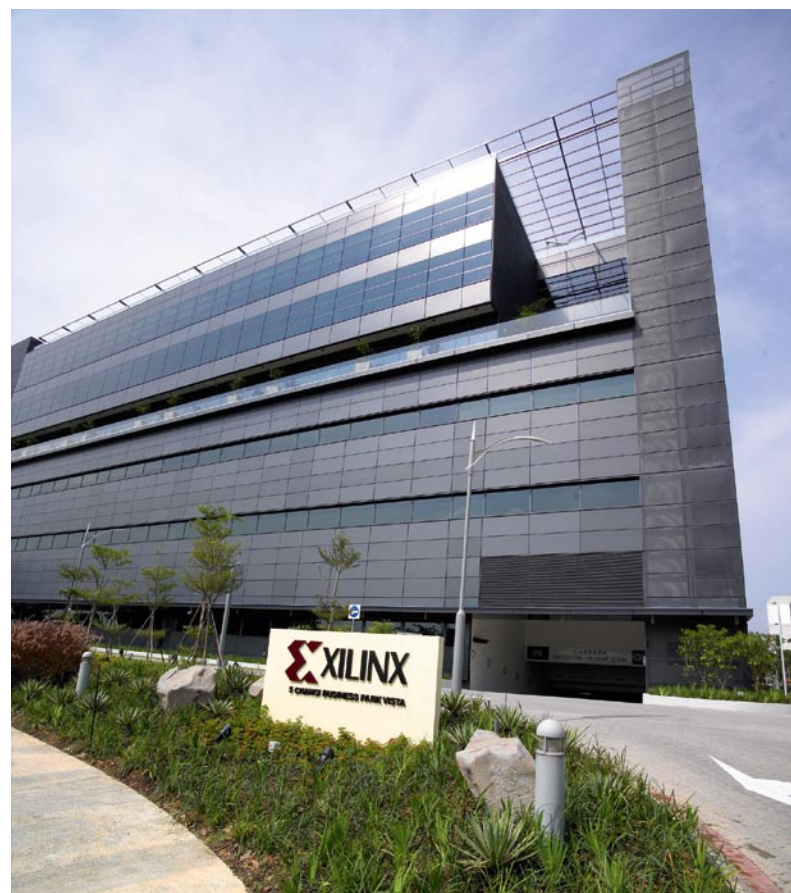
The dark grey façade comprises high performance double-glazed units with low-emissive coating in its curtain wall
