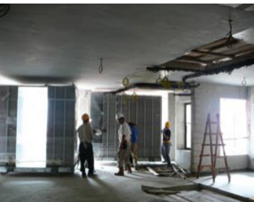
Loading of prefab bathroom units into each apartment
