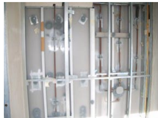
Coordinated services within drywall construction
