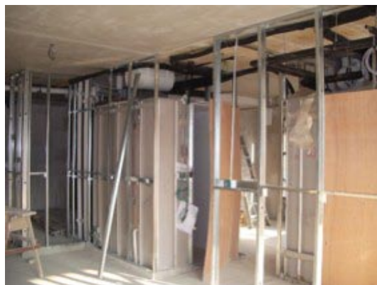
Installed prefab bathroom units
