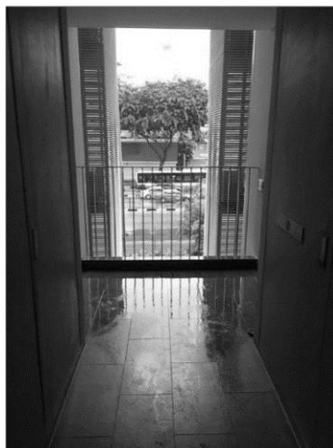
Figure 7: Railing as safety barriers resulting in extensive wind-driven rain into corridor
