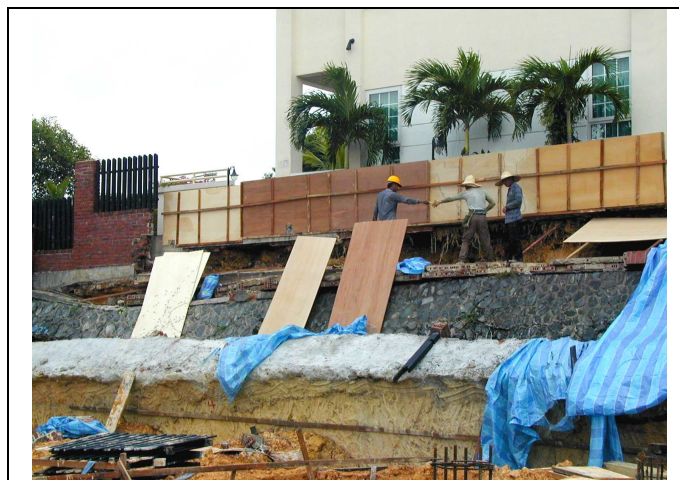
Figure 2: The failed rubble retaining wall
