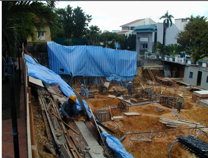
Figure 1: Excavation was carried out near the base of existing rubble wall
