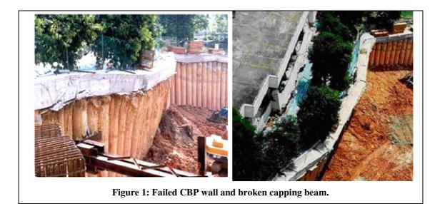
As there were buildings adjacent to the CBP wall, the excavated site had to be backfilled immediately. Non-stop round the clock backfilling operation was carried out over 7 days to restore the site back to its original level in order to stabilise the site condition.
