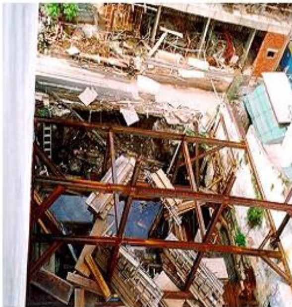
Figure 1: Excavation site with struts on 3 sides
